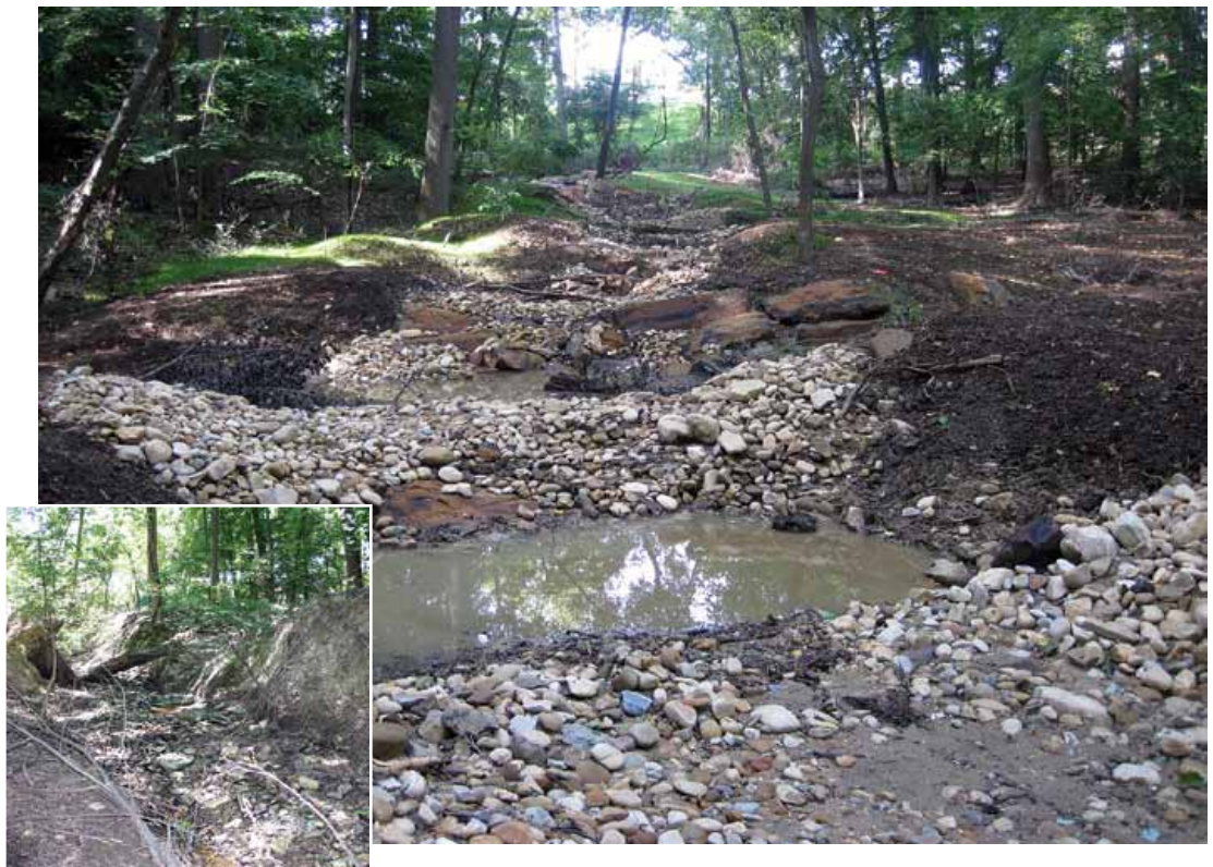
Completed stormwater conveyance on Millhouse Tributary in Rock Creek Park, DC, and stream condition before the project (inset)
