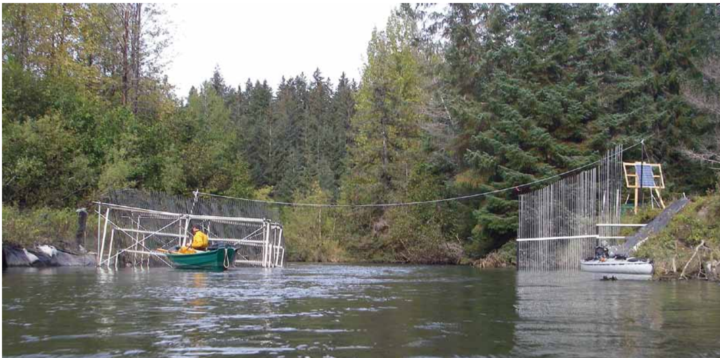
Fish fence installation on the Bartlett River in Glacier Bay National Park and Preserve NPS PHOTO
