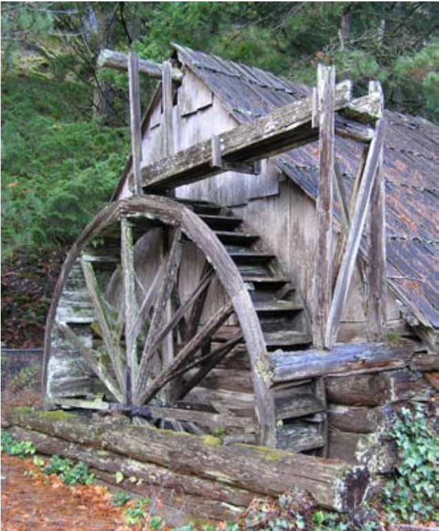
Historic water wheel building in Diablo.
