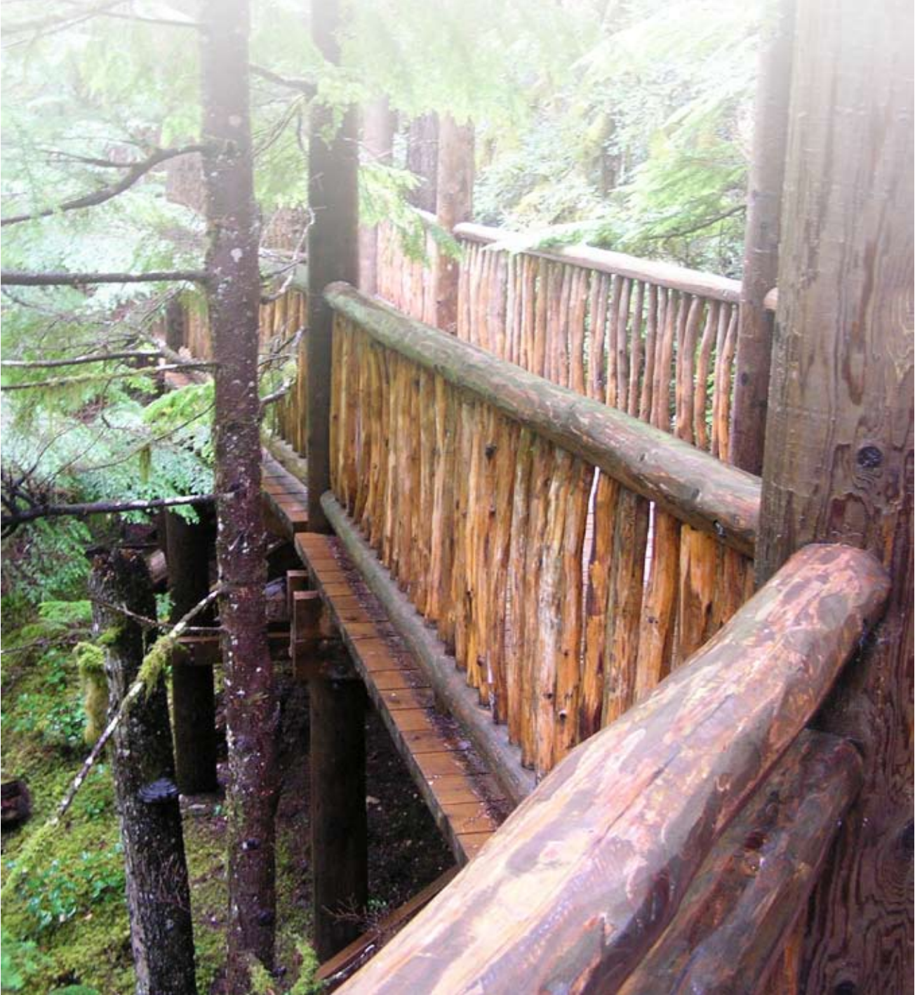
The accessible boardwalk of the Rock Shelter Trail near Newhalem.
