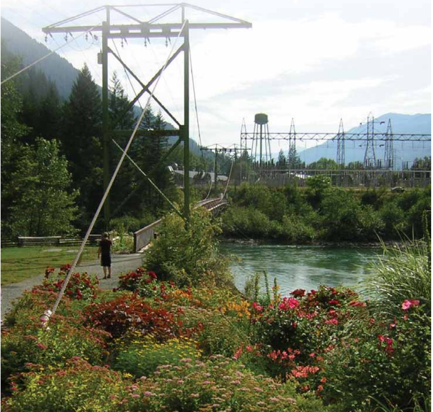
View from Gorge Dam hydropower facility toward Newhalem.
