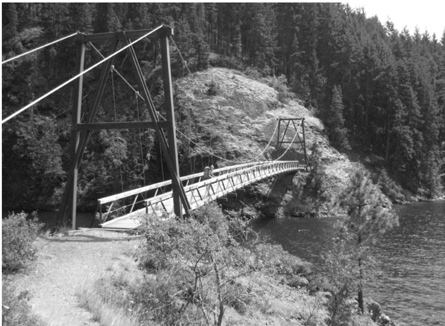
Bridge over Lightning Creek.
