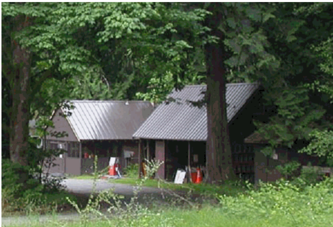
The garage (right) has had the front doors removed (PWRO-Seattle, 2004).
