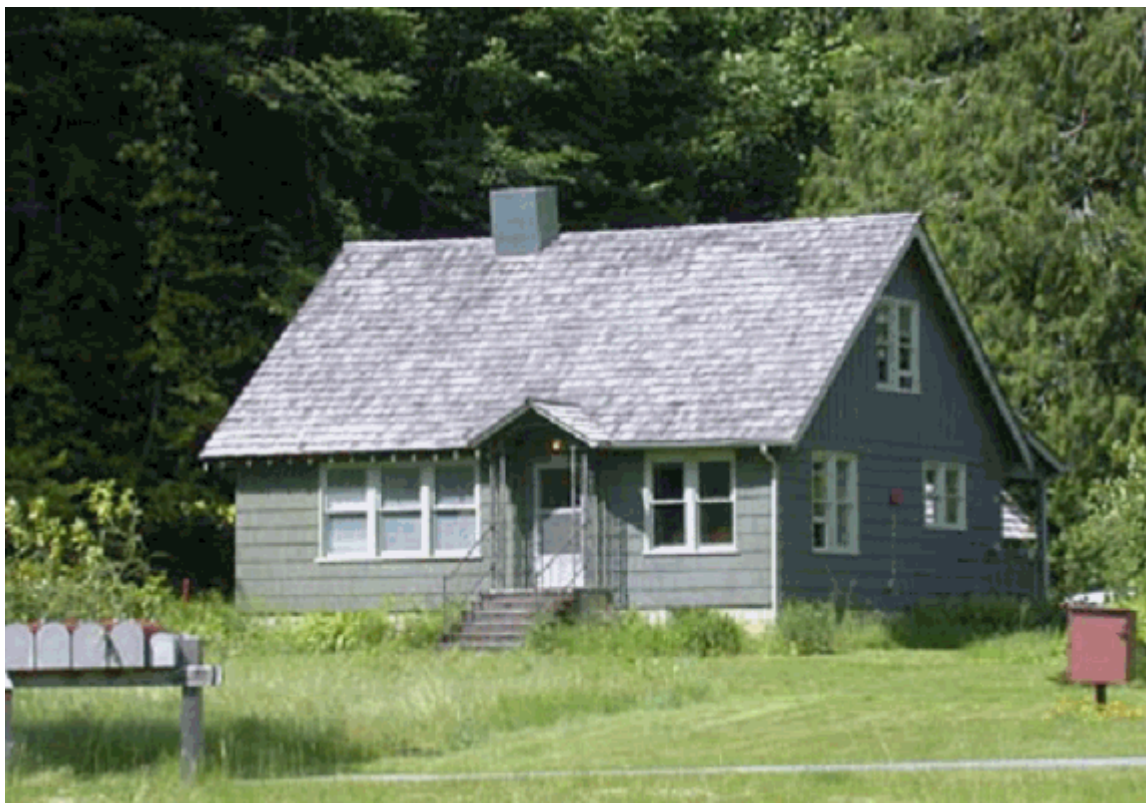
The District Ranger's Residence (building 1010), constructed in the 1930s by the CCC (PWRO-Seattle, 2004).
