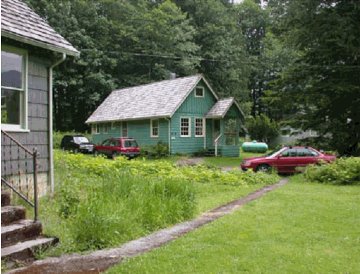
Historic concrete pathways to both residences still remain. This shows one of the walkways at the District Rangers Residence (PWRO-Seattle, 2004).
