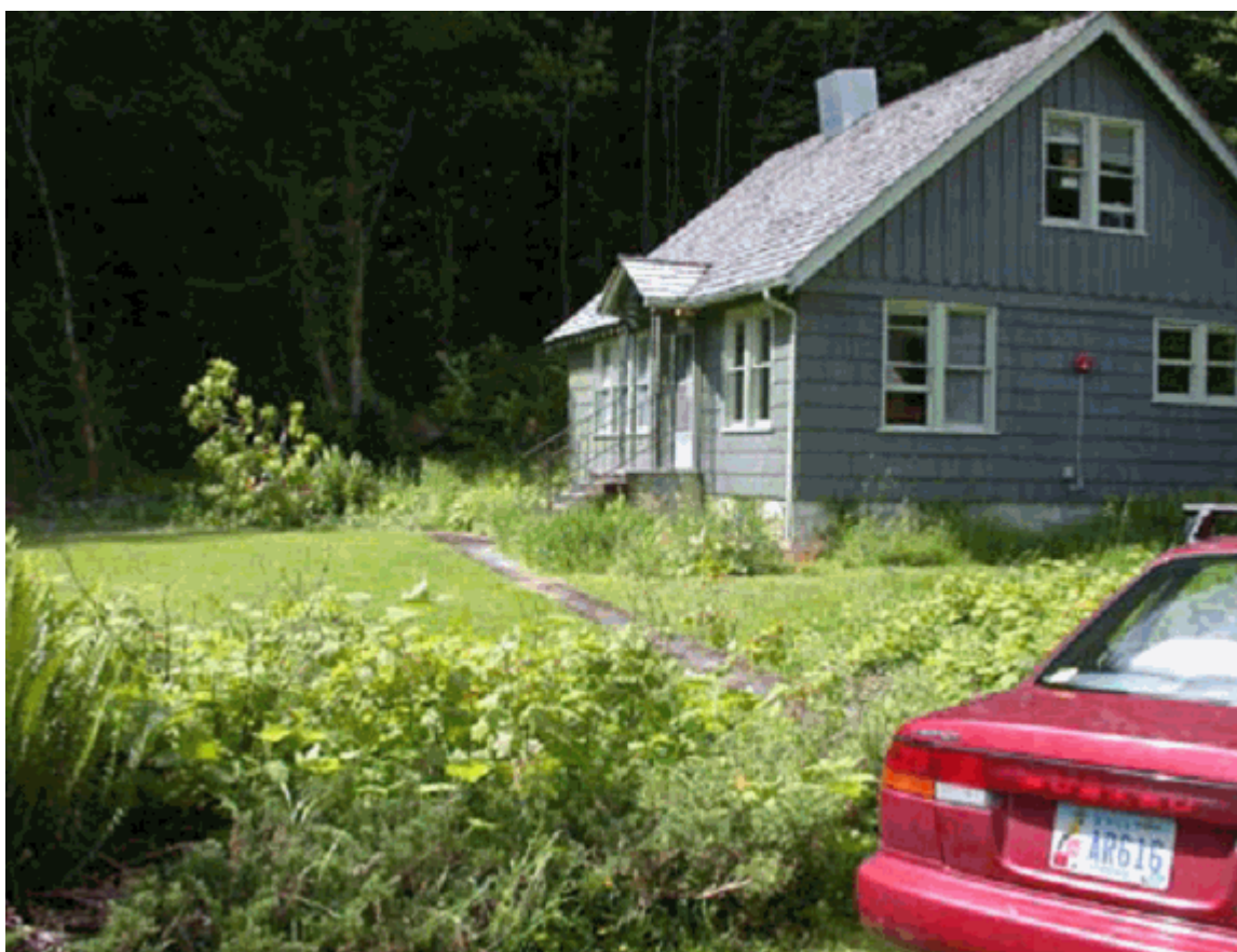
Ornamental shrubs and perennials grow in historic plant beds around the District Rangers Residence (PWRO-Seattle, 2004).
