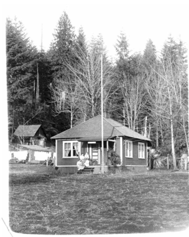
The first district ranger's house at Marblemount (Backus) Ranger Station, ca. 1916. Note the flagpole in front of the house and the barn and chicken coop in the rear (NOCA 11589, ca. 1916). This house was removed during the period of significance.
