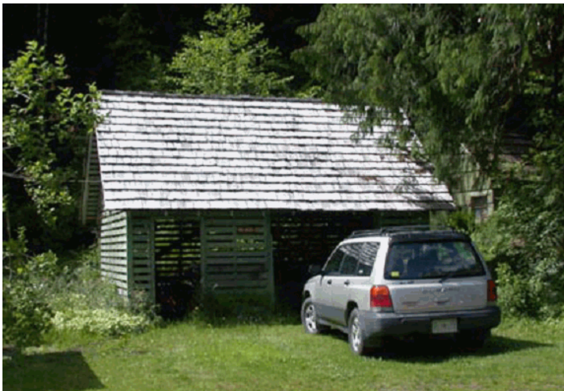
The Woodshed located behind the District Ranger's Residence (PWRO-Seattle, 2004).
