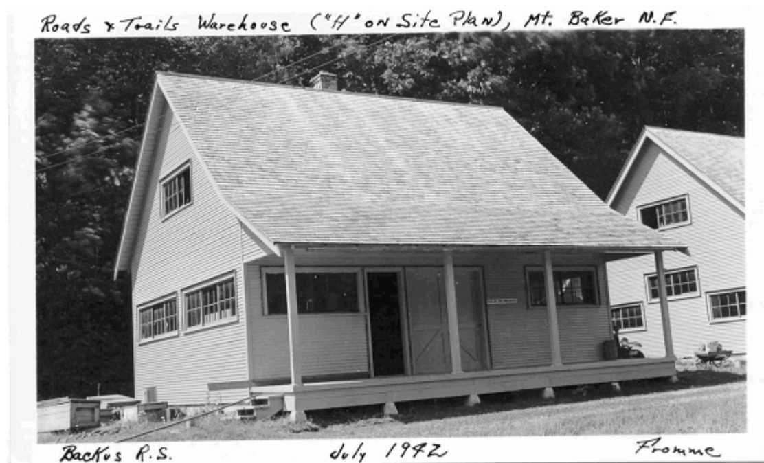
Historic photograph of the R&T storage building at Marblemount (Backus) Ranger Station, built by the CCC during the 1930s (NOCA 11294, 1942).
