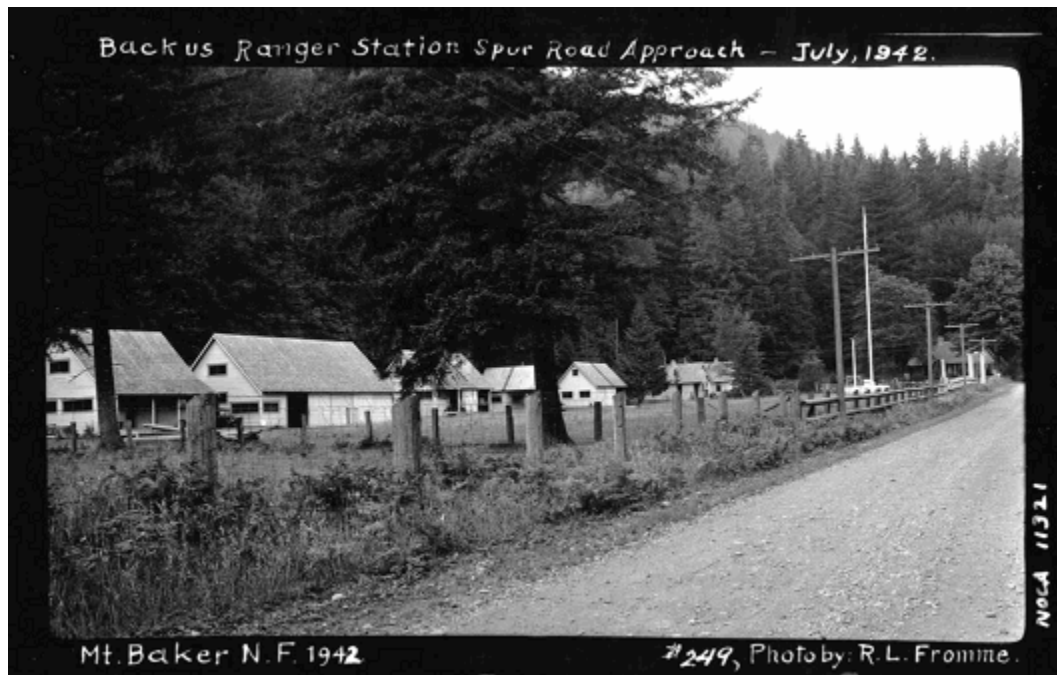
Historic photograph of Marblemount (Backus) Ranger Station, viewed looking north and west from Ranger Station Road. Note the row of utilitarian buildings built by the CCC and the fenced pasture (NOCA 11321, 1942).
