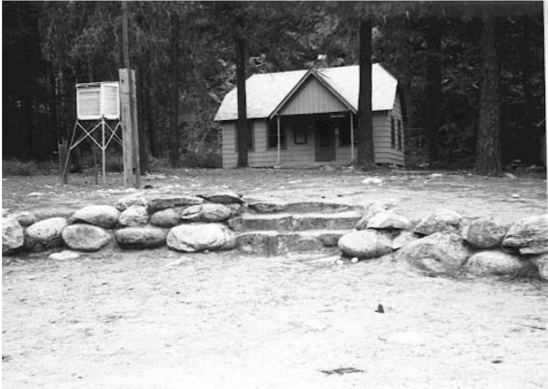
Photograph c. 1984 showing residence in the background and the weather station on the left. As there were no designated trails aligned to the weather station, vegetation was trampled by foot traffic (NOCA Collection).
