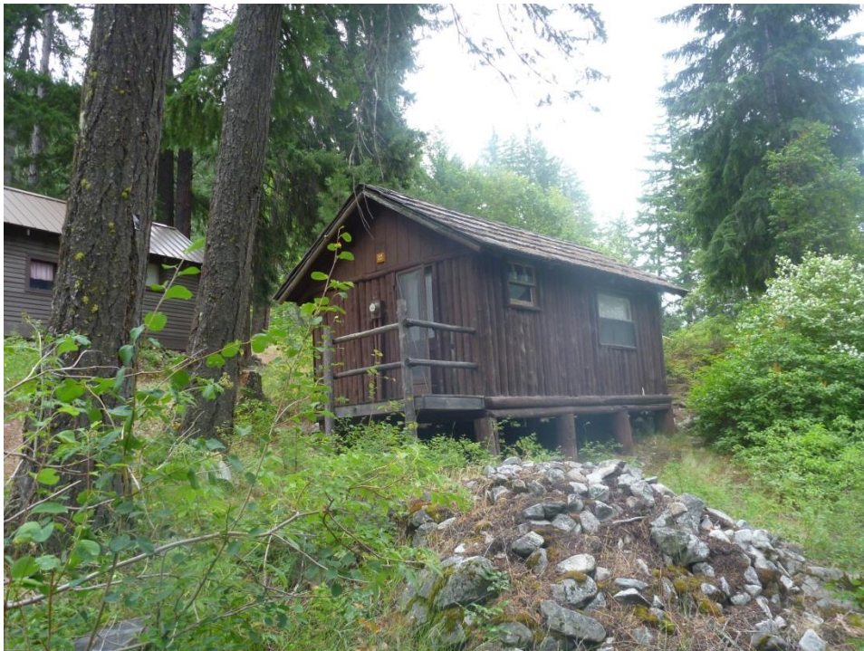
Buildings and Structures #5: Cabin #12, looking east. (PWRO, June 2013)
