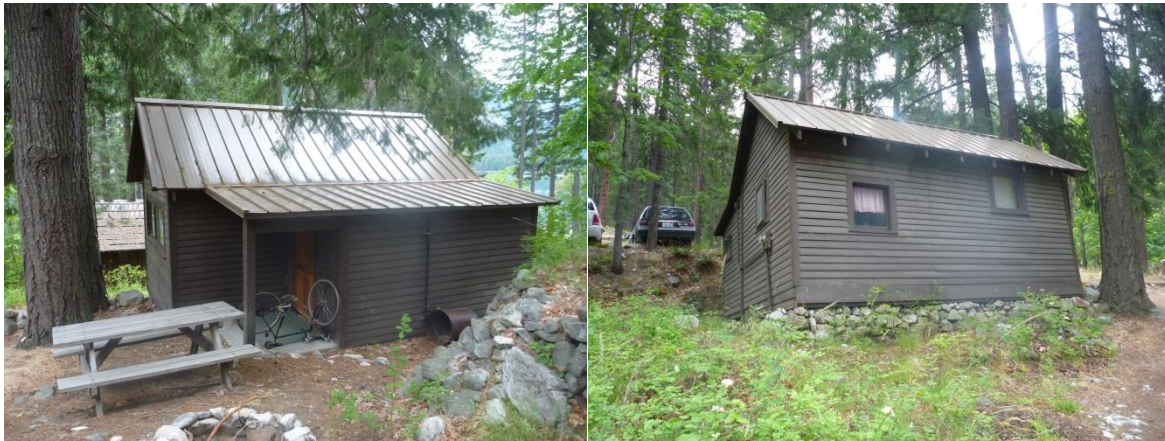
Buildings and Structures #3: Cabin #10, looking west (left) and east (right). (PWRO, June 2013)
