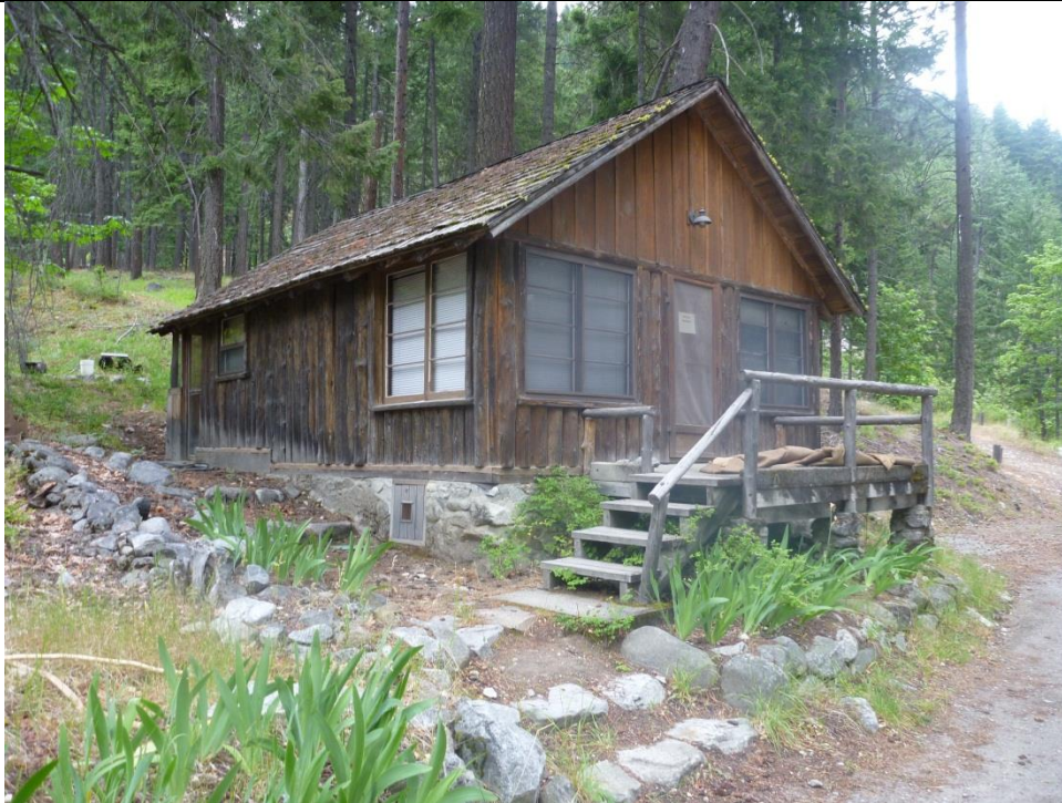
Buildings and Structures #4: Cabin #11, looking northeast. (PWRO, June 2013)
