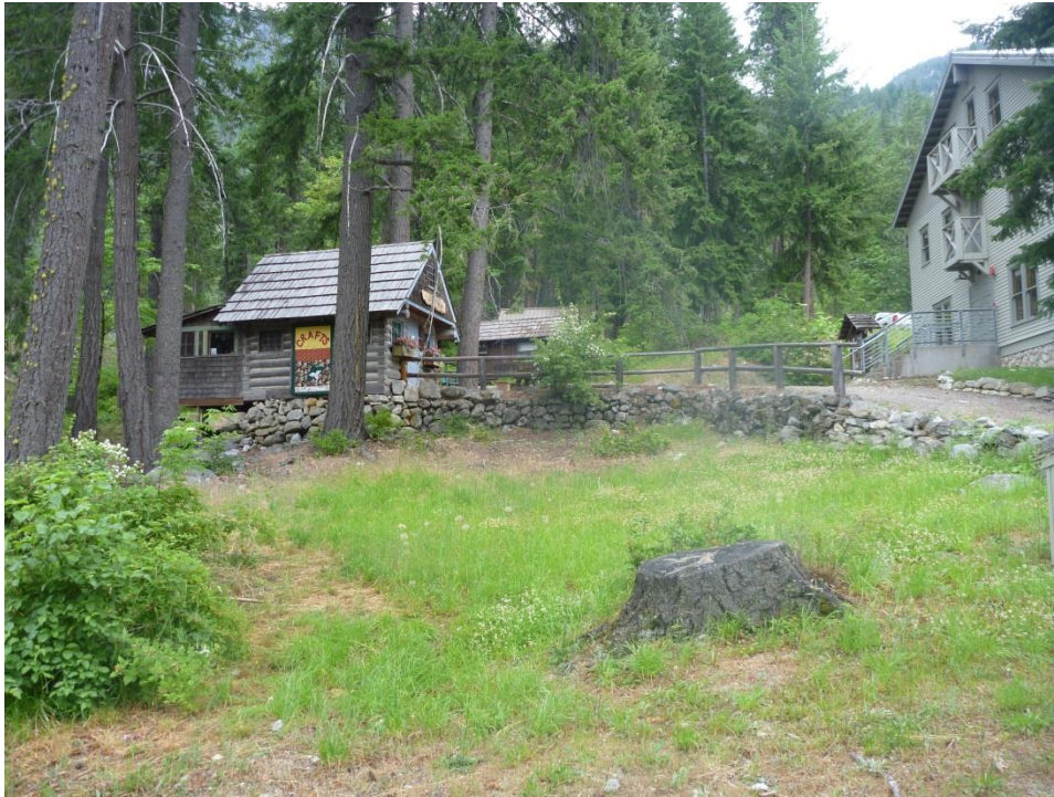
Topography #8: Rock wall on downhill side of the road around the lodge and Cabin #14 (The House that Jack Built), looking northeast. (PWR, June 2013)
