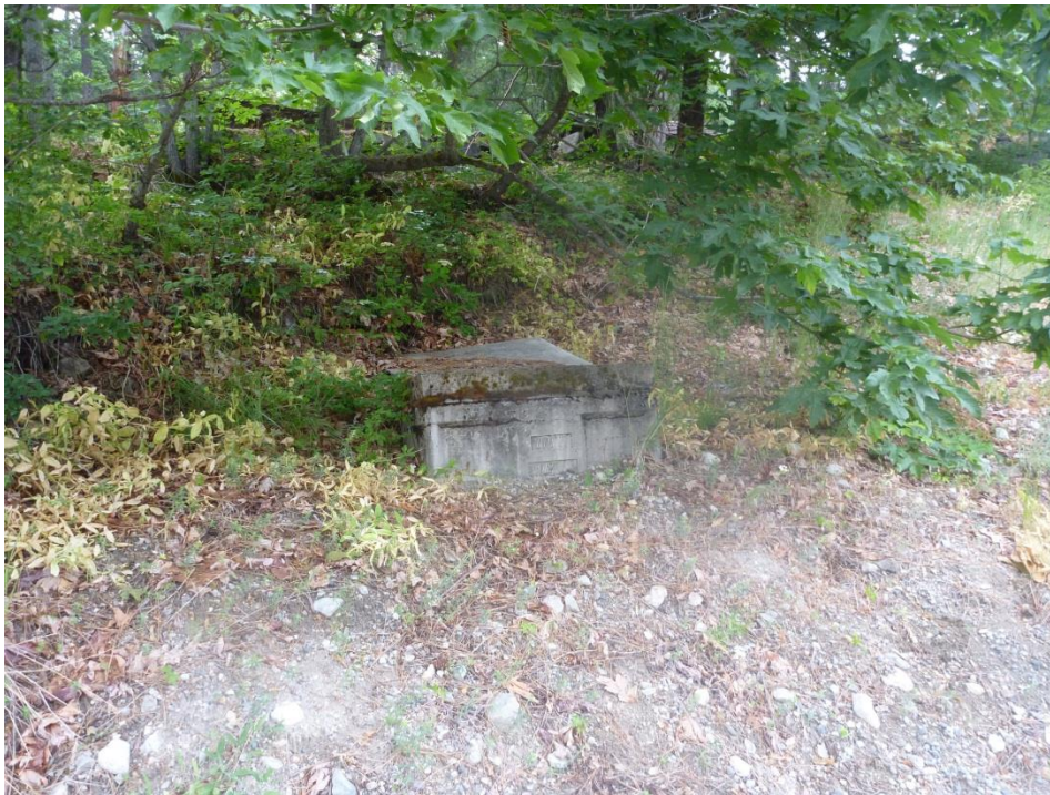
Buildings and Structures #10: Concrete Vault, looking northeast. (PWRO, June 2013)
