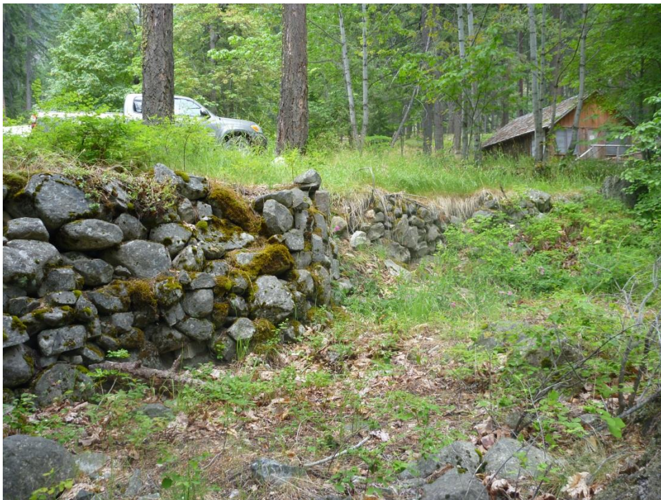
Topography #9: Rockwall supporting road segment near Cabin #11, looking east. (PWR, June 2013)
