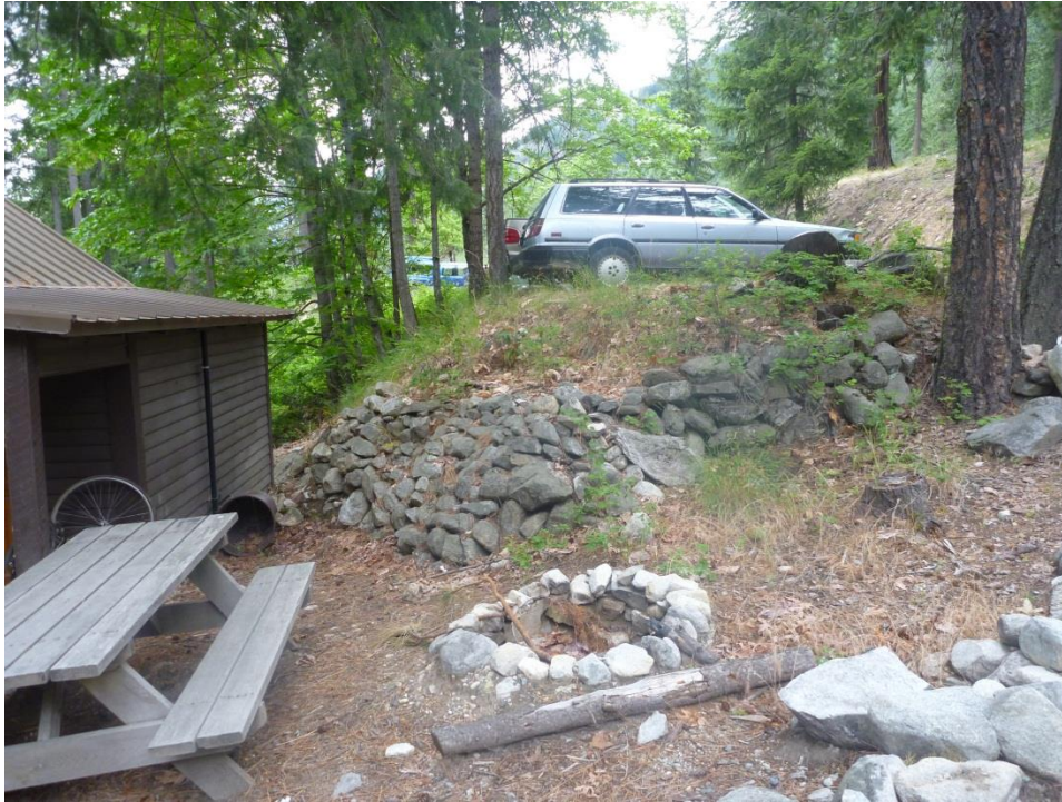
Topography #10: Retaining wall behind Cabin #10, looking northwest. (PWR, June 2013)
