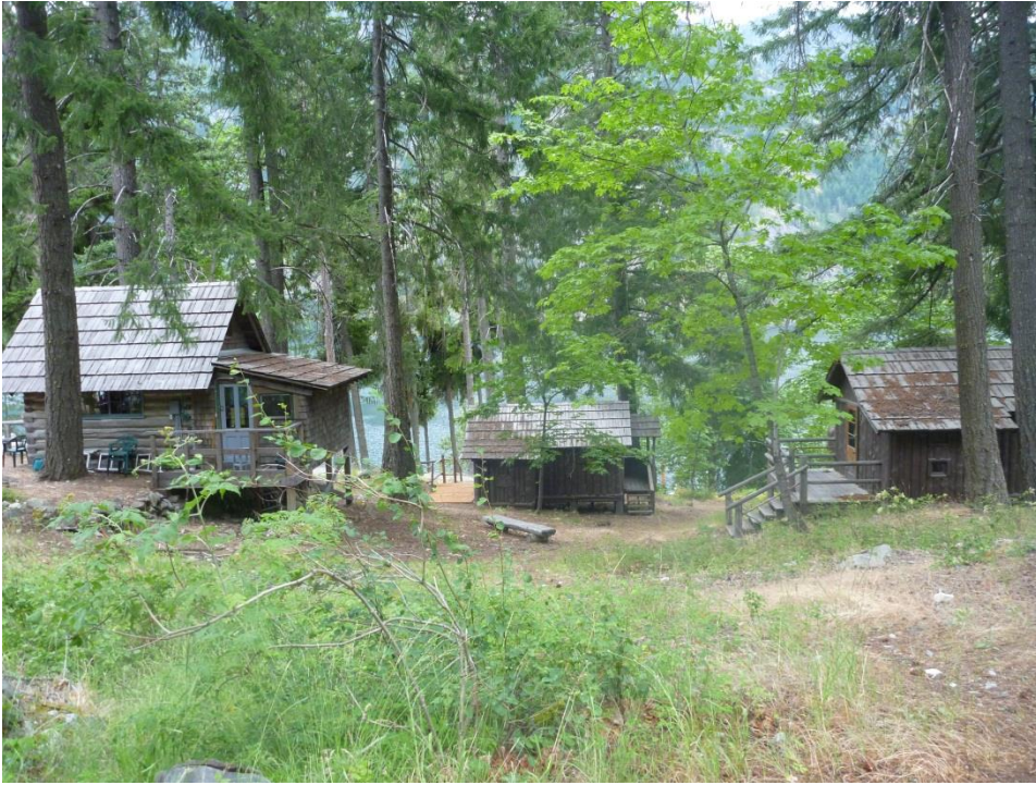
Spatial Organization #3: Cluster of cabins north of the Golden West Lodge: Cabins #14, #15, and #13 (from left to right), looking southwest. (PWR, June 2013)
