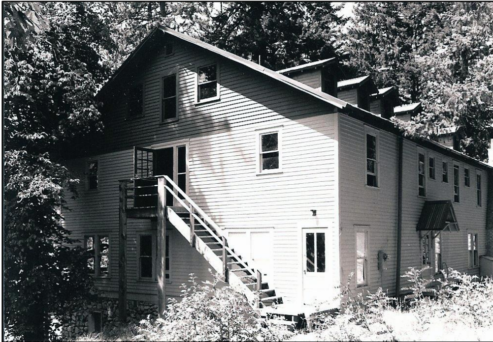
History #13: Photograph of the side and rear of the Golden West Lodge, circa 1980s. This photograph was taken prior to rehabilitation work, which modified both elevations (NOCA 17304-30).
