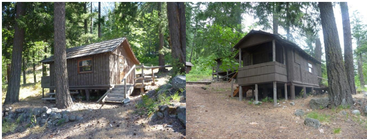
Buildings and Structures #8: Cabin #15, looking north (left) and east (right). (PWRO, June 2013)
