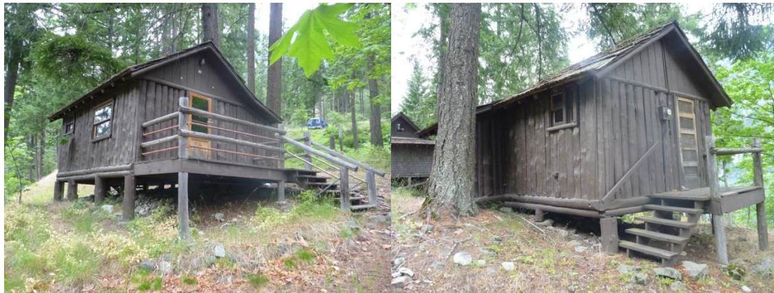
Buildings and Structures #6: Cabin #13, looking north (left) and east (right). (PWRO, June 2013)
