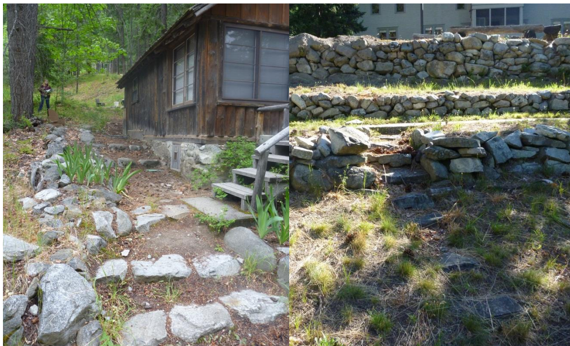
Circulation #4: Stone steps and paths at Cabin #11 (left) and the shuffleboard court (right). (PWR, June 2013)
