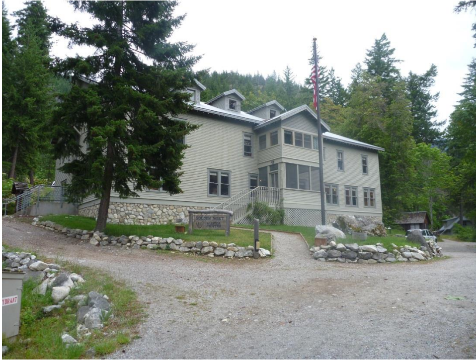
Circulation #2: Road around the Lodge and the reestablished entrance path to the lodge, looking east. (PWR, June 2013)
