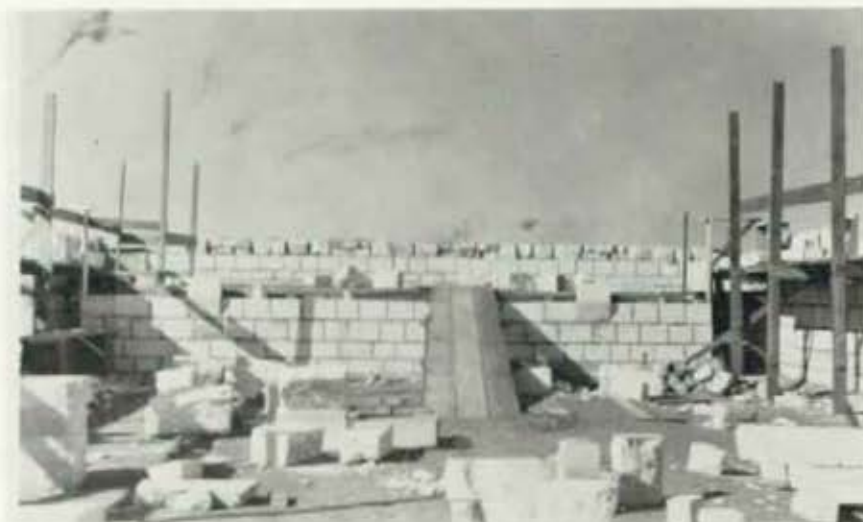
FIGURE III-6 & 7: Dedicated in 1939, Nicodemus Township Hall is shown under construction in these historic photographs. A team of 12 black and white local residents undertook this WPA project using locally quarried stone. It is the largest structure in town today. (Photographs: Angela Bates)
