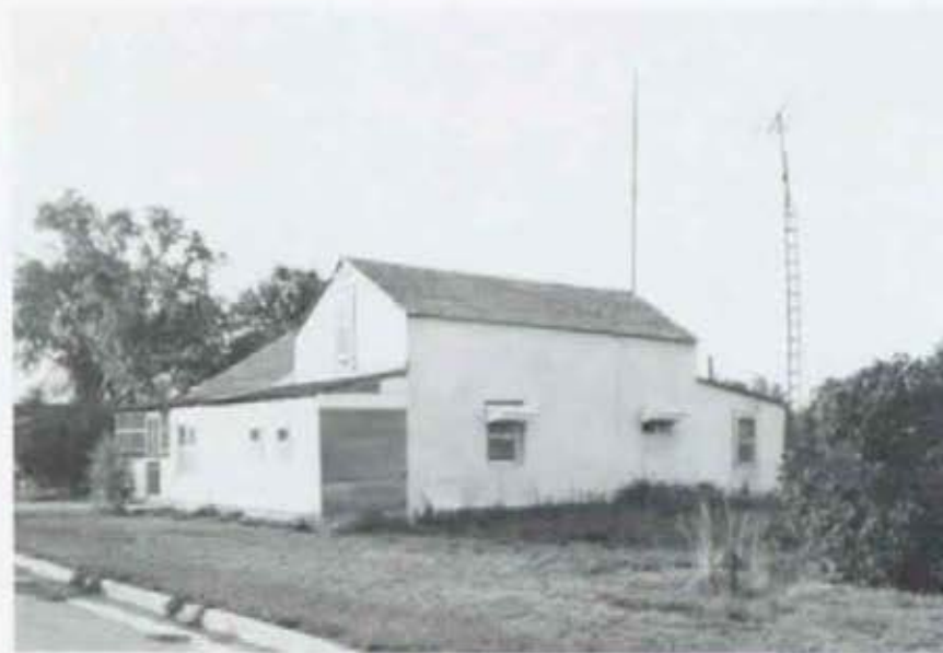
FIGURE II-9: The Saint Francis Hotel (now referred to as the Fletcher-Switzer residence). Zach Fletcher's 1881 hotel is the two-story stuccoed portion to the right, and originally featured a cut limestone appearance with a one-story stone kitchen addition on the east. This historic structure has received numerous alterations and additions over the years, but remains as one of the oldest extant historic buildings in Nicodemus today. (Photograph: Clayton Fraser)
