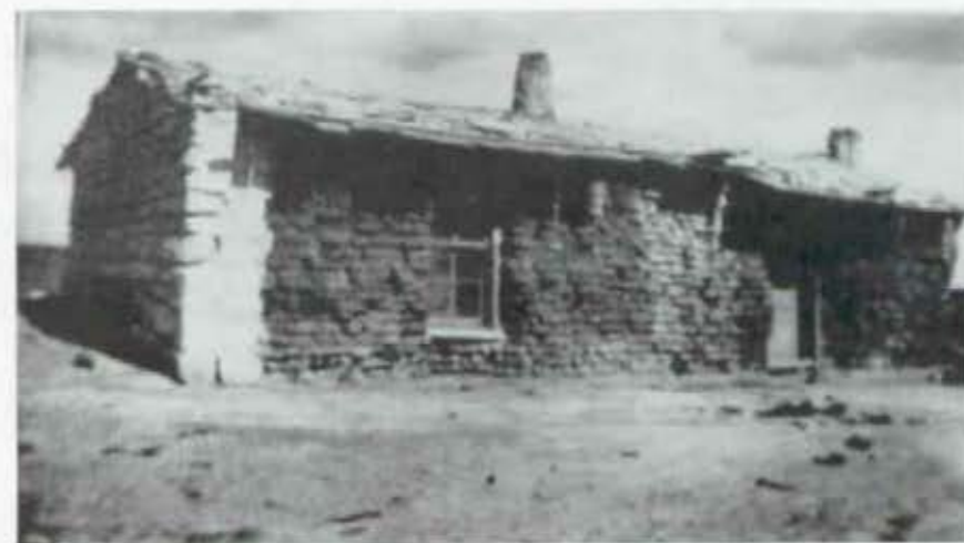
FIGURE 1-7: This rare historic photograph of an above-ground Nicodemus sod house, or "soddy," was identified as the Tuss-Lacey house by present-day local residents. Note that one elevation is of limestone construction, a popular but more expensive and time-consuming building method than was usually employed. The structure is no longer extant. (Photograph: Ernestine VanDuvall)
