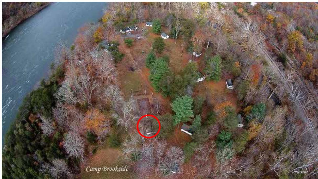
Figure 18. Aerial photograph of Camp Brookside showing pool's chemical treatment building (circled) and other historic structures with New River's Brooks Falls to the left (George Bragg, photographer).
