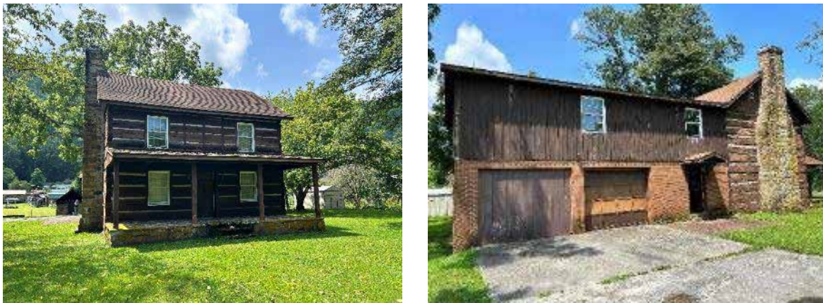
Figure 14. The historic Vallandingham House (left) is a late-19th century log cabin farmhouse with a non-historic rear addition (right) which detracts from its historic character.
