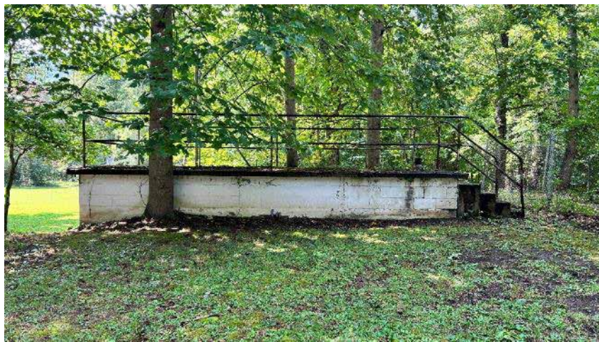
Figure 20. The Camp Brookside Pool Chemical Treatment Building, partially obscured from view from the main camp areas by topography and vegetation.
