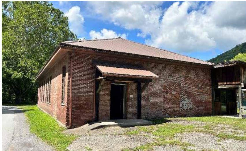
Figure 17. The Dun Glen Building/Ranger Station is a remnant of the former Dun Glen Hotel, which was documented as a pivotal structure to the Thurmond Historic District.
