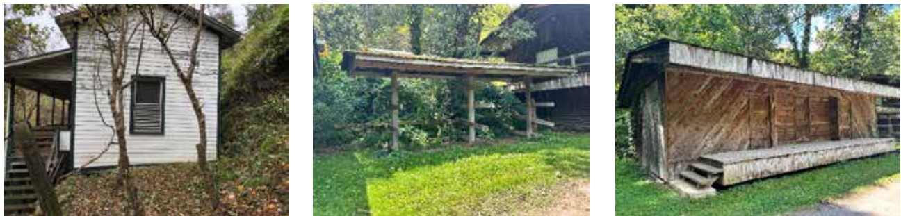
Figure 11. The Tom Kelly House (left), the Dun Glen Boat Storage Rack (center), and the Dun Glen Mini Ark (right) would potentially be retained if viable lease proposals are received by the NPS.
