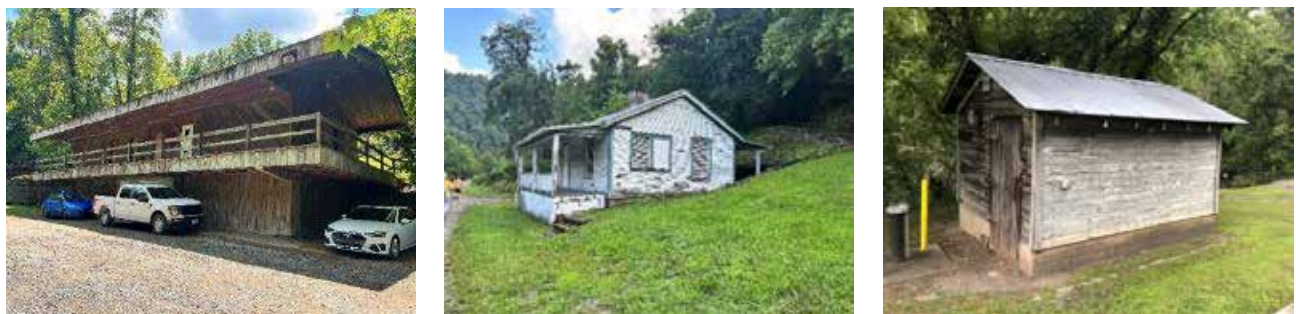
Figure 10. The Dun Glen Ark (left), the Marilyn Brown House (center), and the Thurmond Ice House (right) would be retained under alternative C.
