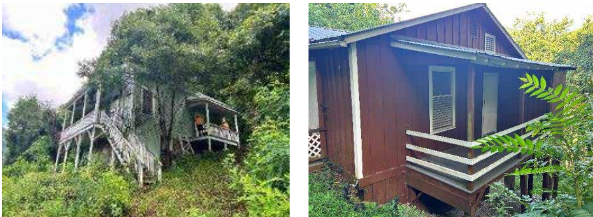
Figure 16. The Sidney Allen Ward House (left) and the Harold Smith House (right) are examples of houses for railroad managers and railroad workers, respectively; both are proposed to be excess.
