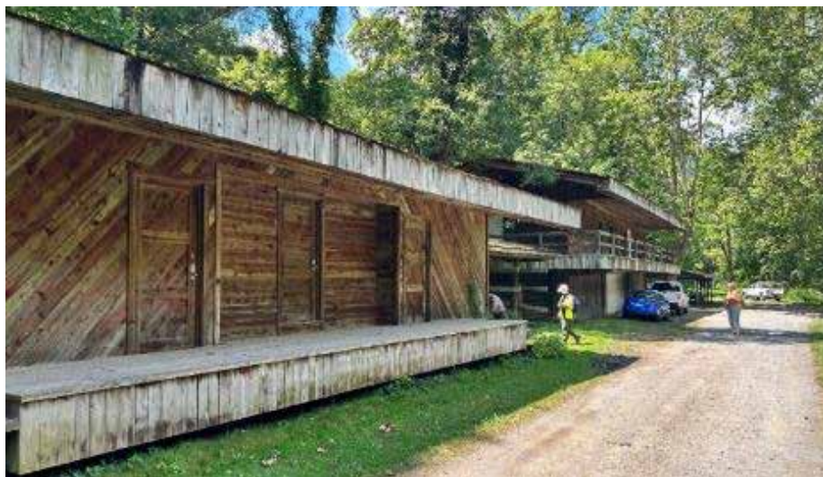
Figure 13. The Dun Glen Mini Ark (foreground), Boat Storage Rack (center), and Ark (background right) are associated with the statewide whitewater rafting industry.
