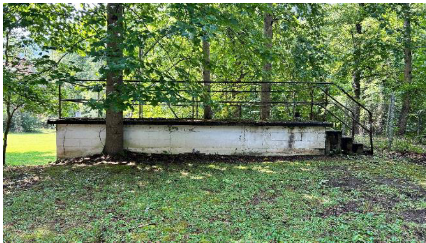
Figure 19. The Camp Brookside Pool Chemical Treatment Building, partially obscured from view from the main camp areas by topography and vegetation.
