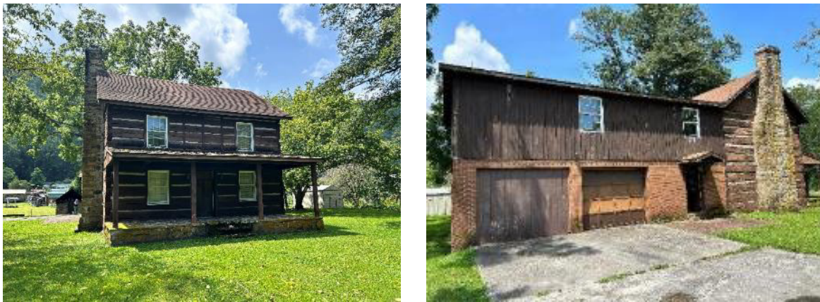
Figure 13. The historic Vallandingham House (left) is a late-19th century log cabin farmhouse with a non-historic rear addition (right) which detracts from its historic character.
