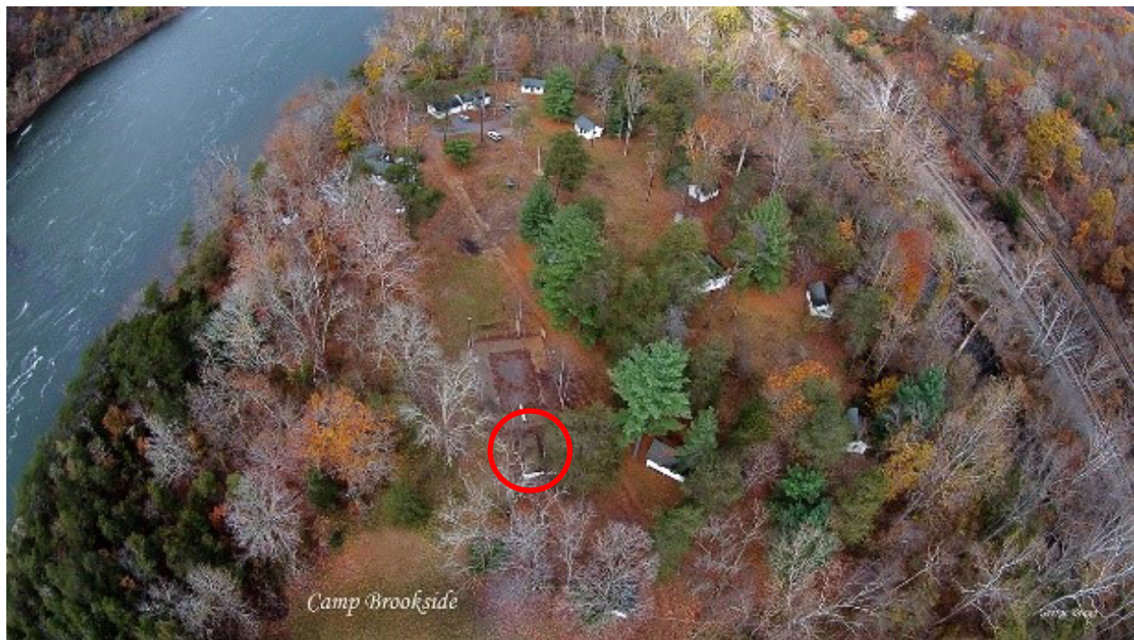
Figure 17. Aerial photograph of Camp Brookside showing pool's chemical treatment building (circled) and other historic structures with New River's Brooks Falls to the left (George Bragg, photographer).
