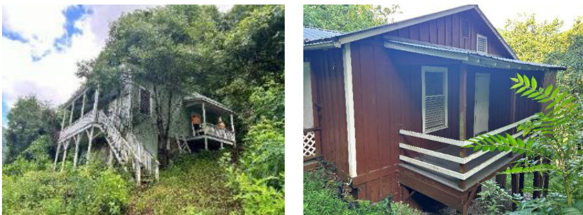
Figure 15. The Sidney Allen Ward House (left) and the Harold Smith House (right) are examples of houses for railroad managers and railroad workers, respectively; both are proposed to be excess.
