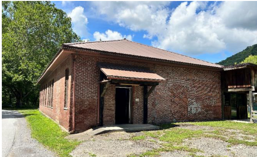
Figure 16. The Dun Glen Building/Ranger Station is a remnant of the former Dun Glen Hotel, which was documented as a pivotal structure to the Thurmond Historic District.
