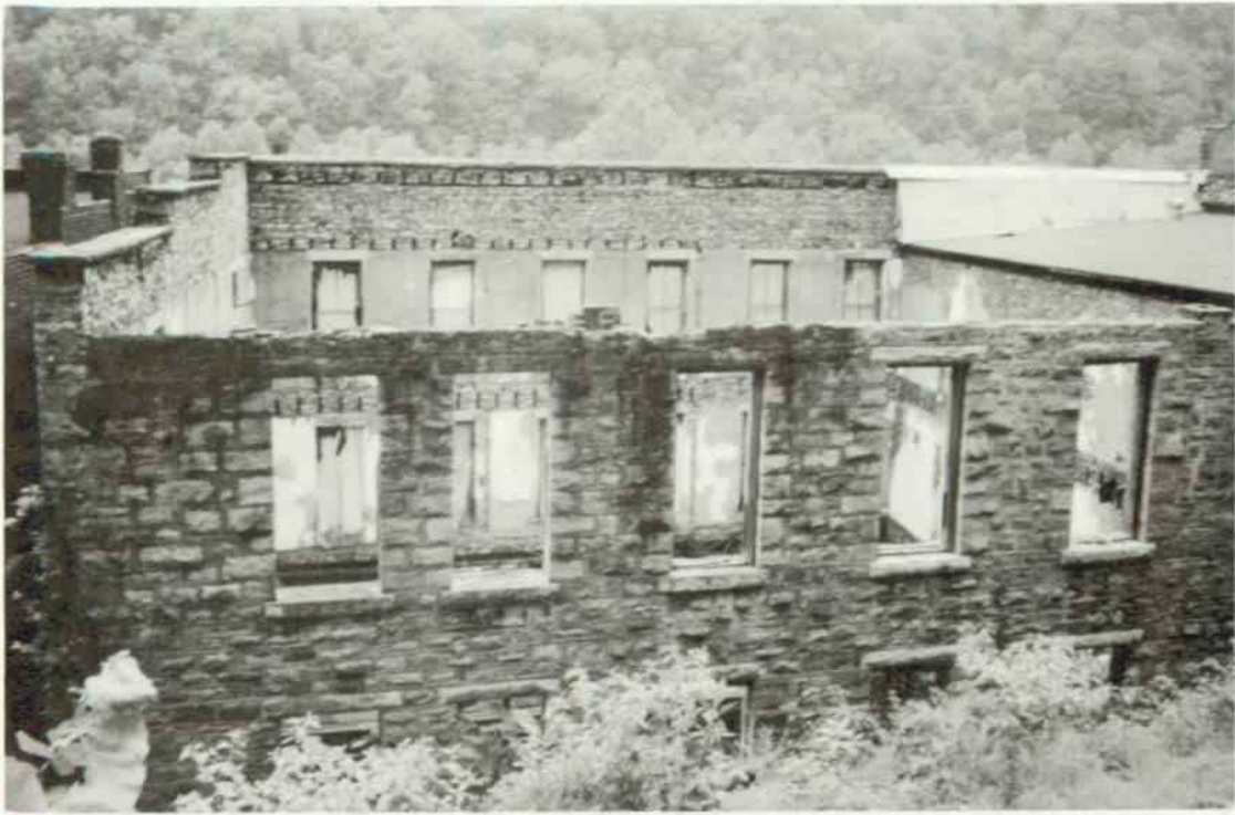
PHOTOGRAPH NO. 10: Goodwin-Kincaid Building - back view
