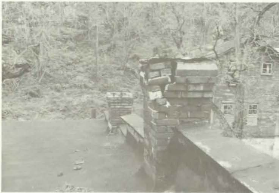
Figure 19 Southwest Chimney, Mankin-Cox Building, April 1991 (NPS Photo)
