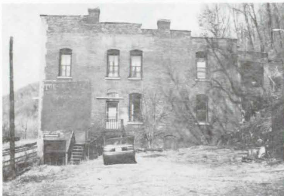
Figure 13 South Elevation, Mankin-Cox Building, March 1990 (NPS Photo)
