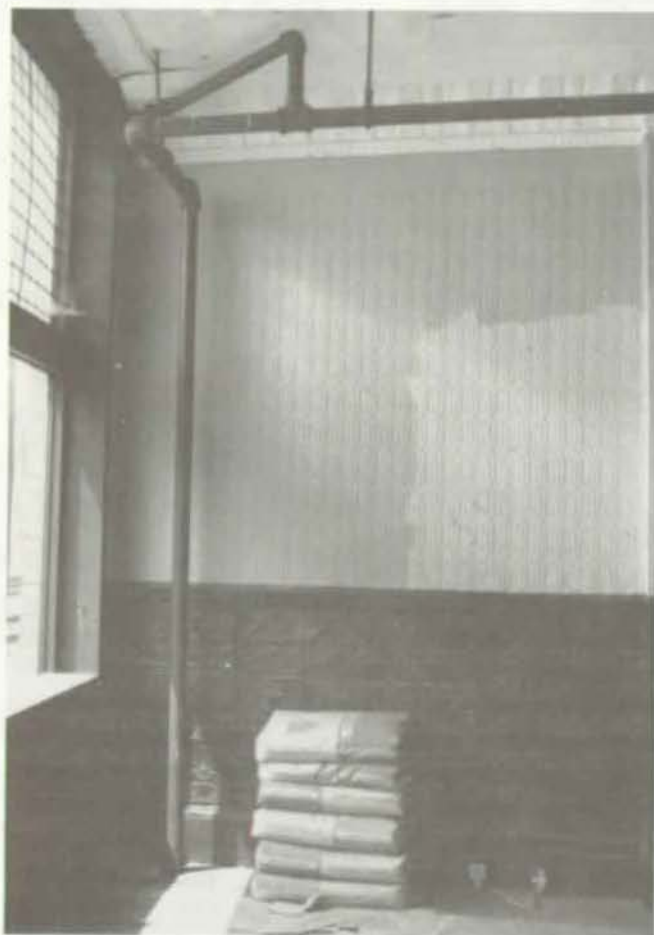
Figure 22 Pressed Tin Panels, Room 101, Mankin-Cox Building, April 1991 (NPS Photo)
