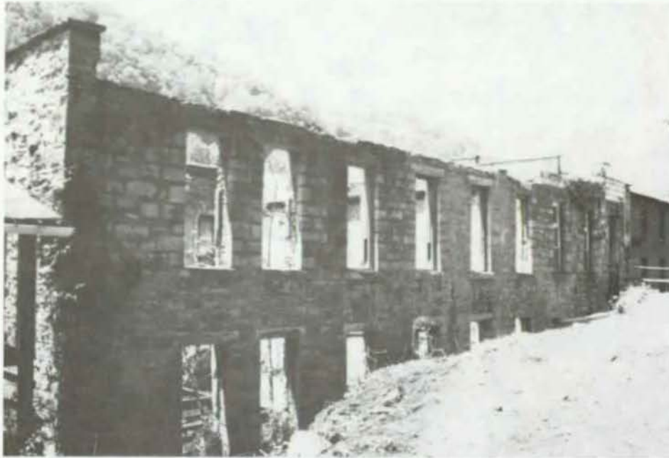
Figure 54 East Elevation, Goodman-Kincaid Building, May 1990 (NPS Photo)
