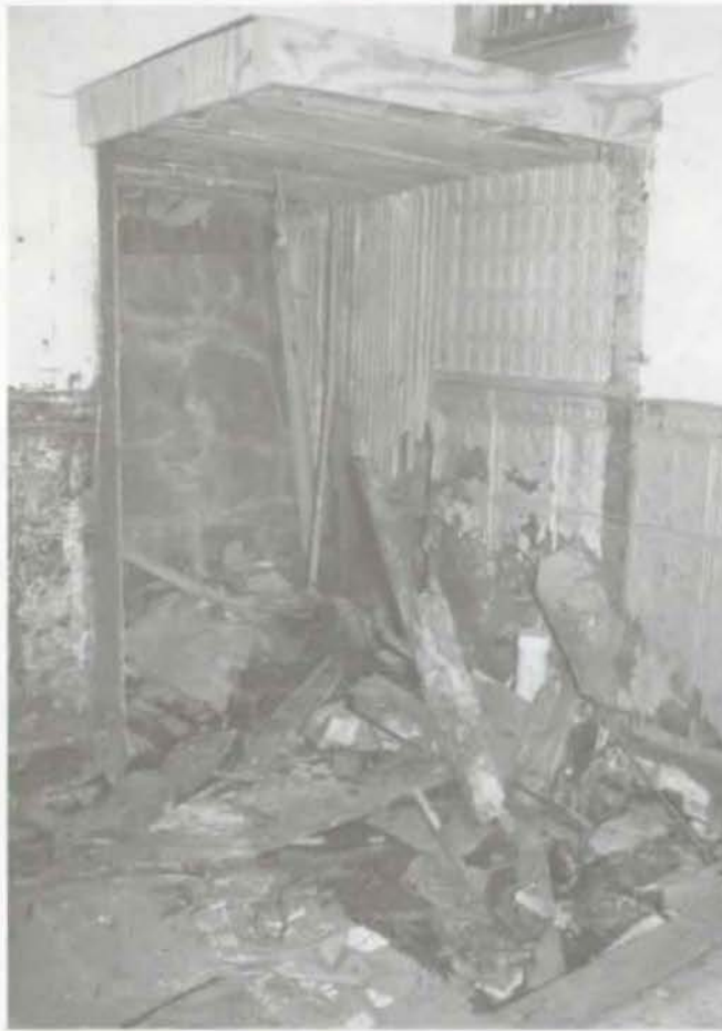
Figure 29 Room 105, Mankin-Cox Building, April 1991 (NPS Photo)
