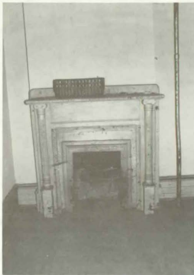
Figure 31 Mantle, Room 203, Mankin-Cox Building, May 1990 (NPS Photo)
