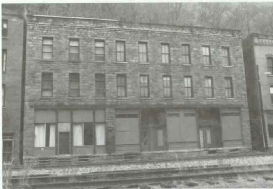
Figure 52 West Elevation, Goodman-Kincaid Building, April 1991 (NPS Photo)
