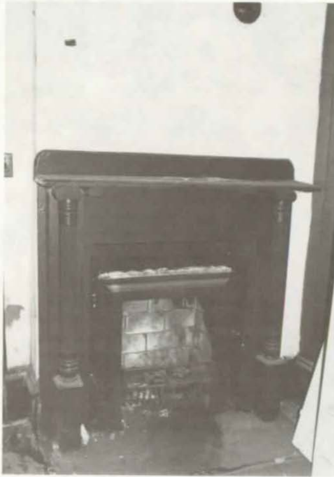
Figure 36 Mantle, Room 211, Mankin-Cox Building, May 1990 (NPS Photo)
