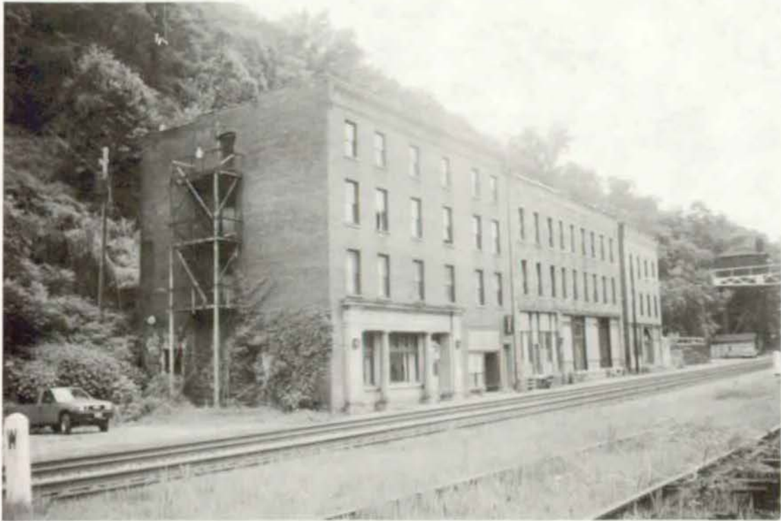
Photograph No. 1: Commercial buildings - west side
