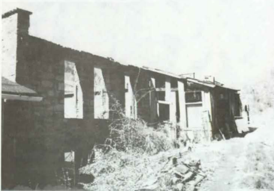
Figure 55 East Elevation, Goodman-Kincaid Building, March 1990 (NPS Photo)
