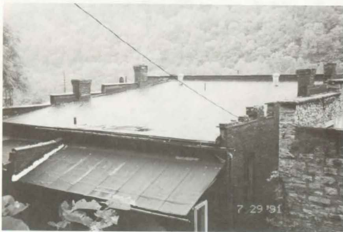
PHOTOGRAPH NO. 13 Mankin-Cox Building - roof
