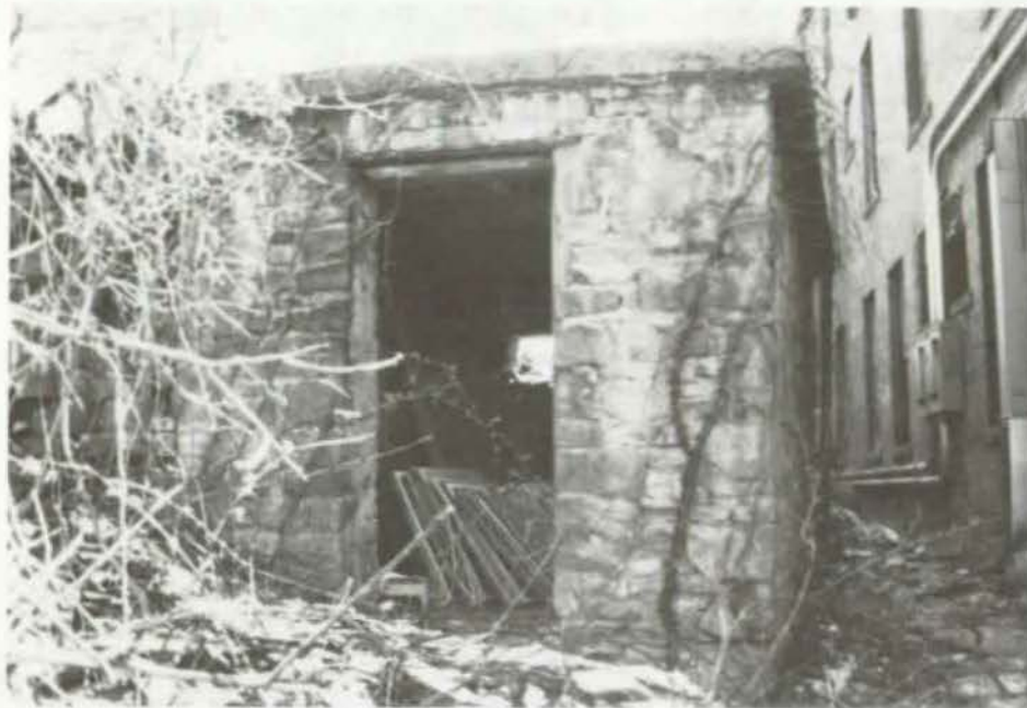
Figure 90 North Elevation, Stone Structure, March 1990 (NPS Photo)
