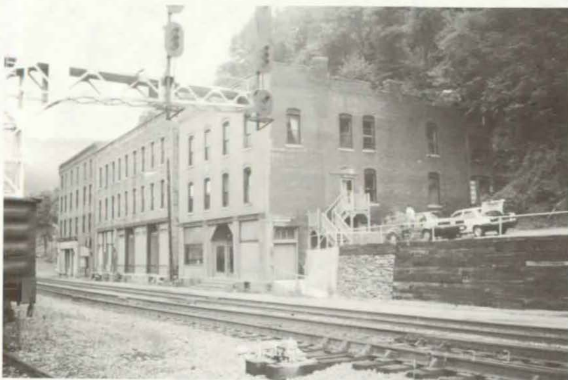
PHOTOGRAPH NO. 2: Commercial buildings - east side
