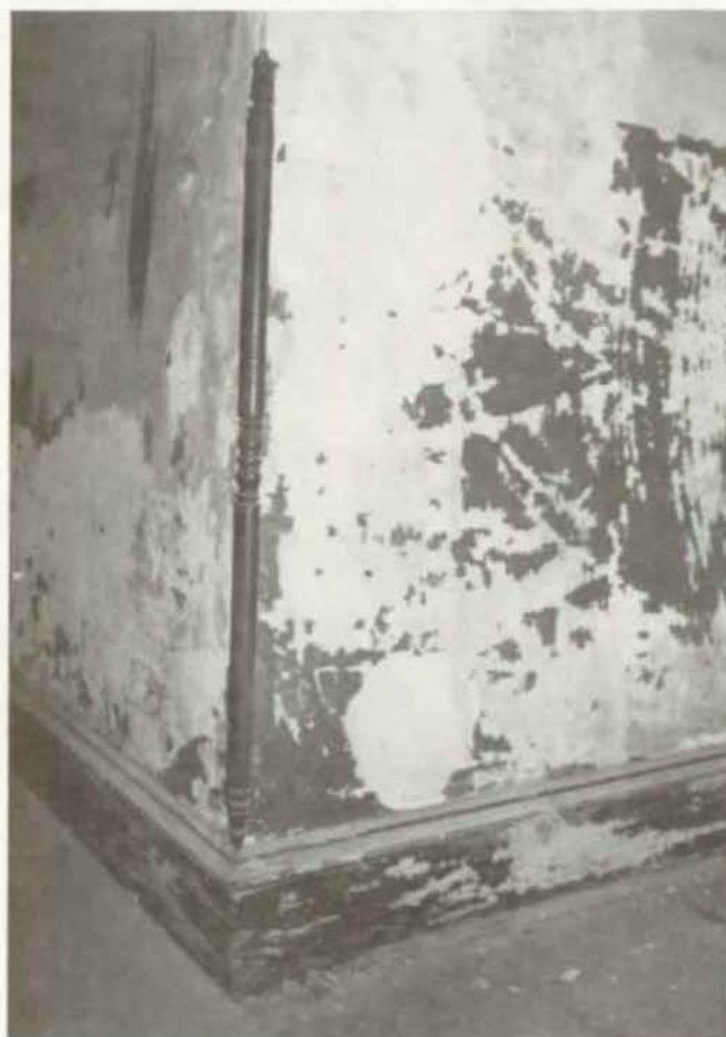
Figure 40 Wood Corner Guards, Mankin-Cox Building, April 1991 (NPS Photo)
