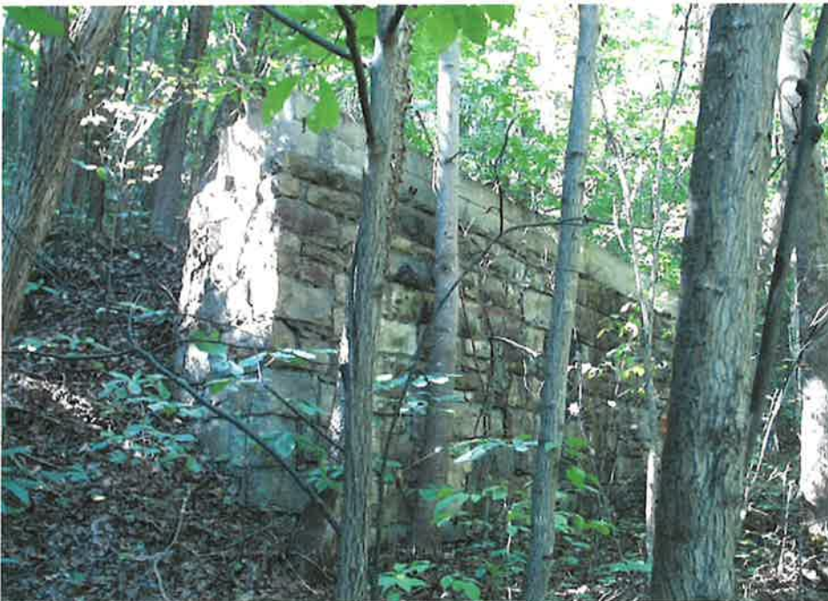
Tipple headwall at Brooklyn (OCLP 2003).
