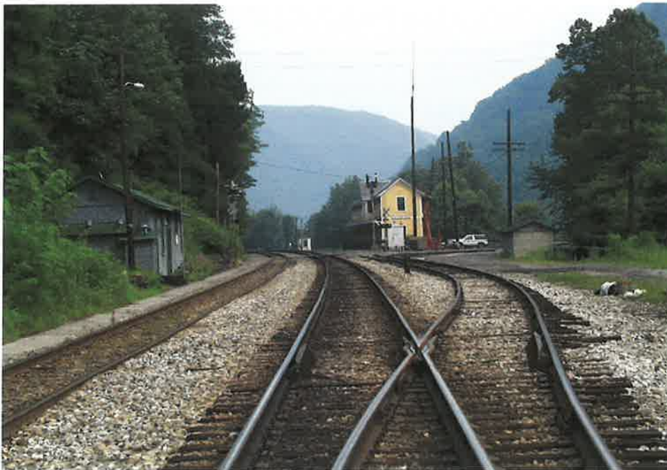
Railroad tracks at Thurmond are still a viable mode of transportation through the park, though passenger trains are less frequent than they were historically (PHSO 2002).
