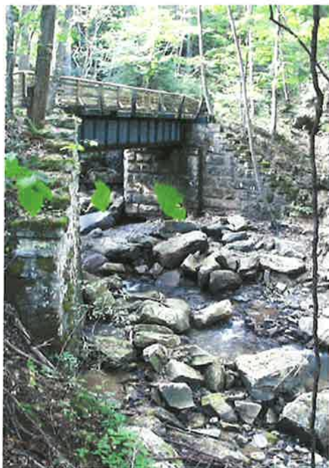
An abandoned rail bridge near Cunard has been adapted for use as a pedestrian trail (OCLP 2003).
