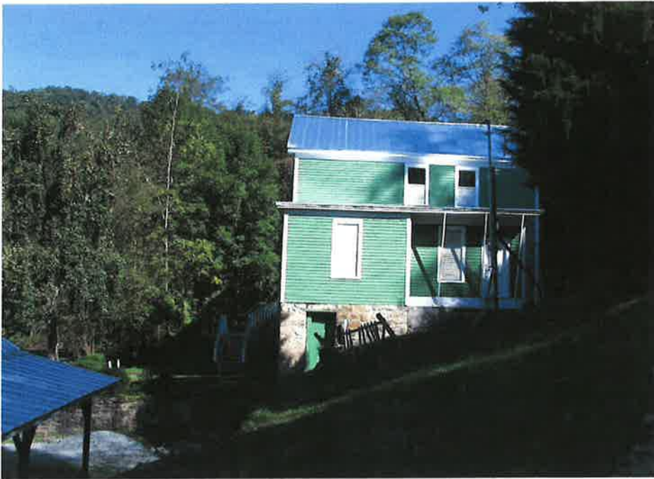
The repainted Fatty Lipcomb House in Thurmond is an example of the stabilization work being done in the park (OCLP 2003).
