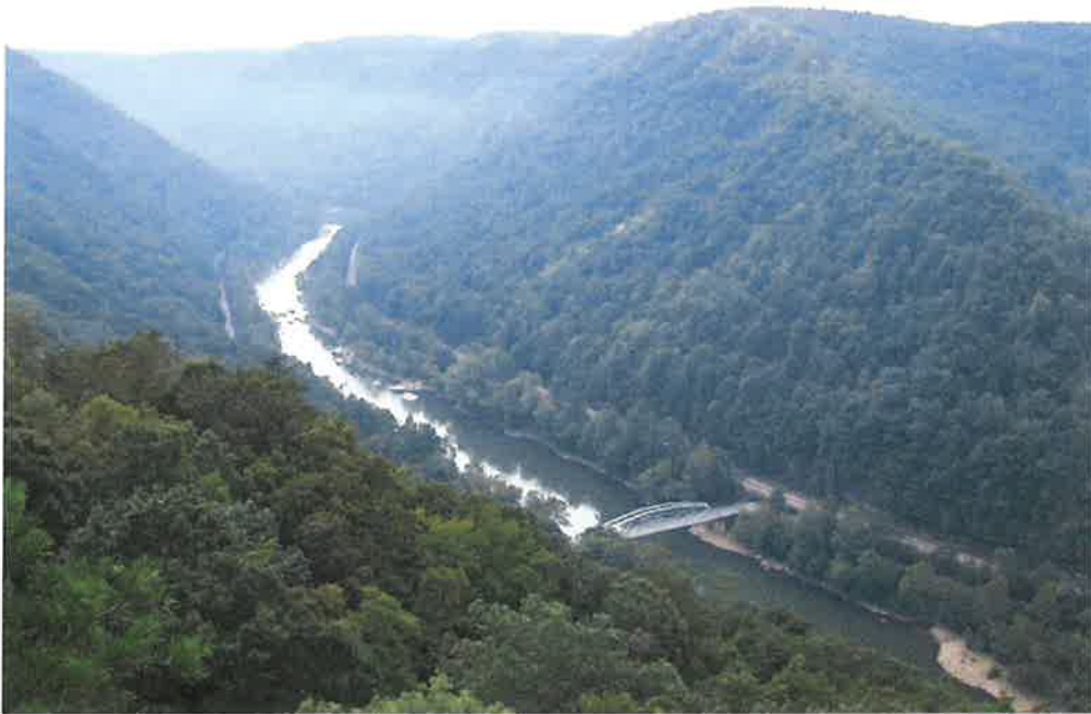
View of the Fayette Bridge from the main overlook at the Canyon Rim Visitor Center (OCLP 2003).
