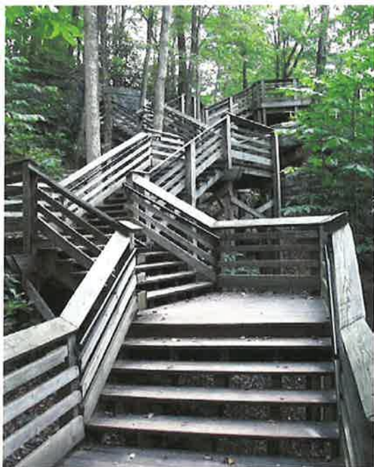
The main overlook boardwalk at the Canyon Rim Visitor Center (OCLP 2003).
