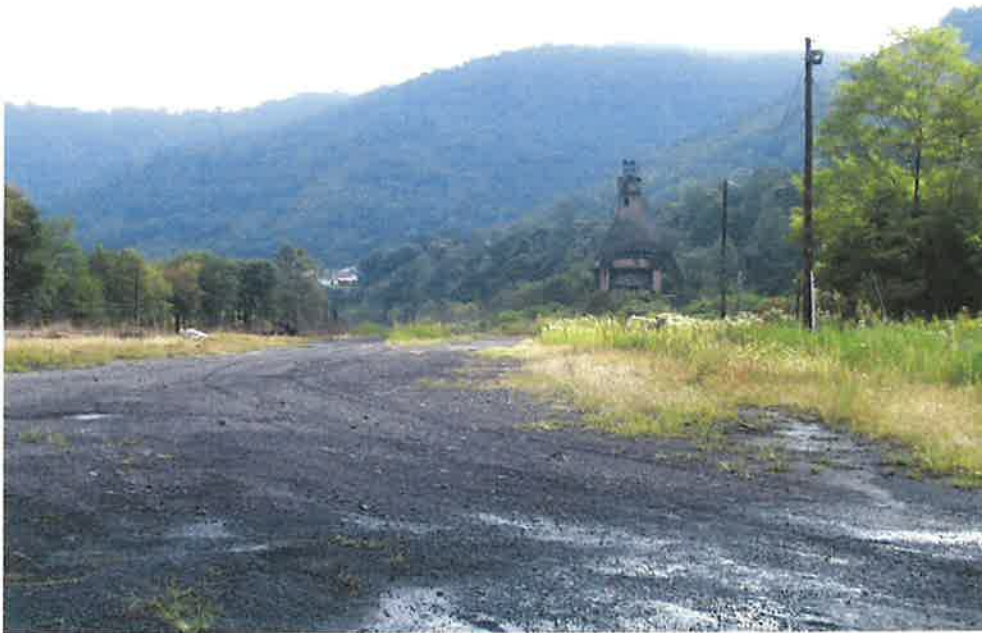
The Hinton coaling tower sits isolated now that many of the CSX tracks have been removed (OCLP 2003).
