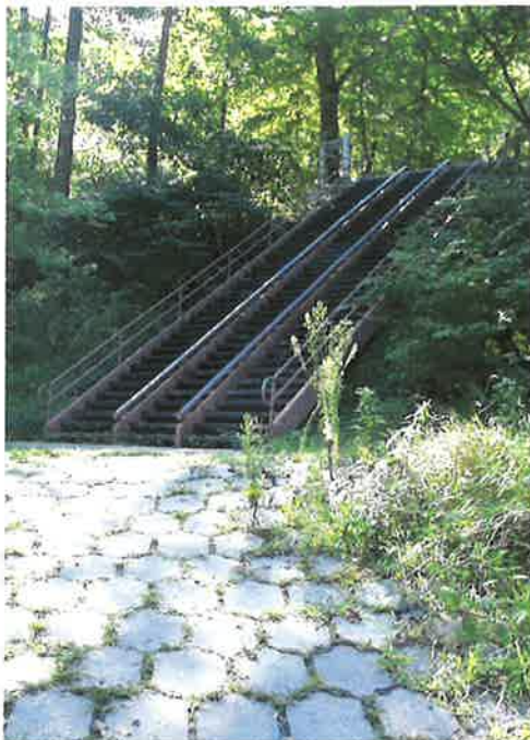
One of the ramps for loading and unloading rafts at Cunard (OCLP 2003).
