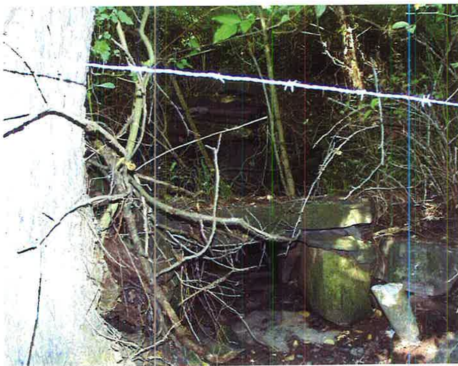
Stone culvert built over stream bed adjacent to barn 1 (PHSO 2001).
