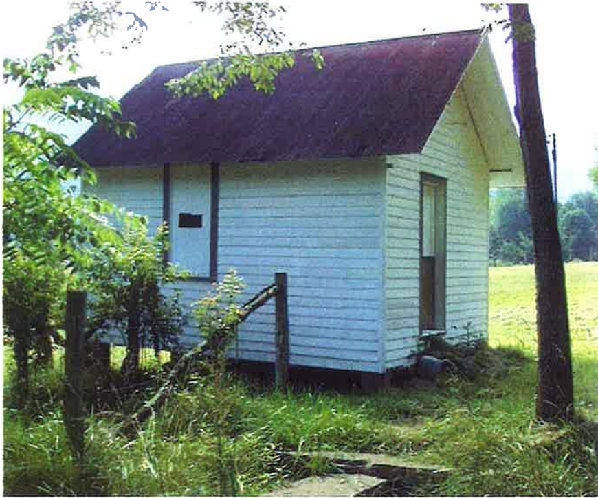
Frame outbuilding looking southeast from stone bridge over stream bed (PHSO 2001).
