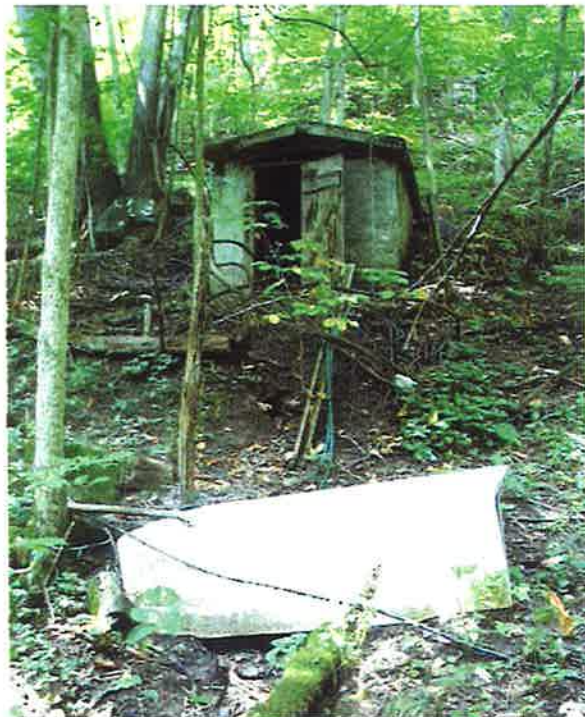
Springhouse located on hillside. (Note tub in foreground, which is mentioned in Small Scale Features section (PHSO 2001).
