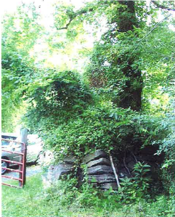
Looking south at gate entrance to farm with Route 26 immediately behind photographer. Understory invasive vegetation typical on the site. Note dry-laid masonry wall mentioned in the Buildings and Structures section of this report (PHSO 2001).
