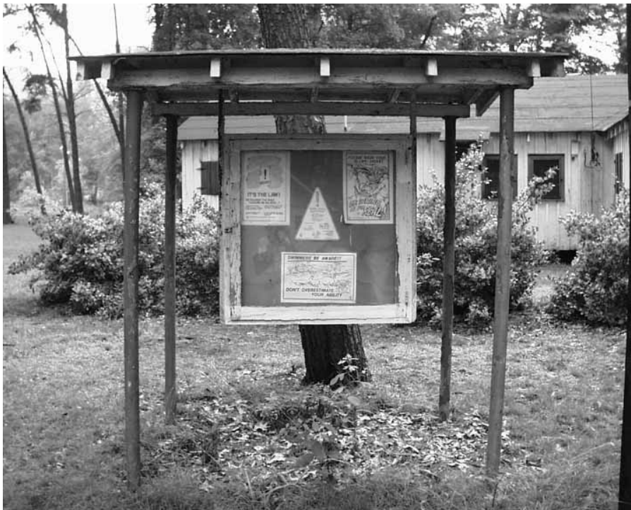
Camp era sign pavilion located adjacent to administration building (PHSO 2001).
