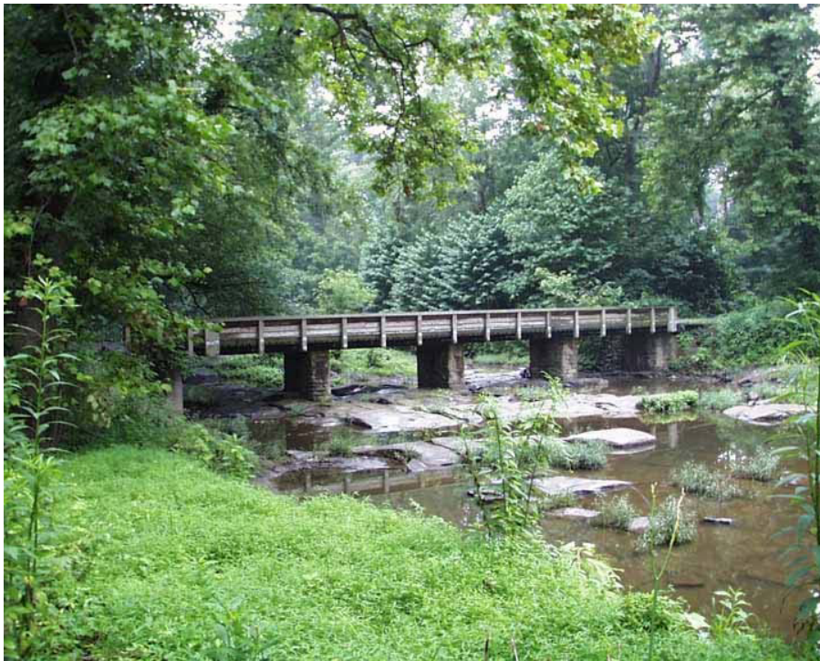
Entry drive bridge crossing mill slough (PHSO 2001).
