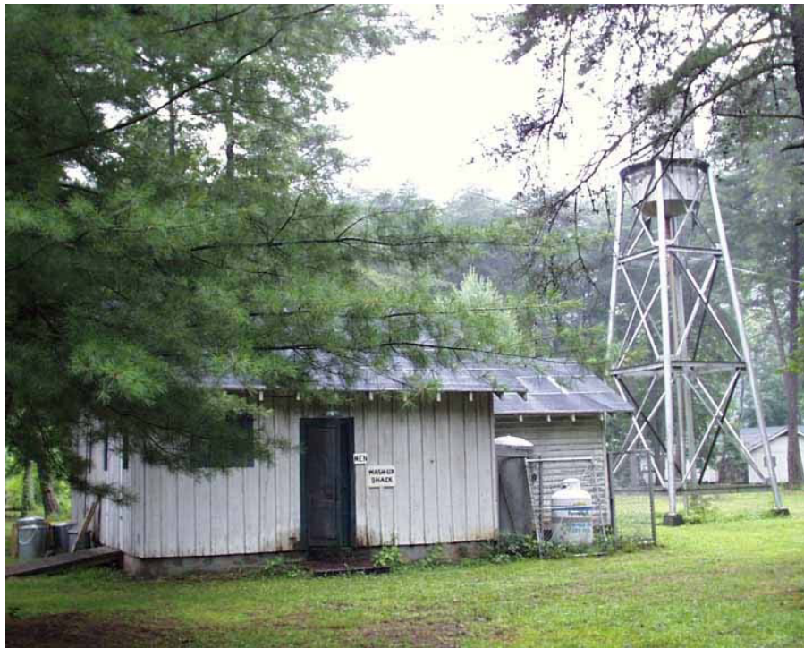
Wash house and water tower (PHSO 2001).
