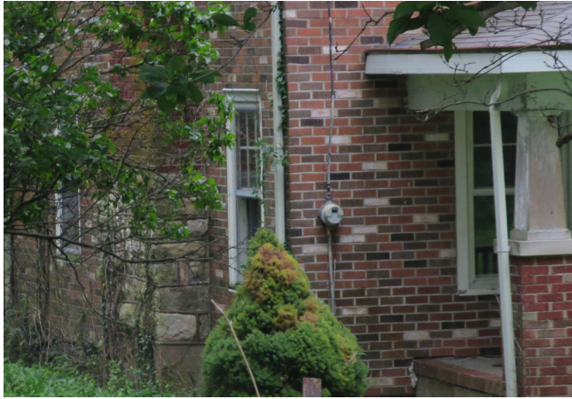
Figure 71. Exterior of House, Looking Northwest at Galvanized Gutter and Downspouts (source: Alvine, 2025)
