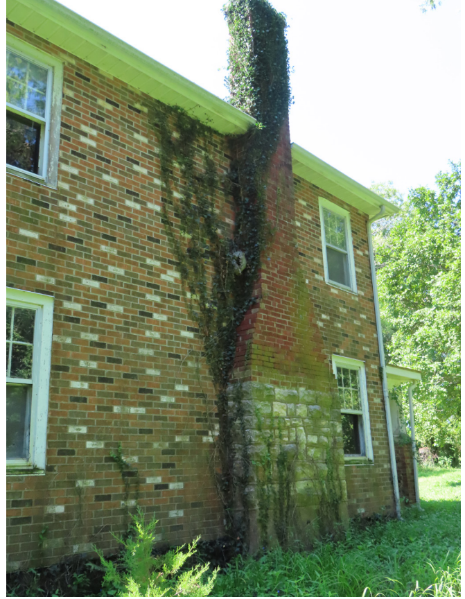
Figure 53. Primary chimney at north wall. (source:RRJ, 2025)
