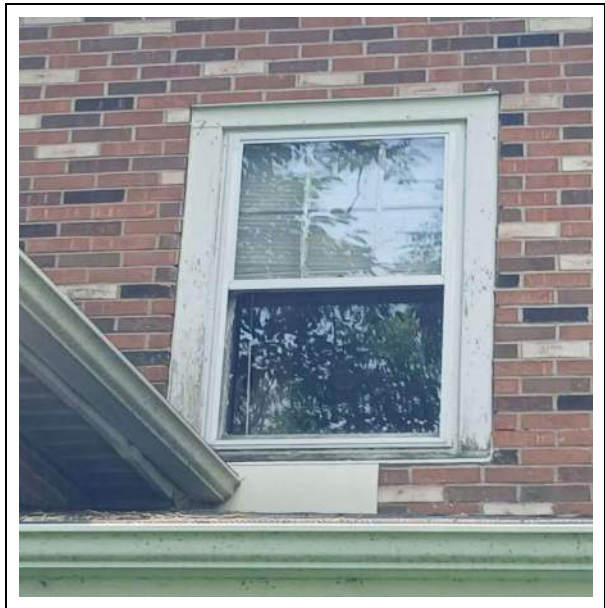
Photograph 12: East exterior building LBP window (Seven panel window, window frame and sill).
