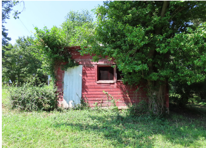
Figure 21. West wall of shed. (source:RRJ, 2025)
