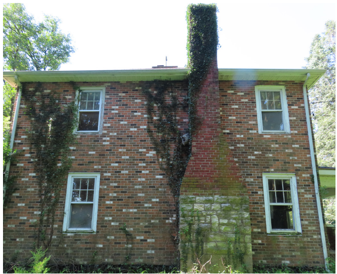
Figure 11. North (side) wall of the Burdick House in July 2025. (source: RRJ, 2025)
