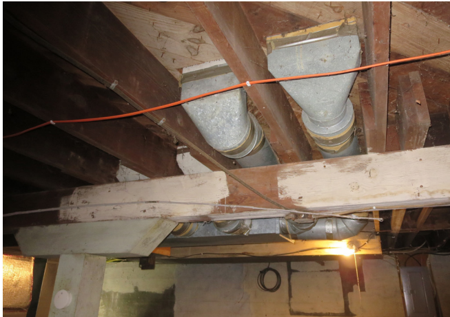
Figure 98. Basement Level, Looking East at Round Branch Air Ducts Offset Up Through the First Level. (source: Alvine, 2025)
