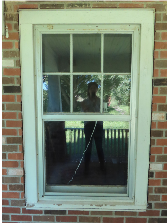
Figure 34. Typical 6-over-1 window unit with aluminum storm window at exterior. (source: RRJ, 2025)
