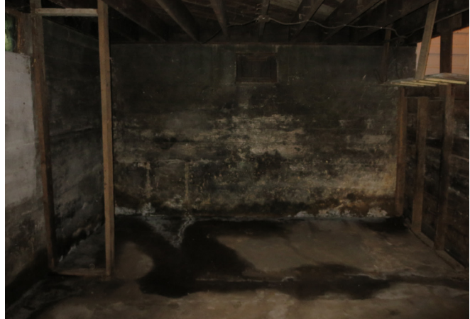
Figure 88. Basement Level, Looking West at Basement Wall Near Northwest Corner Where Coal Door is Located. (source: Alvine, 2025)
