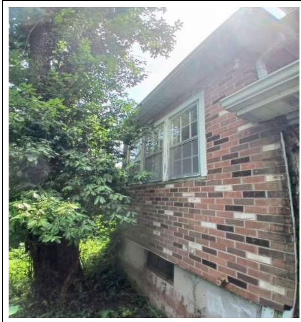
Photograph 9: East exterior building LBP windows (12-seven panel windows, window frames and sills).
