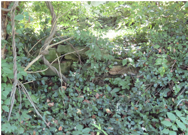
Figure 14. Stone wall at southeast corner of house covered by vegetation. (source:RRJ, 2025)
