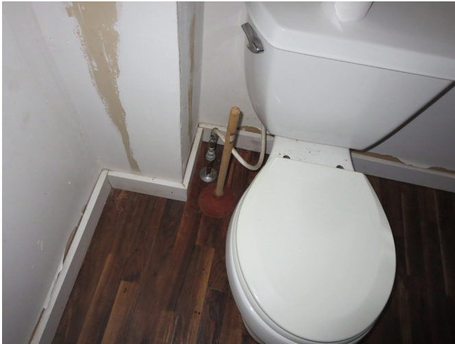
Figure 83. Second Level, Looking Northwest at Floor-Set, Flush-Tank Water Closet at Restroom. (source: Alvine, 2025)
