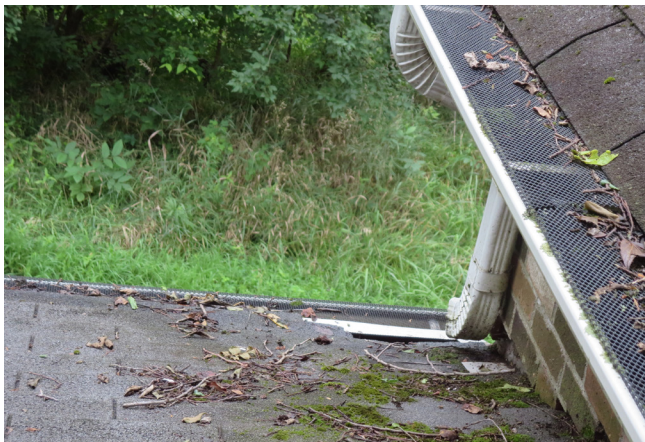
Figure 73. Second Level, Looking West from Stairway to Attic Through Window at Gutter Screen Covers. (source: Alvine, 2025)
