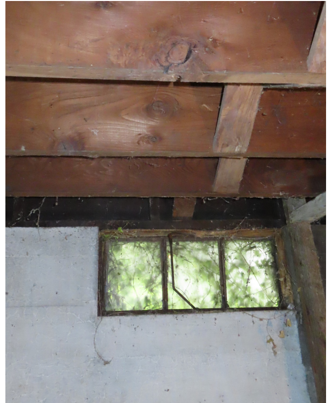
Figure 50. First-floor framing with diagonal bracing between joists. (source: RRJ, 2025)
