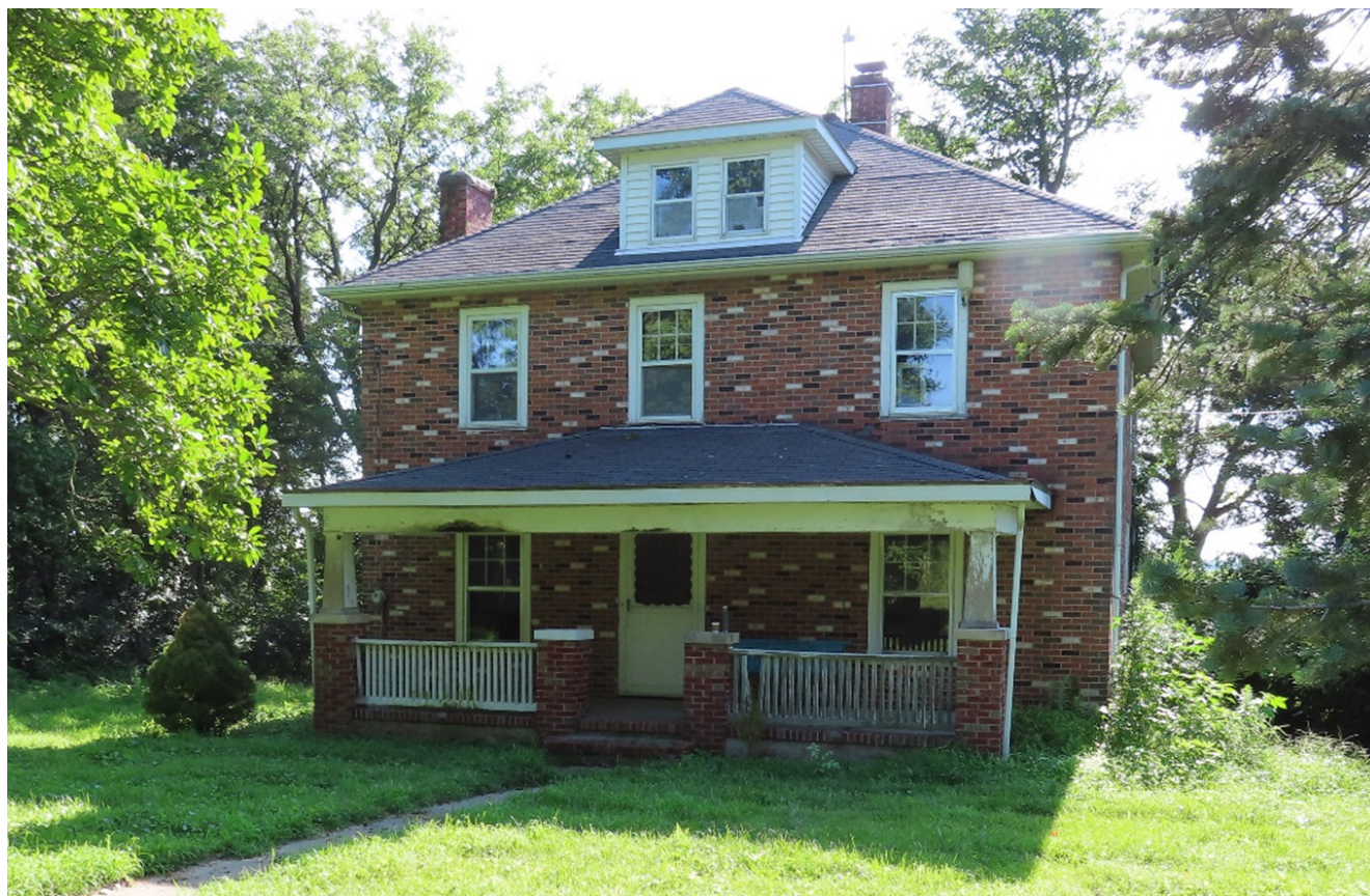
Burdick House, west wall
