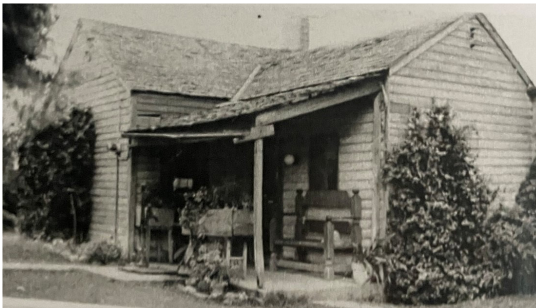
Figure 6. An image of the c. 1800s Burdick house, possibly taken in 1941 before construction of the new Burdick house. (source: Larry Burdick, "Larry Burdick Remembers New Philadelphia," in "Free Frank" McWorter and the "Ghost Town" of New Philadelphia, Pike County, Illinois (1992; Pike County Historical Society, 2023),
