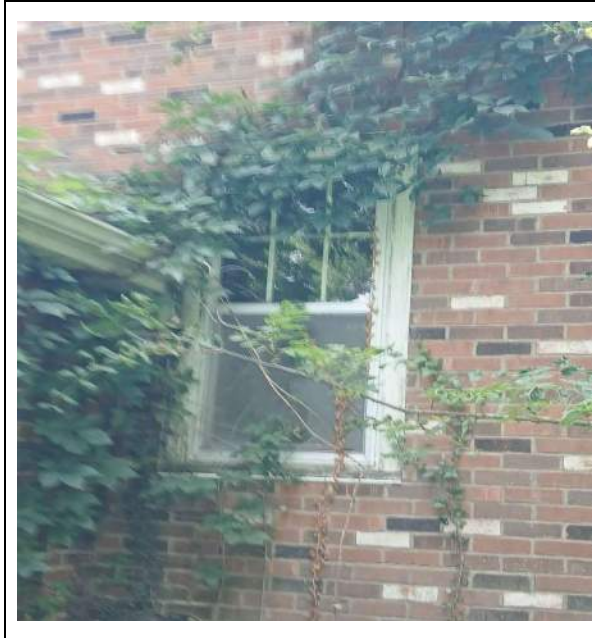
Photograph 13: South exterior building LBP Seven-pane window, window frame and sill.
