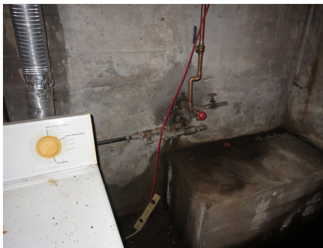
Figure 58. Basement, Looking at South Wall Where Water Service Enters House. (source: Alvine, 2025)
