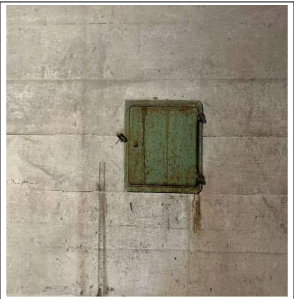
Photograph 24: Basement LBP coal chute door and frame
