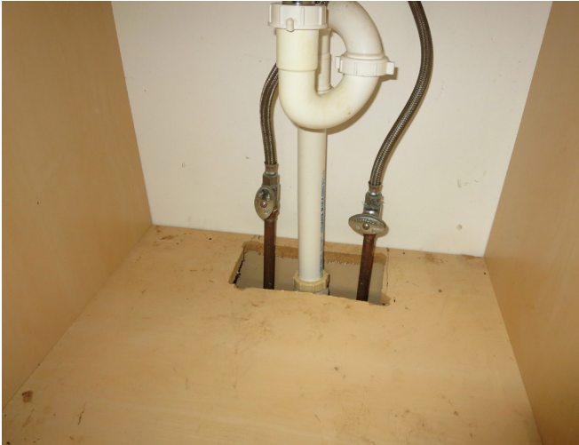
Figure 62. First Level, Looking East at Piping Below Restroom Lavatory. (source: Alvine, 2025)
