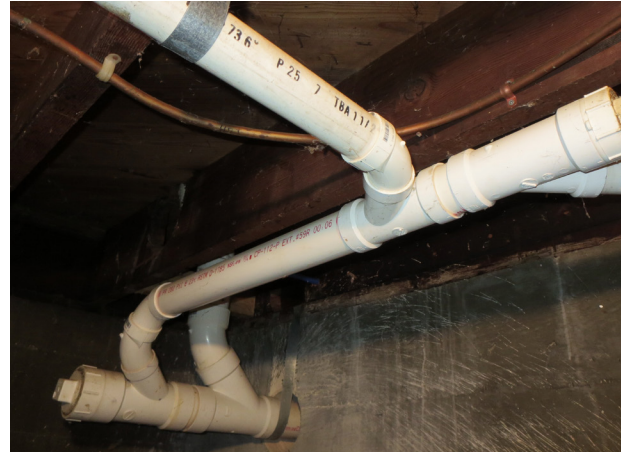
Figure 66. Basement Level, Looking Northwest at Sanitary Piping Serving First Level Restroom Where Piping Exits the House. (source: Alvine, 2025)
