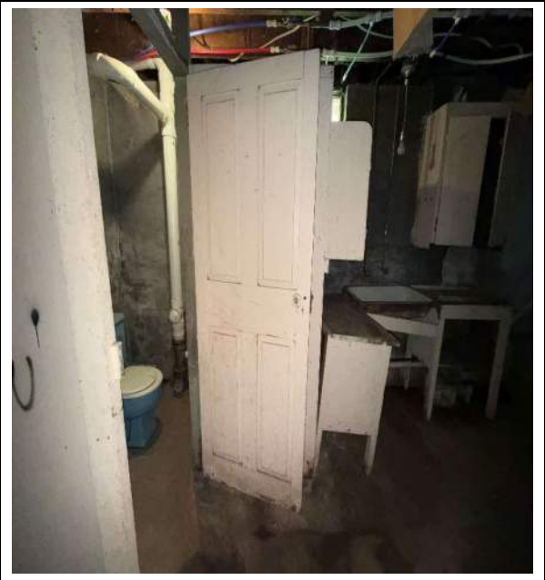
Photograph 22: Basement LBP bathroom door and door frame.
