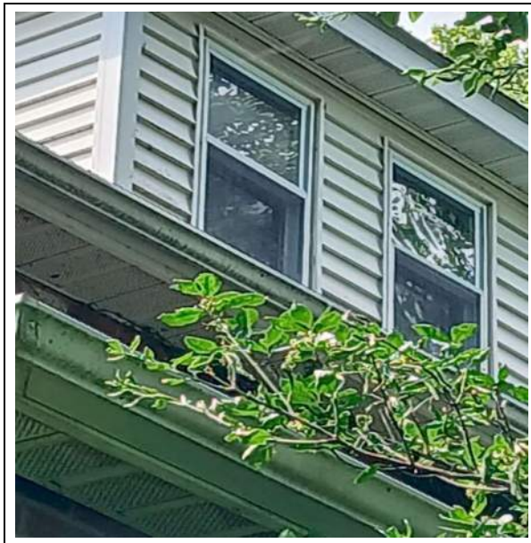
Photograph 15: South exterior attic windows vinyl non-LBP.
