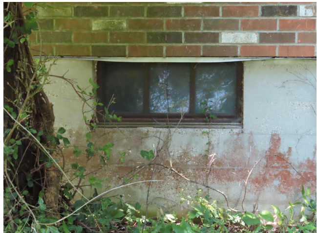
Figure 35. Typical basement level window. (source: RRJ, 2025)
