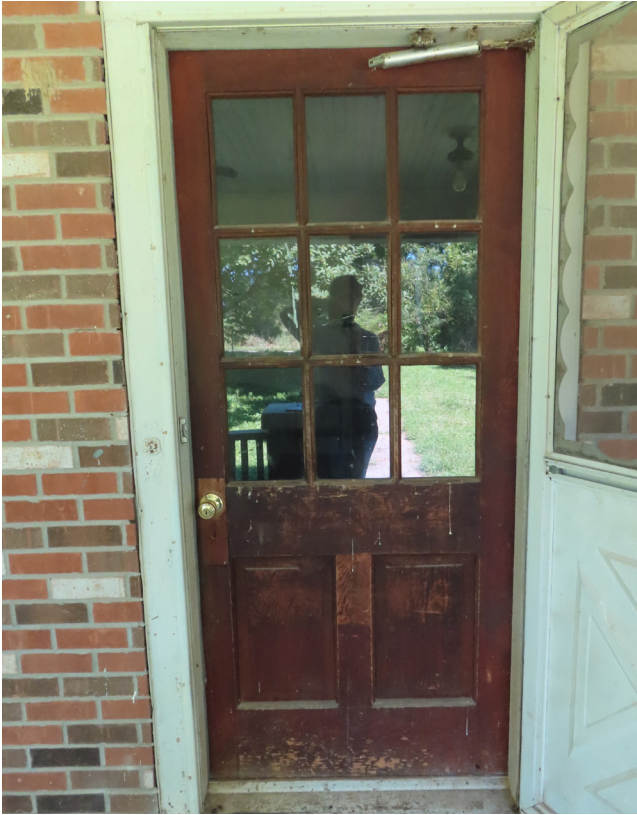
Figure 38. Main entrance door with 9-lite upper panel and lower wooden raised panels. (source: RRJ, 2025)
