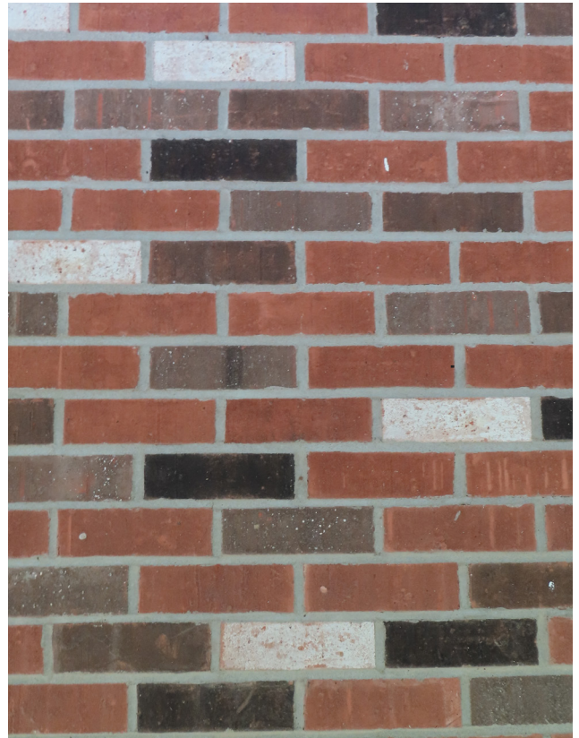
Figure 28. Multi-colored thin brick veneer panel. (source: RRJ, 2025)
