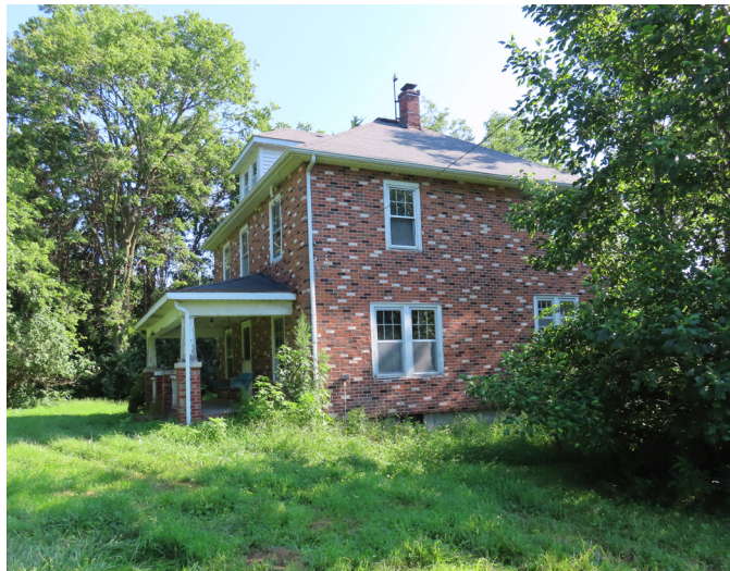
Figure 13. South (side) wall of the Burdick House in July 2025. (source: RRJ, 2025)
