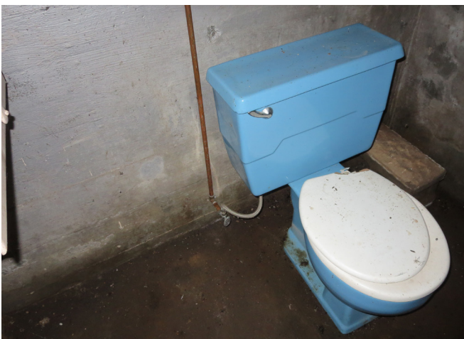
Figure 75. Basement Level, Looking Northwest at Floor-Set, Flush-Tank Water Closet at Makeshift Restroom. (source: Alvine, 2025)
