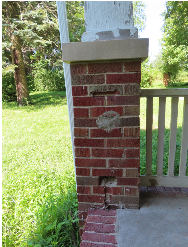
Figure 32. Southwest porch column with rail pockets for former railing. (source: RRJ, 2025)
