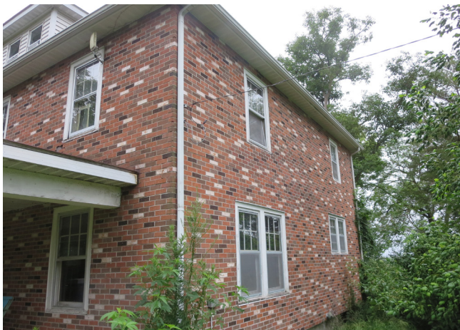
Figure 72. Exterior of House, Looking Southwest at Galvanized Gutters and Downspout. (source: Alvine, 2025)
