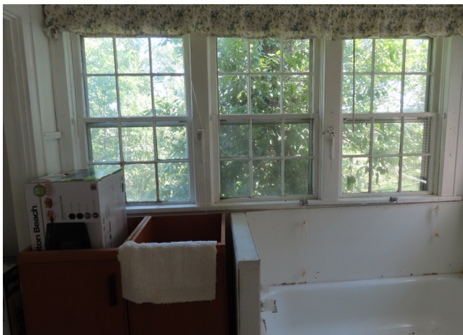
Figure 43. View of Room 106 facing east. (source: RRJ, 2025)
