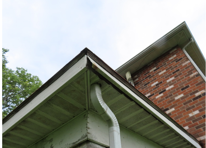
Figure 25. Downspouts at main roof and front porch roof of the house. (source: RRJ, 2025)
