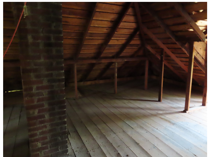
Figure 47. View of Room 301 facing southwest with dormer at right. (source: RRJ, 2025)
