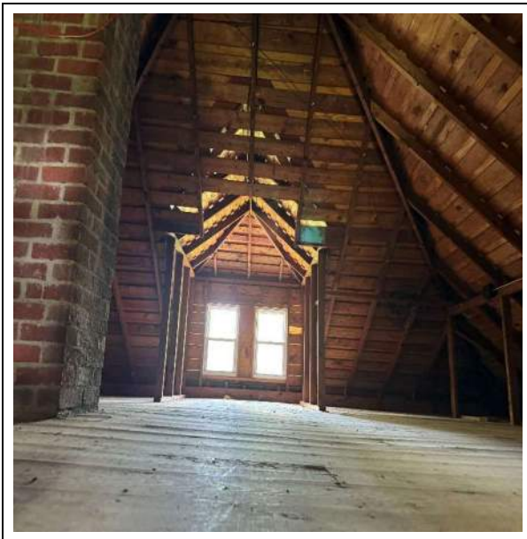
Photograph 39: View of attic with non-LBP vinyl windows.
