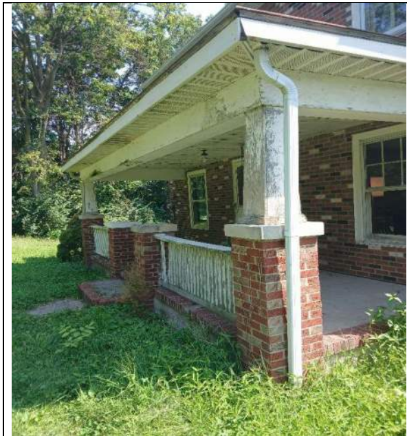
Photograph 3: Exterior Front Porch (ceiling, fascia, posts, bottom rail, balusters, and pillar caps all LBP).
