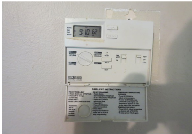
Figure 110. First Level, Looking West at the Wall Where the Furnace Control Thermostat Resides. (source: Alvine, 2025)
