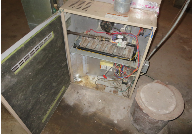
Figure 91. Basement Level, Looking South at Furnace Interior, Indicating Furnace Conditions. (source: Alvine, 2025)
