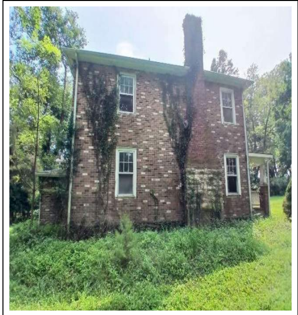
Photograph 14: West exterior building LBP seven-pane windows, window frames, and sills.
