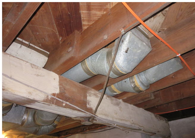
Figure 97. Basement Level, Looking Southeast at Round Branch Air Ducts Offset Up Through the First Level. (source: Alvine, 2025)
