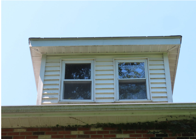
Figure 36. Roof dormer with replacement vinyl windows. (source: RRJ, 2025)
