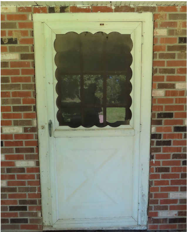
Figure 39. Main entrance door with aluminum storm door in closed position. (source: RRJ, 2025)
