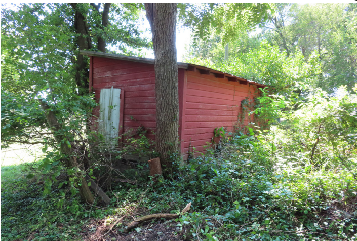
Figure 20. South and east walls of shed.
