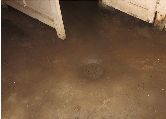
Figure 63. Basement Level, Looking North at Floor Drain Outside Basement Restroom. (source: Alvine, 2025)
