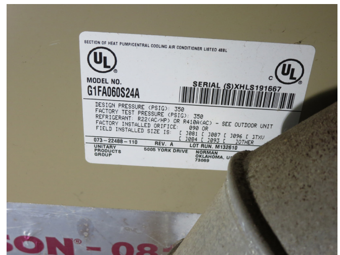
Figure 92. Basement Level, Looking at Furnace Interior Located Manufacturer Informational Sticker. (source: Alvine, 2025)
