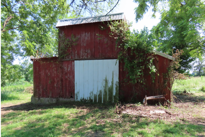
Figure 22. North wall of barn.(source:RRJ, 2025)
