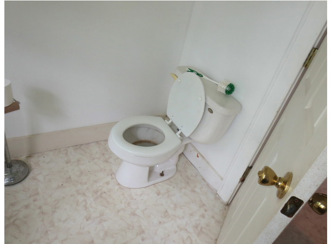
Figure 80. First Level, Looking Northeast at Floor-Set, Flush-Tank Water Closet at Restroom. (source: Alvine, 2025)
