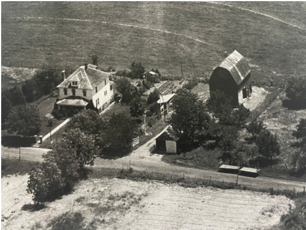
Figure 8. A 1955 aerial image of the Burdick house and outbuildings. (Source: John Drury American Aerial County History Series. Image found on page 126 of McWorter, Gerald A., and Kate Williams-McWorter. New Philadelphia. Path Press, Inc., 2018.)
