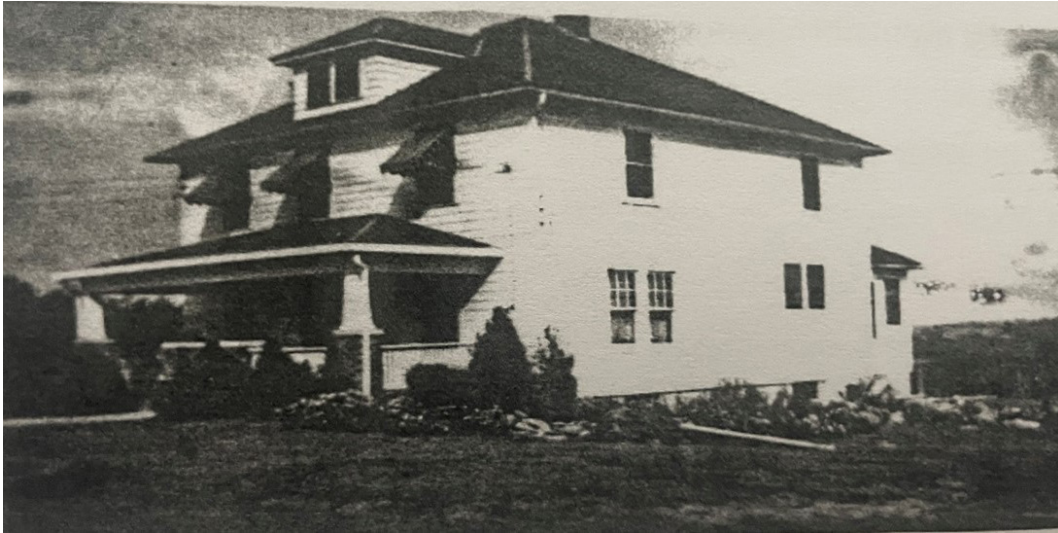
Figure 7. A 1943 view of the Burdick house after completion of the porch, awnings, path, and landscaping. (SOURCE: Image found on page 11 of Matteson, Grace. "Free Frank" McWorter and the "Ghost Town" of New Philadelphia, Pike County, Illinois. 1964; Pike County Historical Society, 2023.)
