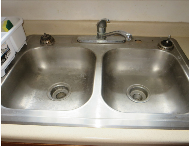
Figure 78. First Level, Looking North at Stainless Steel, Double-Bowl Kitchen Sink. (source: Alvine, 2025)
