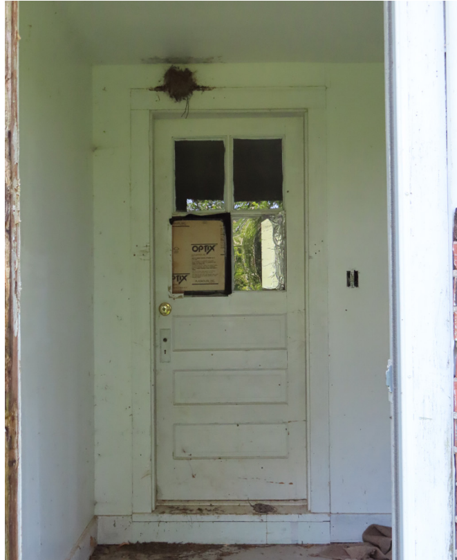
Figure 40. Original exterior door at rear enclosed porch. (source: RRJ, 2025)
