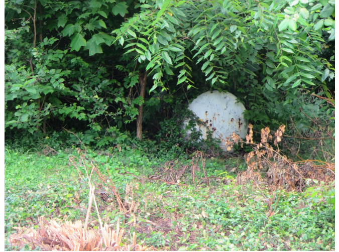
Figure 86. Exterior of House, Looking West at Existing Propane Tank. (source: Alvine, 2025)
