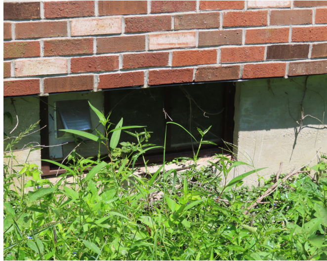
Figure 48. Exterior of cast in place board formed concrete foundation wall with inset basement window and brick veneer above. (source: RRJ, 2025)
