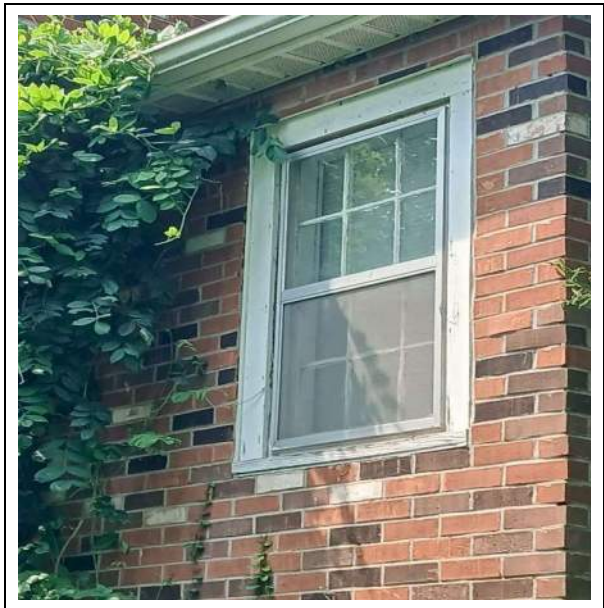
Photograph 8: North exterior building LBP windows (12-seven panel window, window frame and sill).
