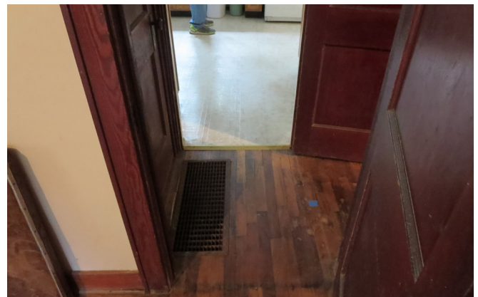
Figure 103. First Level, Looking South at Floor Located Grille at Base of Stairway to Second Level . (source: Alvine, 2025)
