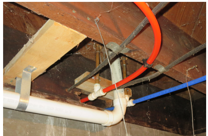
Figure 60. Basement, Looking East From Inside the Room Below the First Level Restroom. (source: Alvine, 2025)
