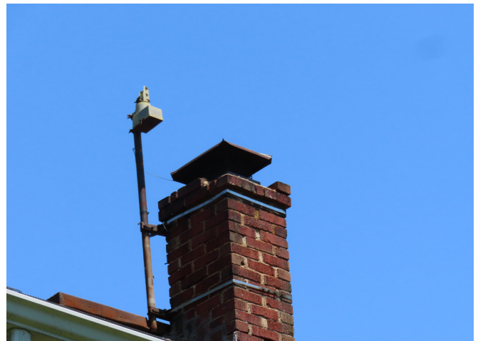
Figure 54. Secondary chimney at center of roof. (source:RRJ, 2025)
