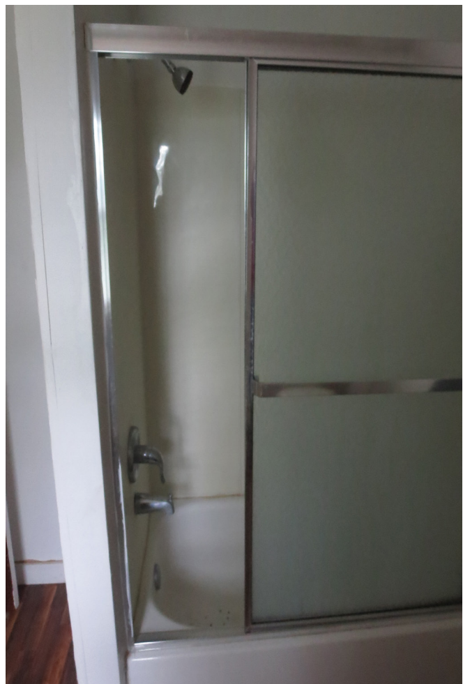
Figure 85. Second Level, Looking South at Bathtub and Shower Enclosure at Restroom. (source: Alvine, 2025)
