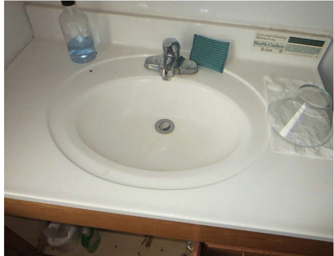
Figure 84. Second Level, Looking Northeast at Counter-Mounted Lavatory at Restroom. (source: Alvine, 2025)
