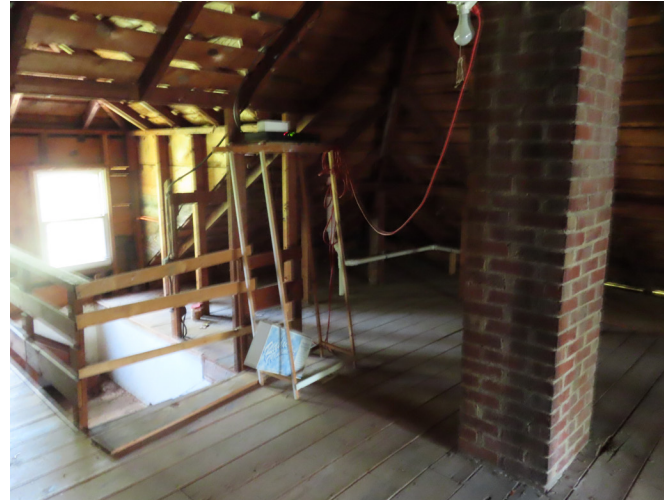
Figure 46. View of Room 301 facing southeast with stairwell at left. (source: RRJ, 2025)
