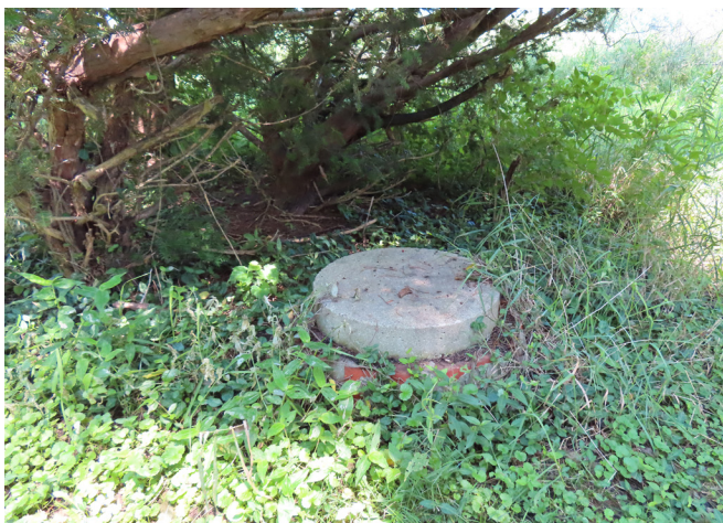
Figure 16. Brick cistern with concrete cap located near southeast corner of the house. (source:RRJ, 2025)
