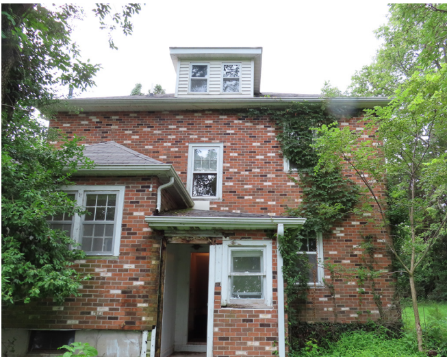
Figure 12. East (rear) wall of the Burdick House in July 2025. (source: RRJ, 2025)
