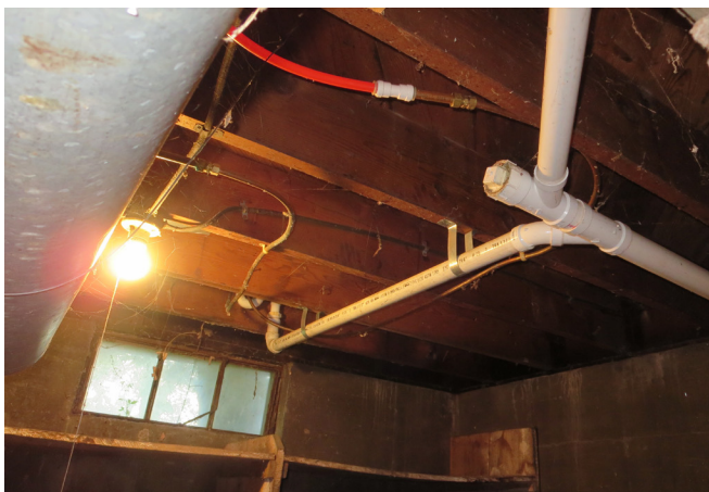
Figure 65. Basement Level, Looking Northwest at Sanitary Piping Serving First Level Restroom Above. (source: Alvine, 2025)
