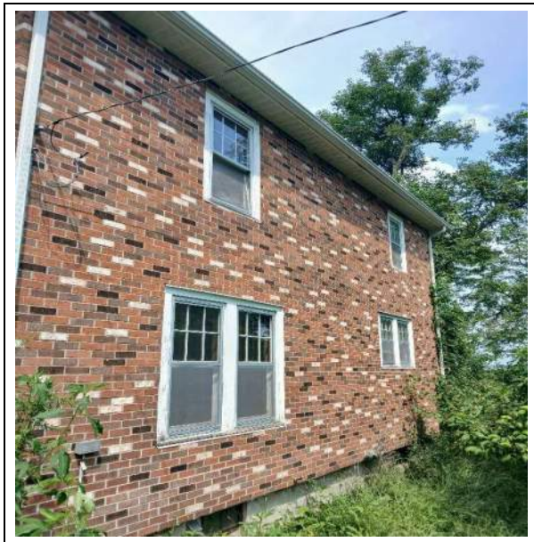
Photograph 7: South exterior building LBP windows (6-seven panel windows, window frames and sills).
