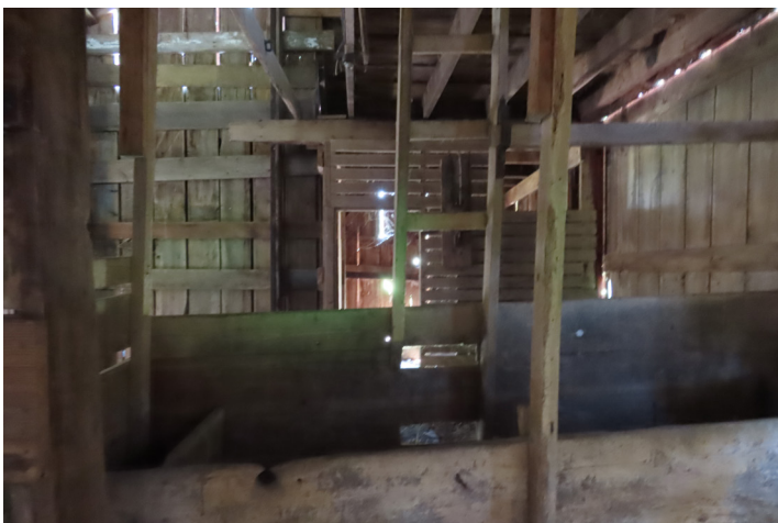
Figure 24. Interior of barn looking north with built-in trough in foreground. (source:RRJ, 2025)
