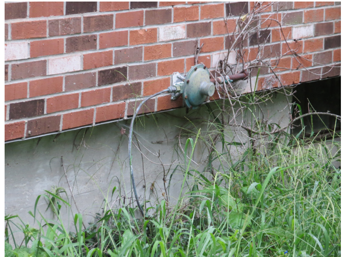
Figure 87. Exterior of House, Looking at North Face of House Propane Meter Location. (source: Alvine, 2025)
