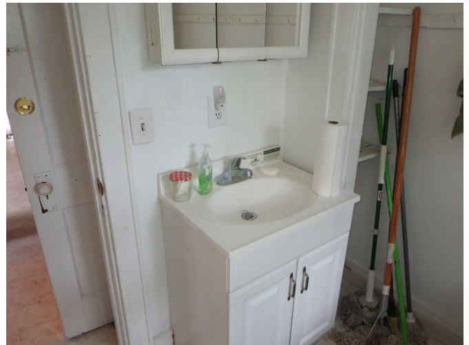
Figure 81. First Level, Looking Southeast at Counter-Mounted Lavatory at Restroom. (source: Alvine, 2025)
