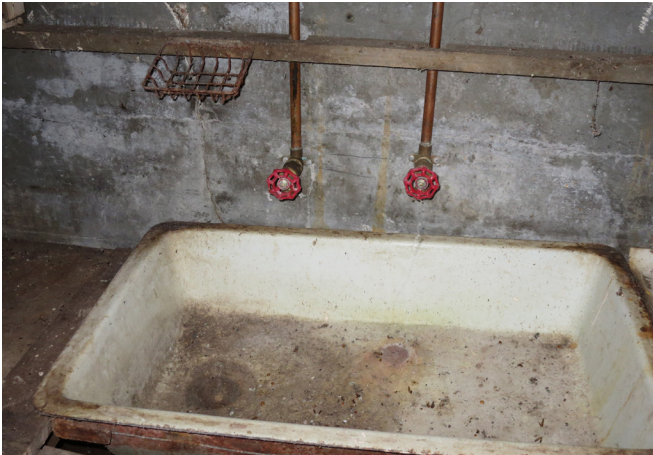
Figure 74. Basement Level, Looking North at Sink and Hose Bibbs Used for Sink Faucet. (source: Alvine, 2025)
