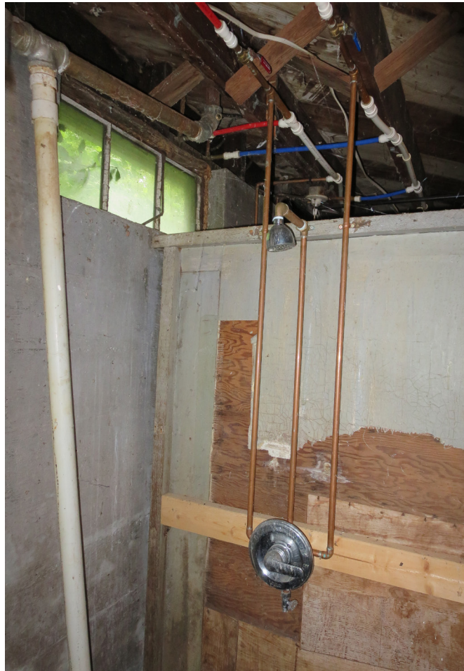
Figure 76. Basement Level, Looking Northwest at Shower Valve and Shower Head at Makeshift Shower Stall. (source: Alvine, 2025)
