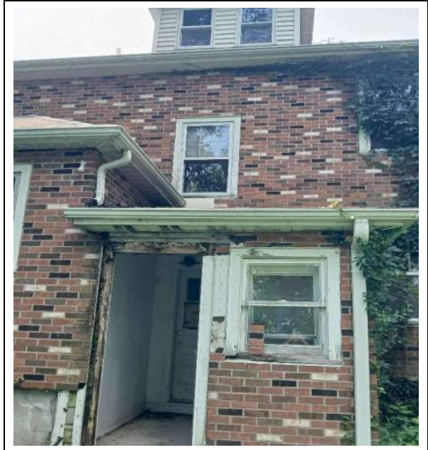
Photograph 10: East exterior building LBP windows (Seven panel window and two-panel windows, window frames and sills).
