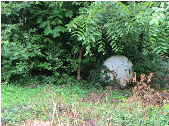
Figure 18. South end of propane tank (covered in vegetation) (source: Alvine, 2025)
