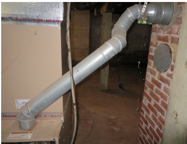
Figure 93. Basement Level, Looking South at Furnace Flue and Connection to Adjacent Chimney. (source: Alvine, 2025)
