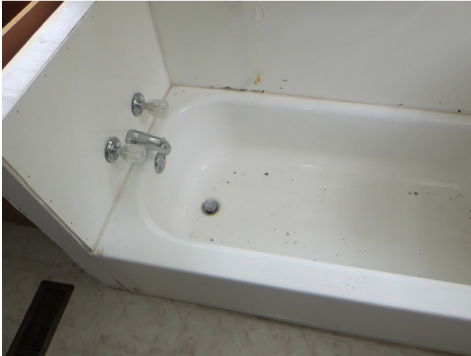
Figure 82. First Level, Looking West at Bathtub Along the West Wall of the Restroom. (source: Alvine, 2025)
