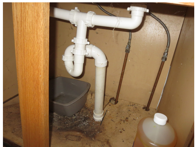
Figure 61. First Level, Looking North at Piping Below the Kitchen Sink. (source: Alvine, 2025)
