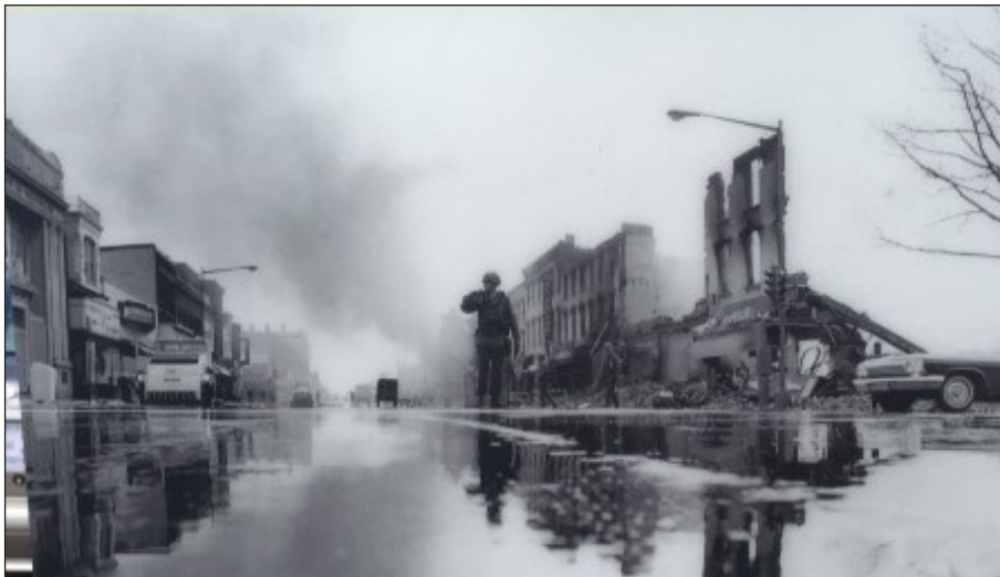
Figure 3. D.C. Riot Damage 1968/ Washington Post
