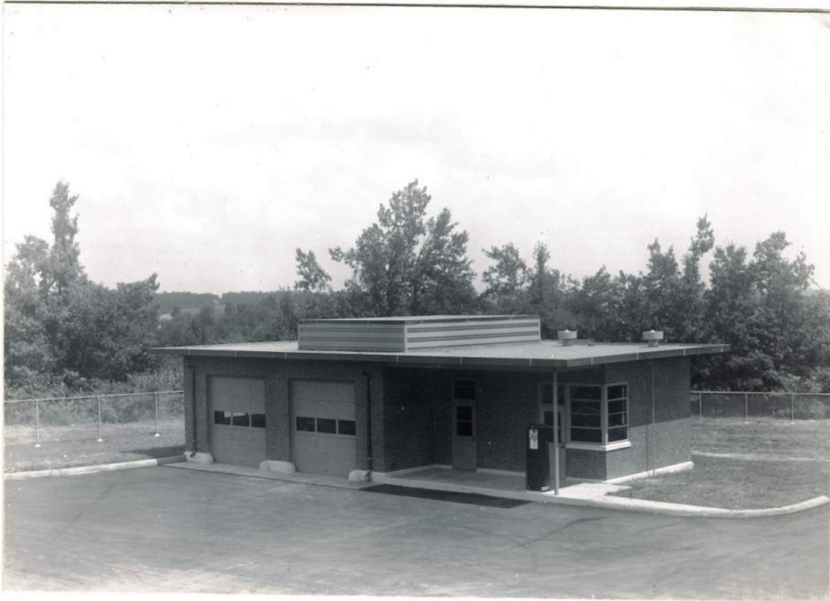
Maintenance Area - Oil and Paint Storage Building
