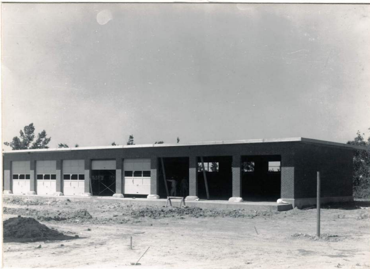
Maintenance Area - Equipment Storage Building
