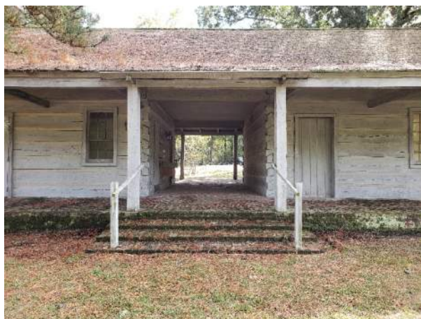
Figure 15. View of north elevation looking through dogtrot.
