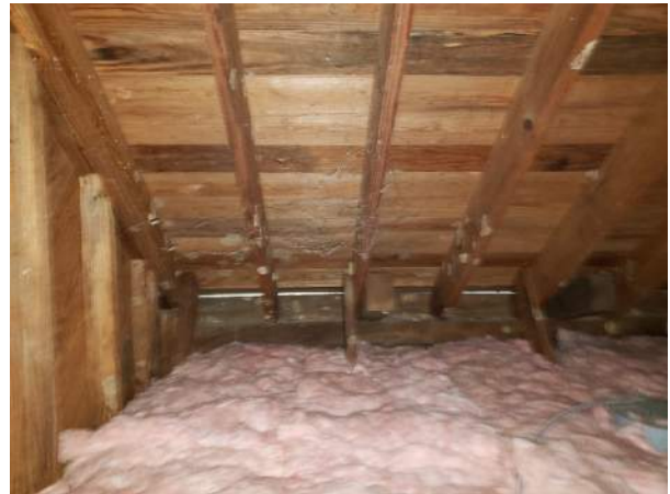
Figure 33. General view of attic.
