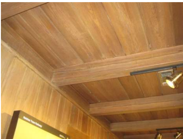
Figure 26. Detail view of exposed wood beams, random width ceiling boards, and vertical wood paneling at upper walls.
