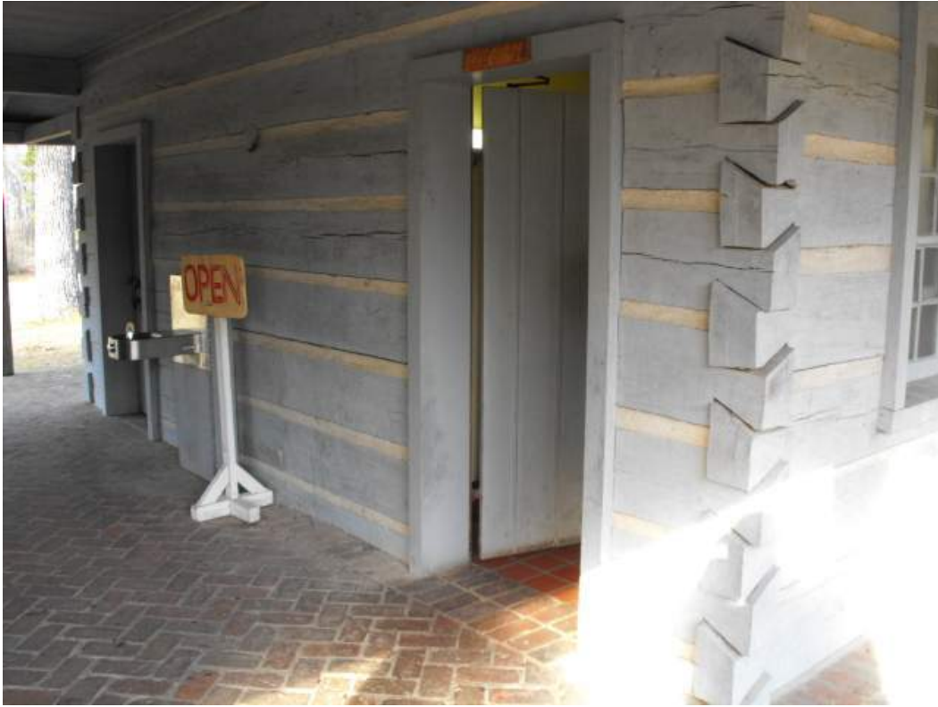
Photo 13: Breezeway area, view of bathroom entrance.
