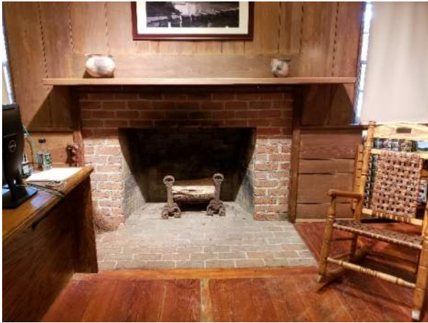
Figure 24. View of fireplace. The mantel shelf does not appear in earliest photograph of room.
