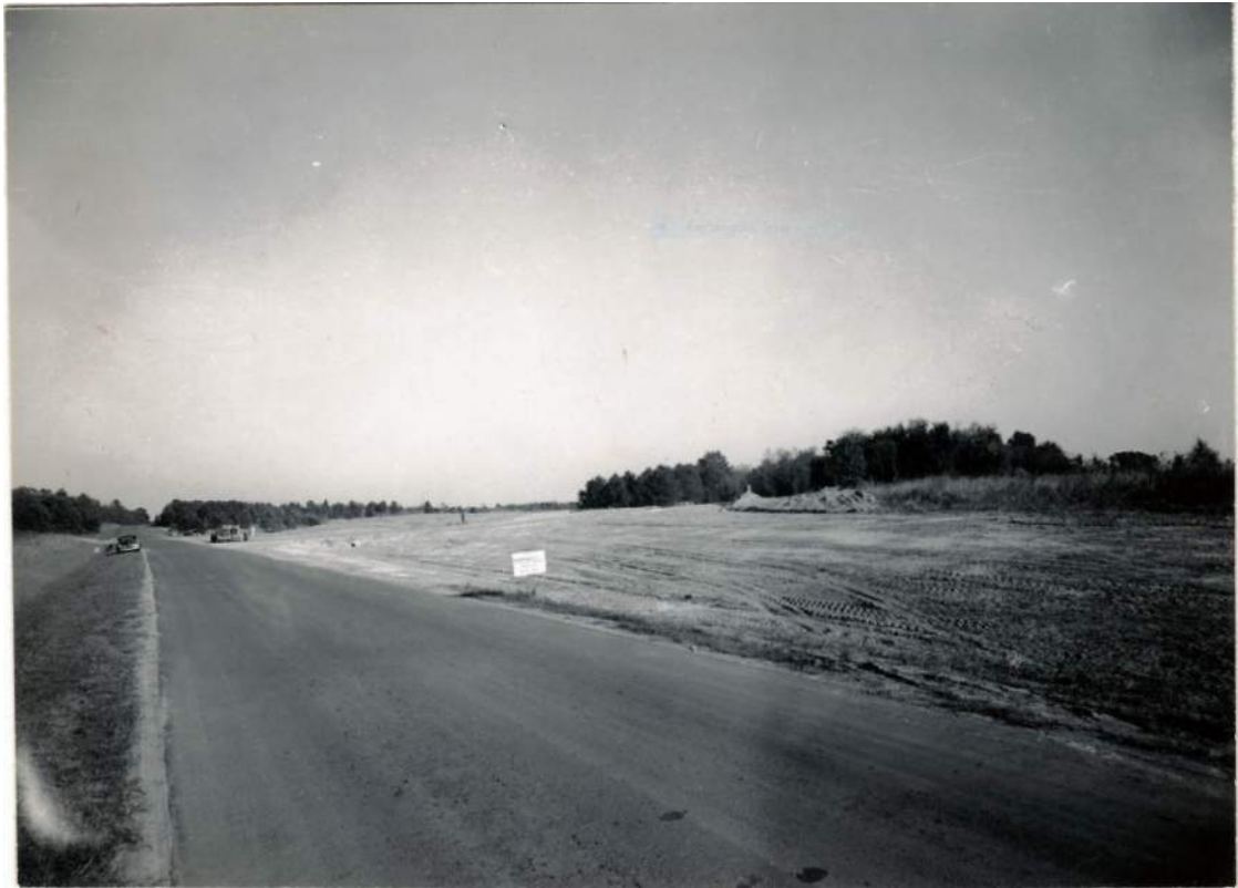
Figure 6. Site of Information Station before construction October 16, 1950. Source: Final Construction Report, Buildings and Incidental work, Ridgeland District Headquarters, Section 3-0, Ridgeland, Miss, Contract no. I-27-27np-333, November 15, 1951. D 2623, FRC Recalled Record Collection, NATR Acc#290, Project Completion Reports-Ridgeland, Box 3, Folder 36A. Natchez Trace Parkway, Tupelo, MS.
