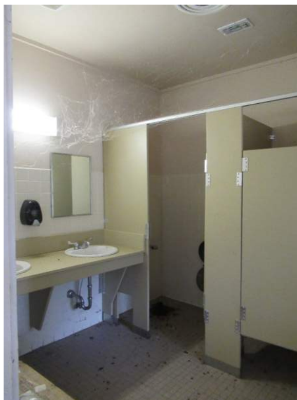
Figure 30. View of Women's Toilet Room.
