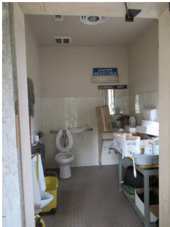
Figure 31. View of Accessible Family Restroom.
