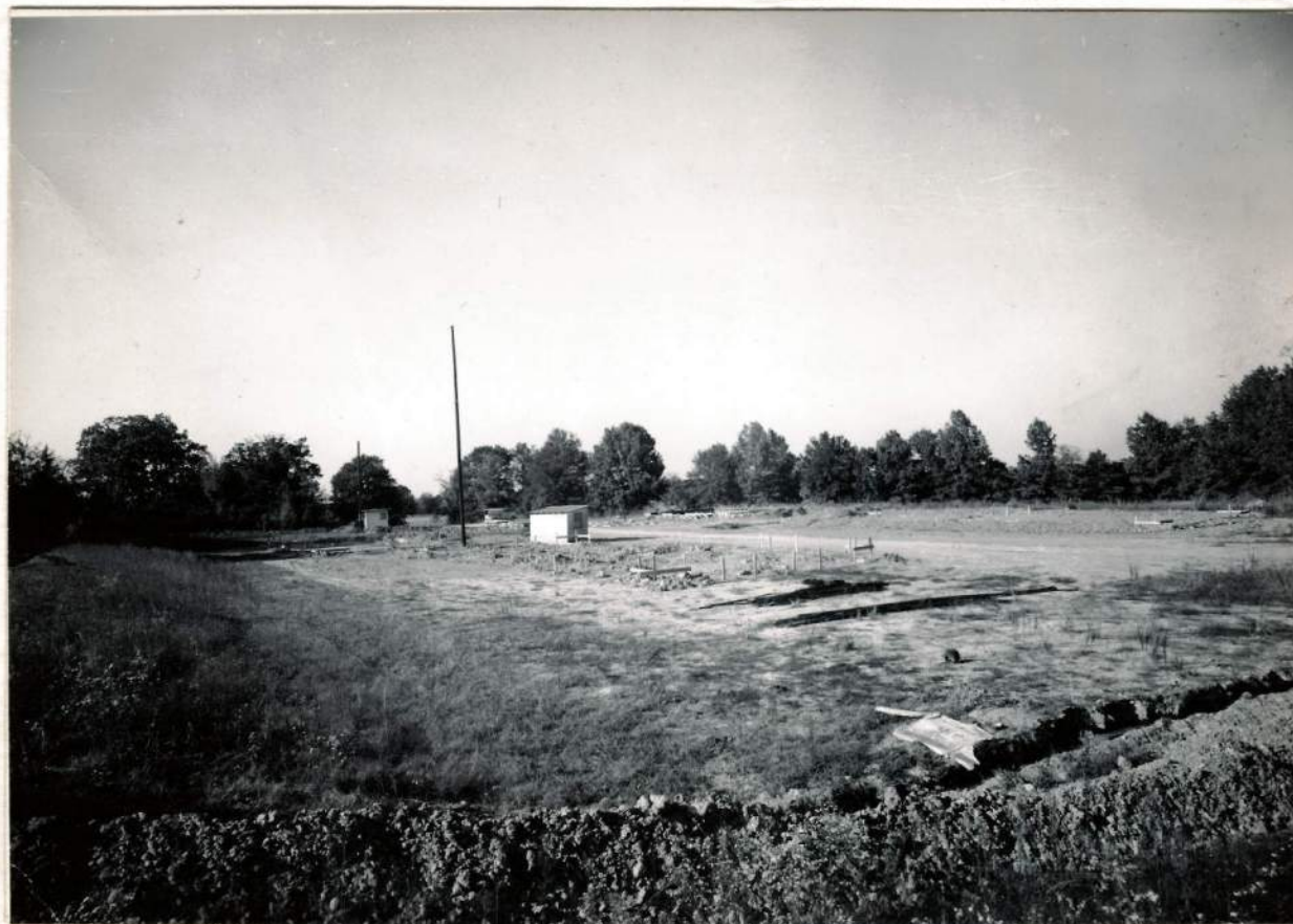
Maintenance Area - Site at Beginning of Construction - 10/16/50
