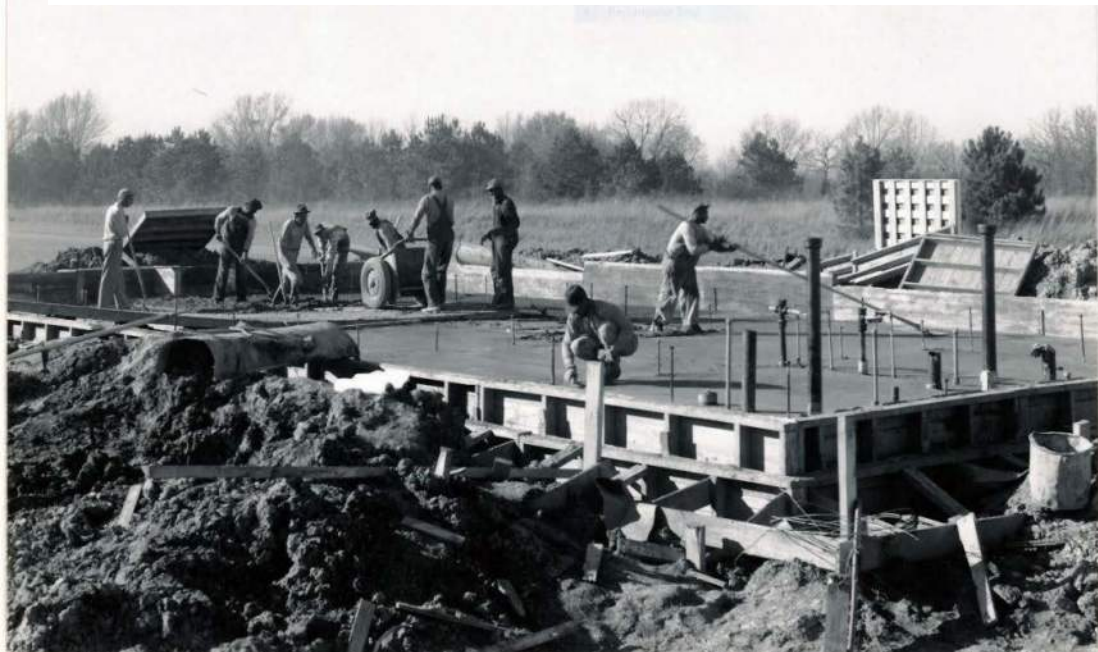
Figure 7. Information Station foundation during construction. January 16, 1951. Source: Final Construction Report, Buildings and Incidental work, Ridgeland District Headquarters, Section 3-0, Ridgeland, Miss, Contract no. I-27-27np-333, November 15, 1951. D 2623, FRC Recalled Record Collection, NATR Acc#290, Project Completion Reports-Ridgeland, Box 3, Folder 36A. Natchez Trace Parkway, Tupelo, MS.
