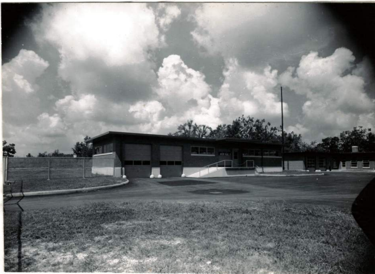
Maintenance Area - Warehouse and Material Storage Room
