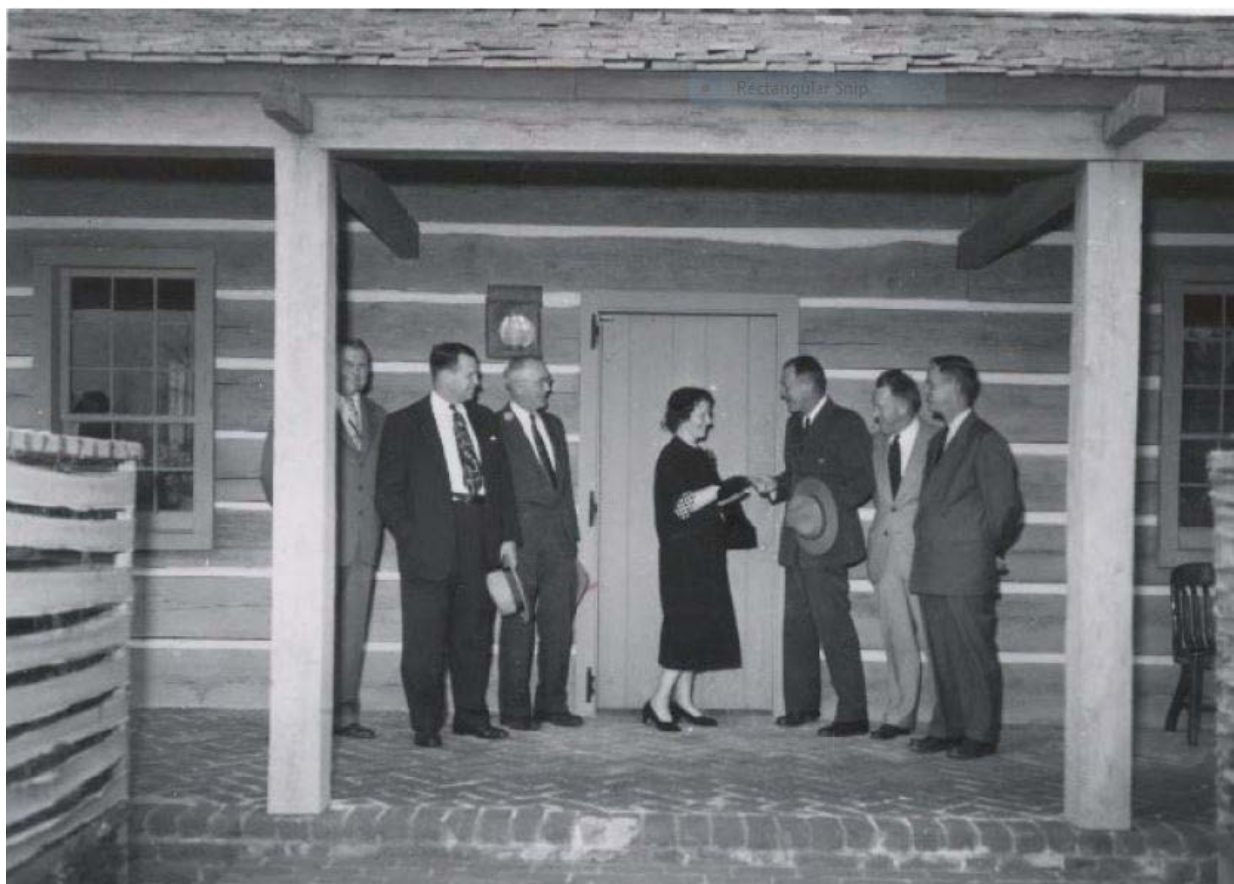
Figure 21. Exterior view from dedication in 1951 looking towards the south entrance to the Exhibit Room. Note contrast between color of logs and chinking. Note original lighting fixture. Wood rain trough and screen door are missing but hinges for screen door are present at the door jamb at left. Source: Interpretive Photographic Collection, Number 9266, Natchez Trace Parkway Archives, Tupelo, MS. 1951.
