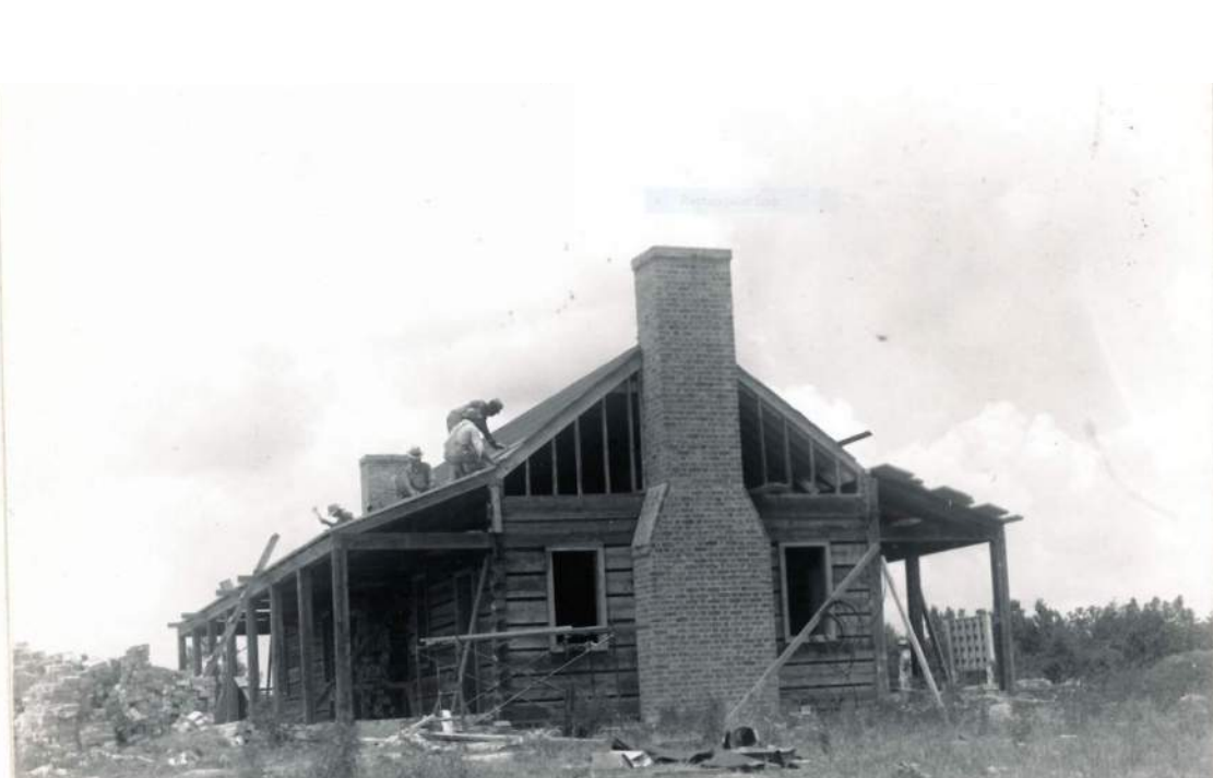
Figure 9. Information Station during construction, August 2, 1951 Source: Final Construction Report, Buildings and Incidental work, Ridgeland District Headquarters, Section 3-0, Ridgeland, Miss, Contract no. I-27-27np-333, November 15, 1951. D 2623, FRC Recalled Record Collection, NATR Acc#290, Project Completion Reports-Ridgeland, Box 3, Folder 36A. Natchez Trace Parkway, Tupelo, MS.
