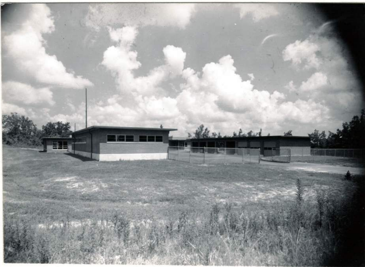
Maintenance Area -- View looking Northwest
