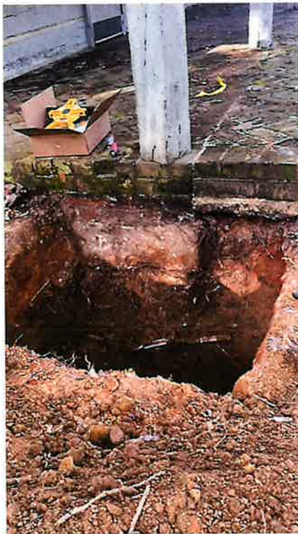
Photograph No. 6 - Grade Beam casted on top of the pile.
