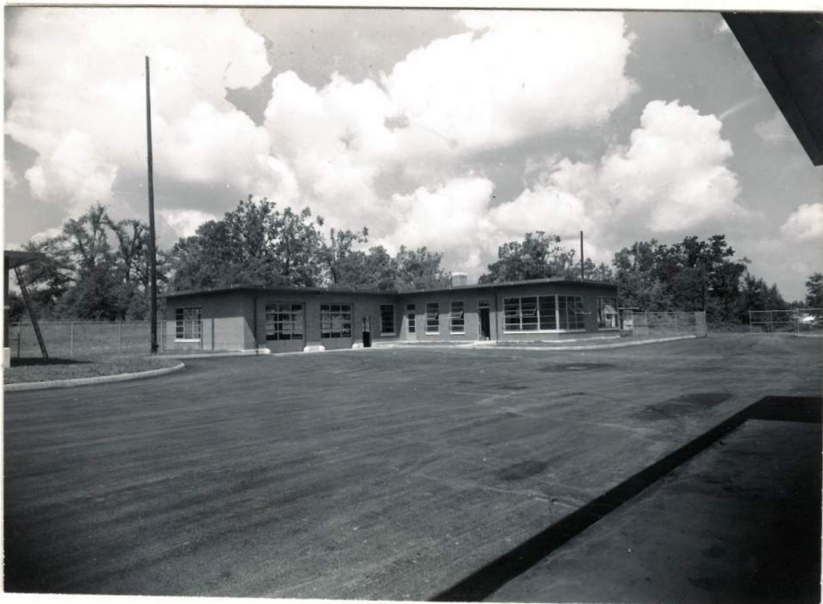
Maintenance Area - Office and Shop
