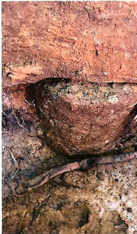
Photograph No. 3 – Exposed pile appears to be in good condition.
