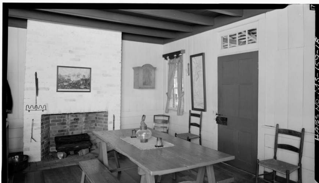
Figure 13. View of interior of Mount Locust Inn, after restoration. 1972. The Ridgeland Information Cabin has features in common including treatment of interior wall boards and wainscot, 9-over-6 window sash, and exposed beams at ceiling. Source: "Mound Plantation, Cannonsburg Vicinity, Jefferson County, Mississippi. Survey Historic American Buildings Survey, National Park Service, U.S. Department of the Interior, 1940. From Prints and Photographs Division, Library of Congress (HABS MISS, 32-Canb. V1/ http://www.loc.gov/pictures/collections/hh/item/MS0048/ ), accessed January 31, 2020.
