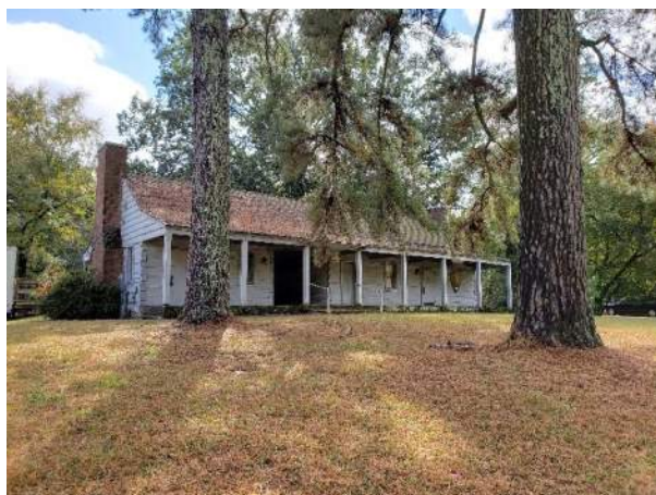
Figure 16. Overall view of cabin from the northeast.
