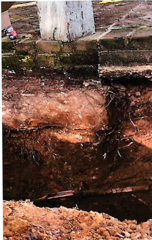
Photograph No. 7 – Grade Beam casted on top of the auger cast pile.
