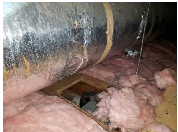
Figure 34. View of attic floor decking over Men's Toilet Room.
