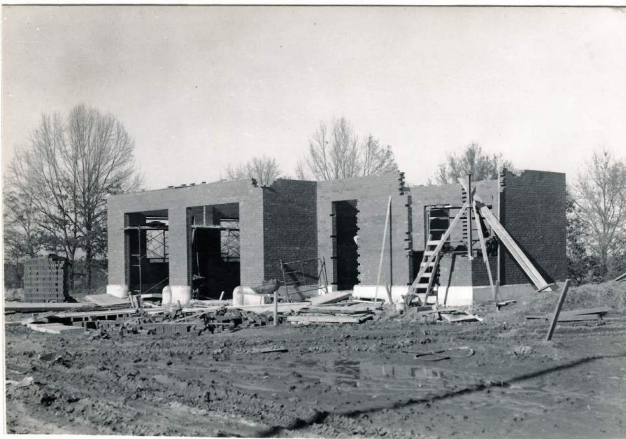
Maintenance Area - Oil and Paint Storage Building - 1/16/51
