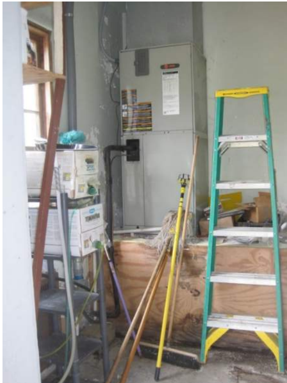
Figure 32. View of Utility Room.
