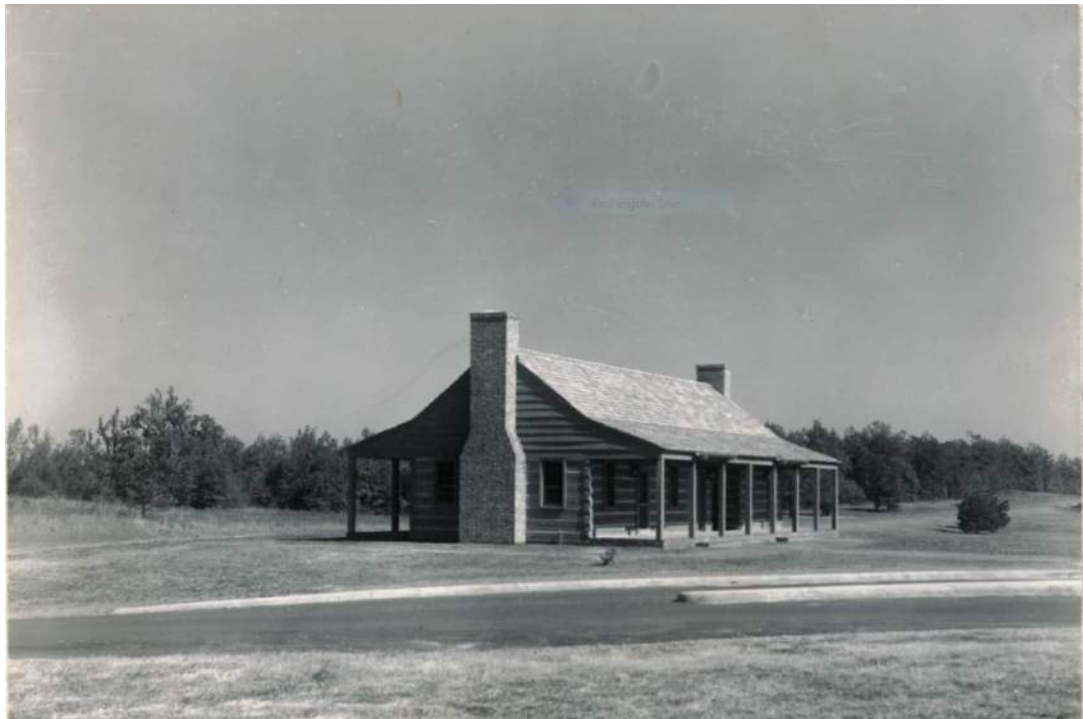
Figure 10. Information Station after completion. 1951. Source: Final Construction Report, Buildings and Incidental work, Ridgeland District Headquarters, Section 3-0, Ridgeland, Miss, Contract no. I-27-27np-333, November 15, 1951. D 2623, FRC Recalled Record Collection, NATR Acc#290, Project Completion Reports-Ridgeland, Box 3, Folder 36A. Natchez Trace Parkway, Tupelo, MS.
