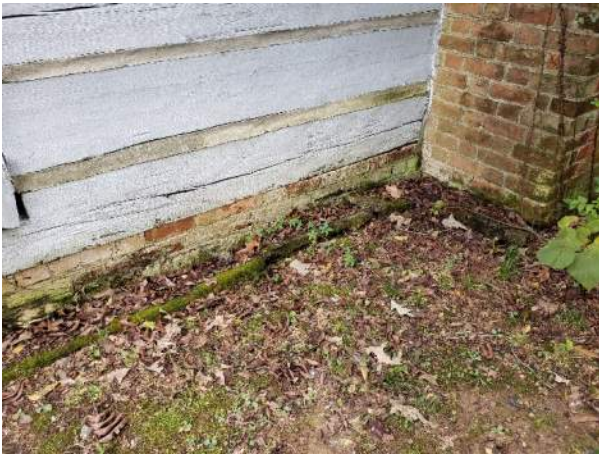
Figure 98. Existing conditions with soil grading at the foundation.
