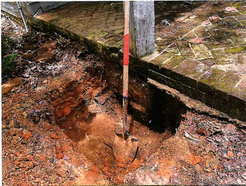
Photograph No. 1 – Test Pit#1 was excavated outside of the building adjacent to the west side at the southwest corner of the cabin.
