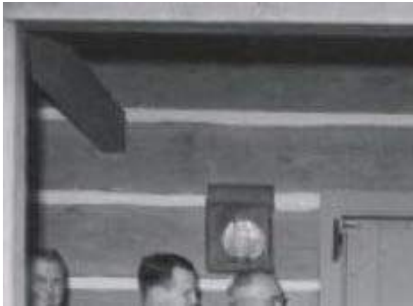
Figure 103 Detail view of original exterior light from historic image from dedication. Source: Interpretive Photographic Collection, Number 9266, Natchez Trace Parkway Archives, Tupelo, MS 1951.
