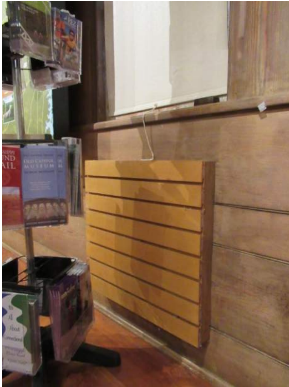
Figure 27. Wood covers have been placed over the original electric heaters.
