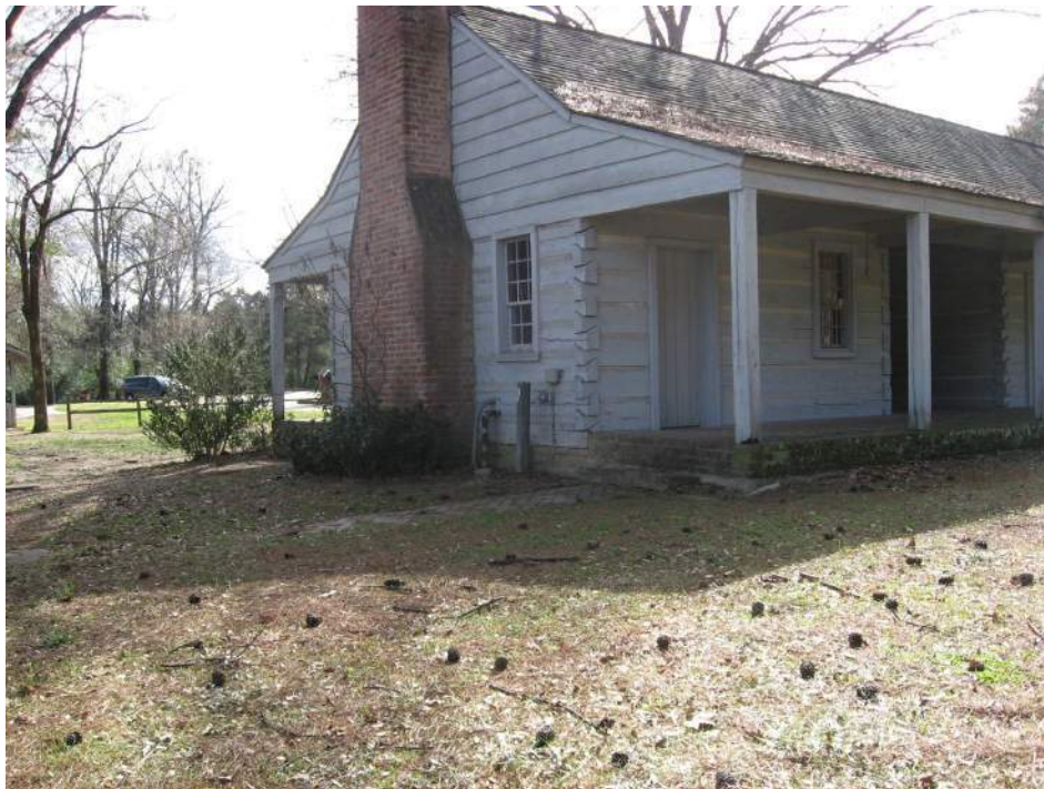
Photo 10: View of the northeast corner.
