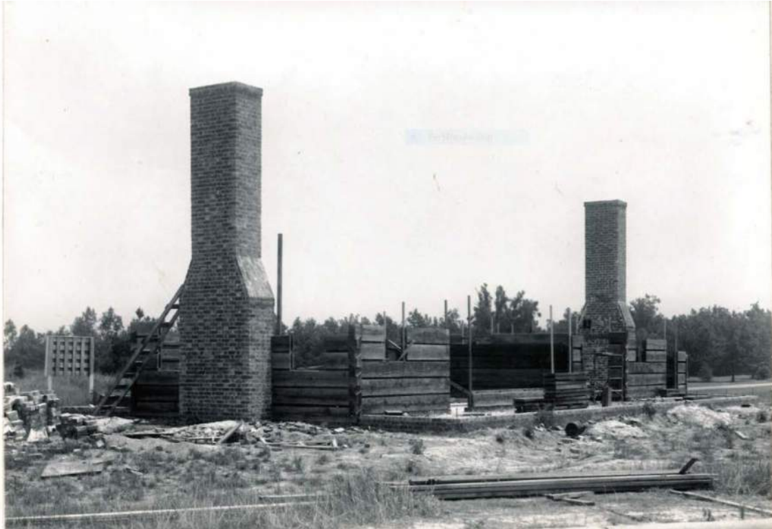
Figure 8. Information Station during construction, June 21, 1951. Source: Final Construction Report, Buildings and Incidental work, Ridgeland District Headquarters, Section 3-0, Ridgeland, Miss, Contract no. I-27-27np-333, November 15, 1951. D 2623, FRC Recalled Record Collection, NATR Acc#290, Project Completion Reports-Ridgeland, Box 3, Folder 36A. Natchez Trace Parkway, Tupelo, MS.
