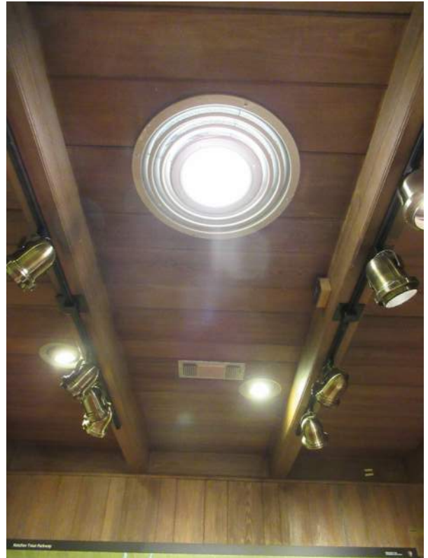
Figure 29. View of ceiling showing original lighting fixture and air diffuser. The brass track lighting was added at a later date.
