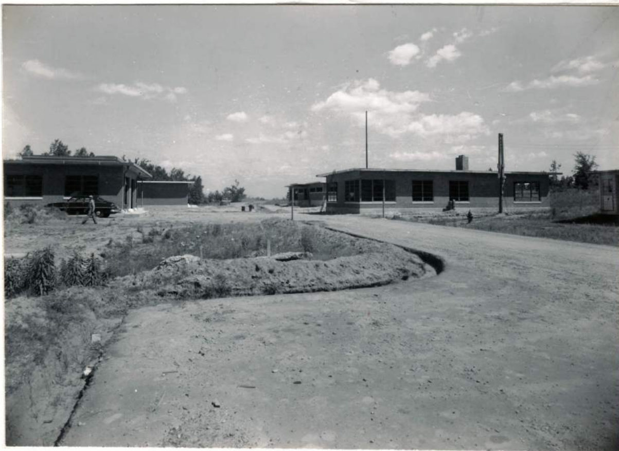
Maintenance Area -- View looking Southeast, 5/23/51
