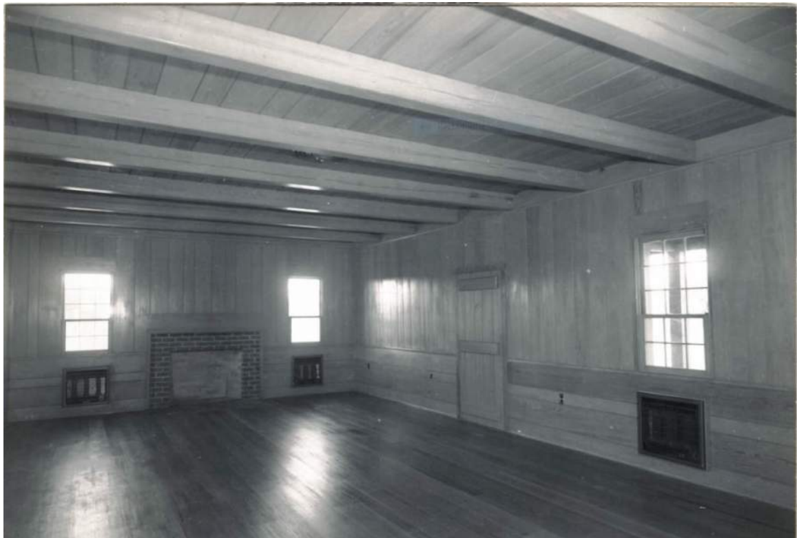
Figure 11. Interior of Exhibit Room, Information Station. 1951 Source: Final Construction Report, Buildings and Incidental work, Ridgeland District Headquarters, Section 3-0, Ridgeland, Miss, Contract no. I-27-27np-333, November 15, 1951. D 2623, FRC Recalled Record Collection, NATR Acc#290, Project Completion Reports-Ridgeland, Box 3, Folder 36A. Natchez Trace Parkway, Tupelo, MS.
