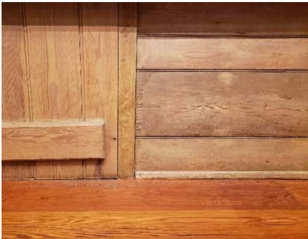
Figure 25. Detail view of interior horizontal boards at wainscot, board and batten doors, and refinished floor.
