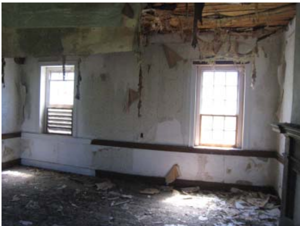
Figure 153. Southeast oblique of West Bedroom (Room 201).
