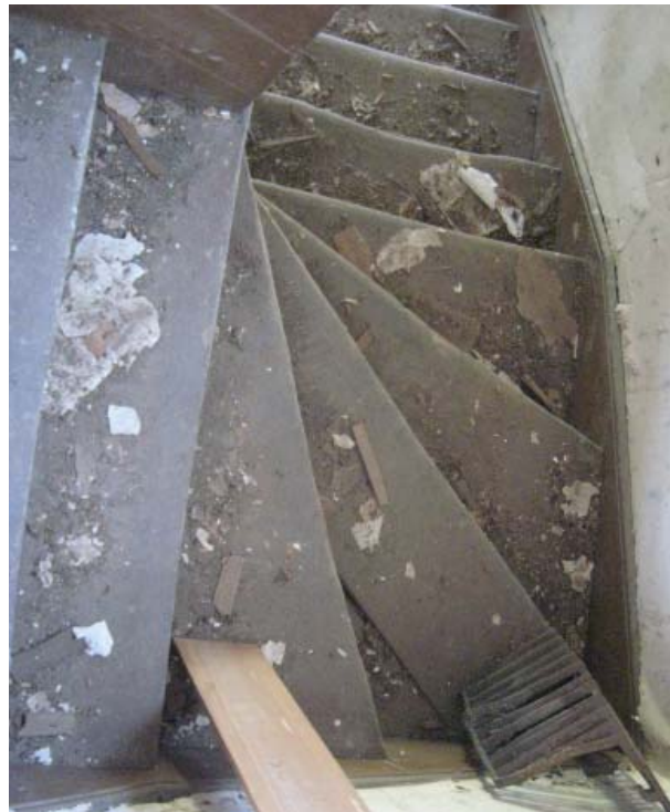
Figure 160. Staircase winders.
