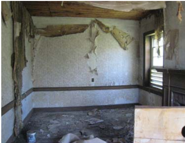
Figure 162. Northwest oblique of East Bedroom (Room 202).
