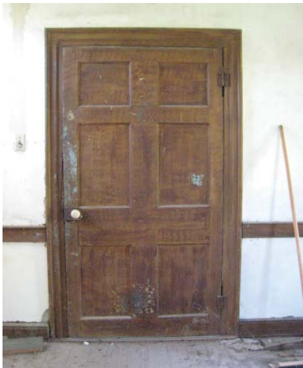
Figure 147. Faux wood graining of door to Hall (Room 101).
