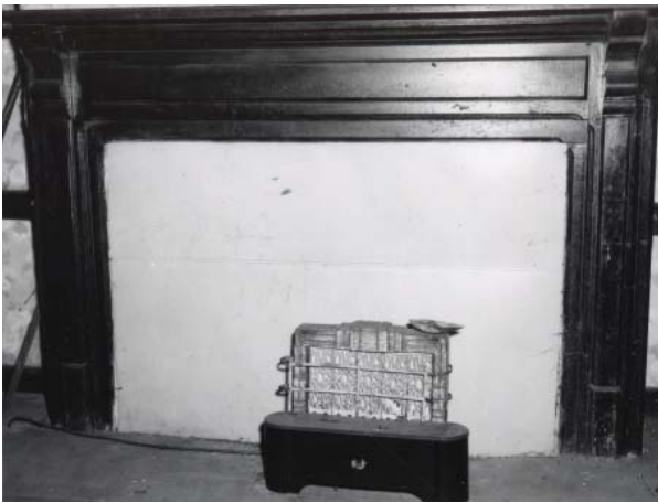
Figure 55. Mantelpiece in first-floor east room (Room 102). (Trout, 1969, NATR collection # 10912)
