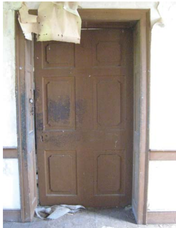
Figure 155. Doorway to East Bedroom (Room 202).
