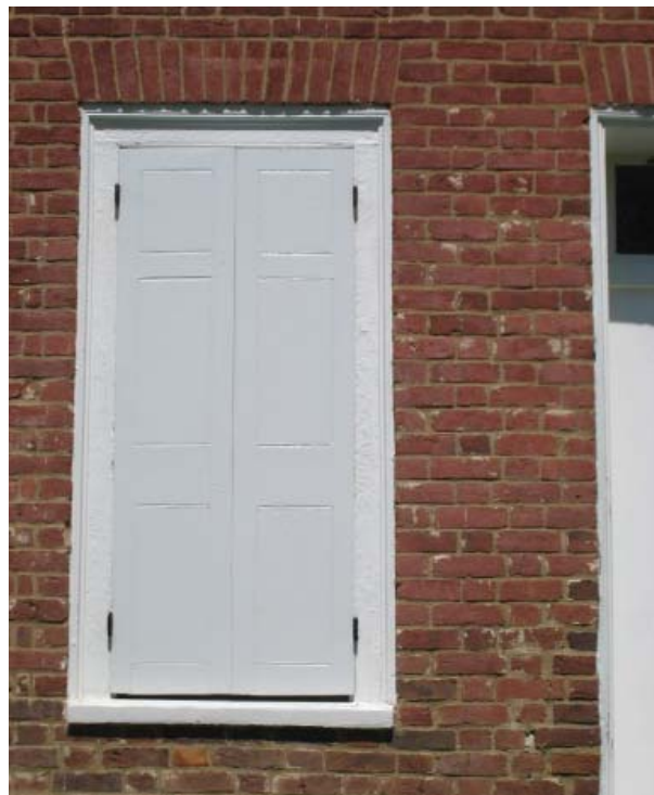
Figure 101. Typical first-floor reproduction window shutters.
