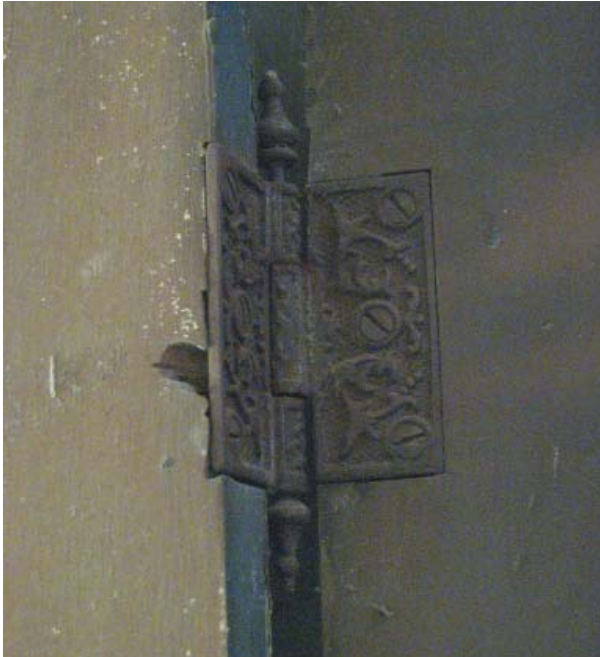
Figure 136. Embossed hinge of door on stairway to second floor.
