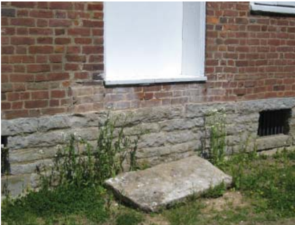
Figure 96. Brick walls atop foundation of chiseled blocks of grey limestone.
