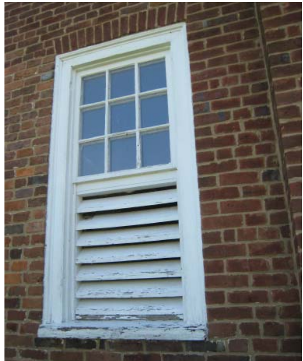
Figure 166. Added window louvers for passive ventilation.
