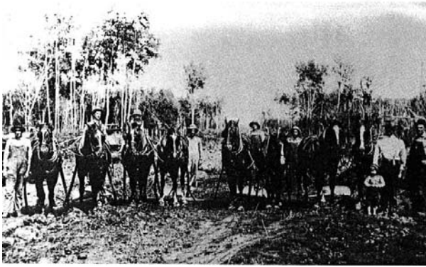
Figure 42. Road Building. (schultzonline.org)
