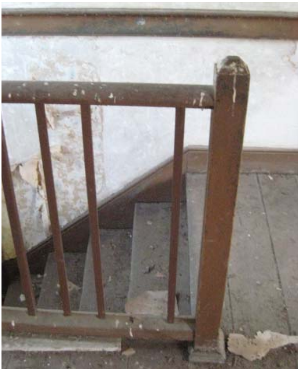
Figure 159. Second-floor staircase newel and balustrade.
