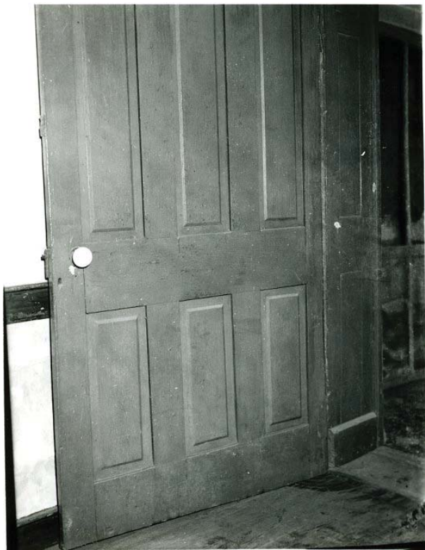
Figure 59. Rear door of Room 102 leading to northeast rear shed porch. The screen door into the annex can be seen. (Trout, stapled in 1969 report, NATR collection)
