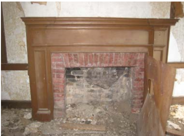
Figure 164. Fireplace of East Bedroom (Room 202).
