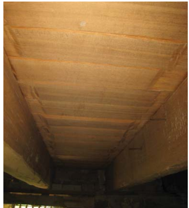
Figure 97. Hewn joists and gauged flooring.
