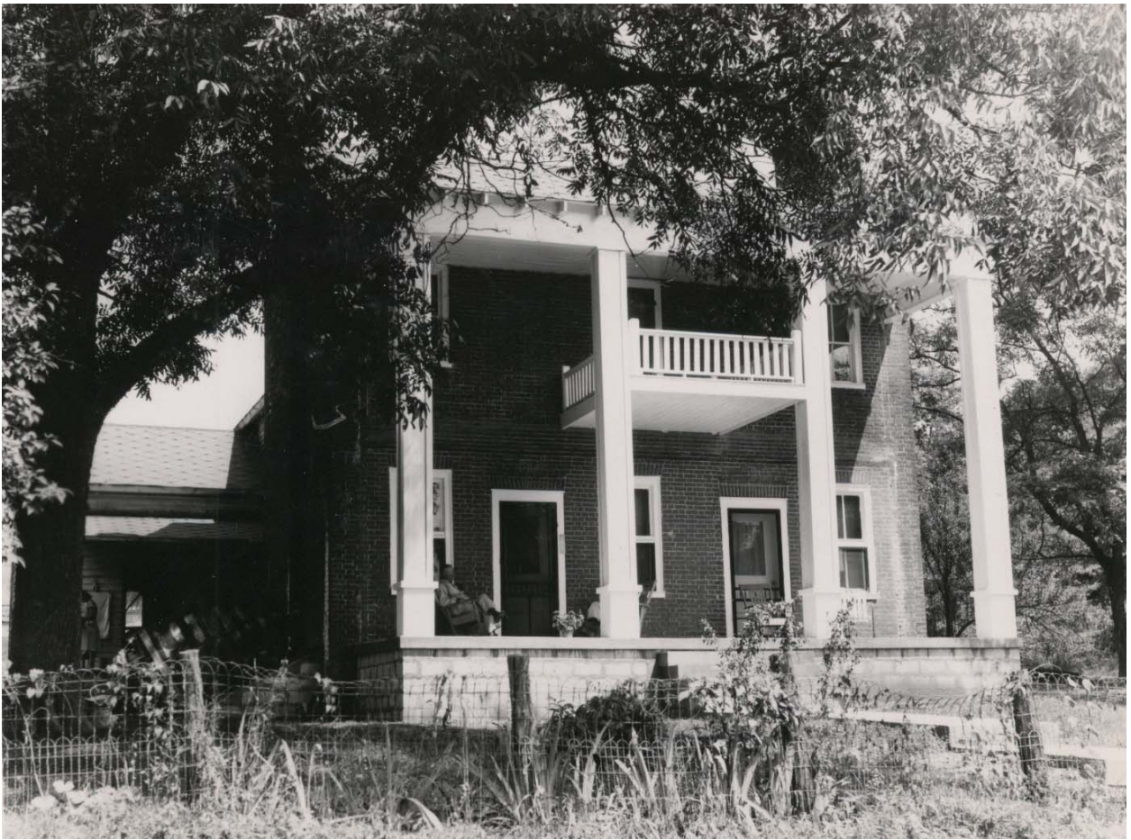
Figure 51. Full-height porch built in 1947-48. (Cotter, 1948, NATR collection #6670)
