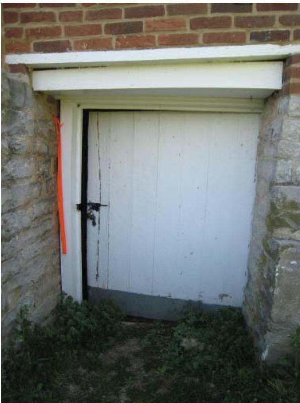
Figure 113. Exterior view of basement doorway.
