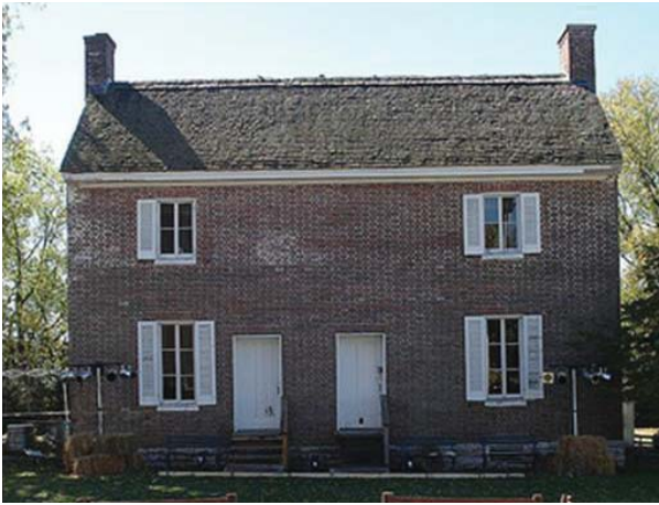
Figure 36. House at Two Rivers Mansion, ca. 1802, Donelson, Tennessee. (nashville.gov/parks/historic)
