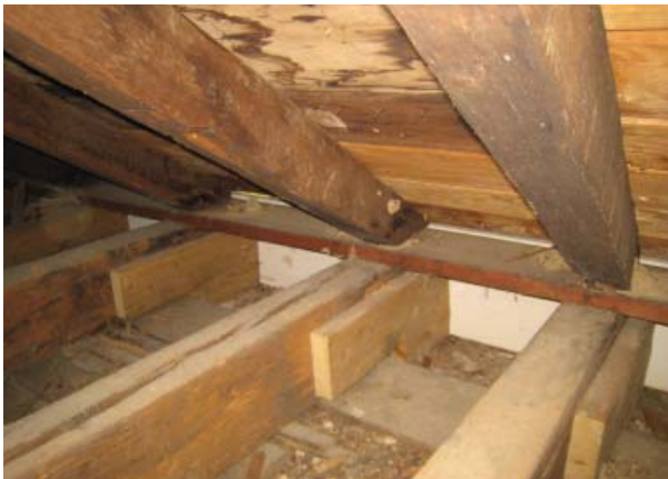
Figure 99. Hewn joists and sash-sawn rafters.
