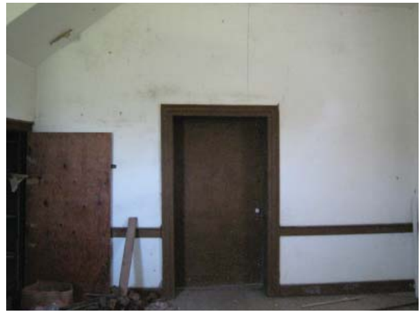
Figure 134. Hall side of doorway to Parlor.
