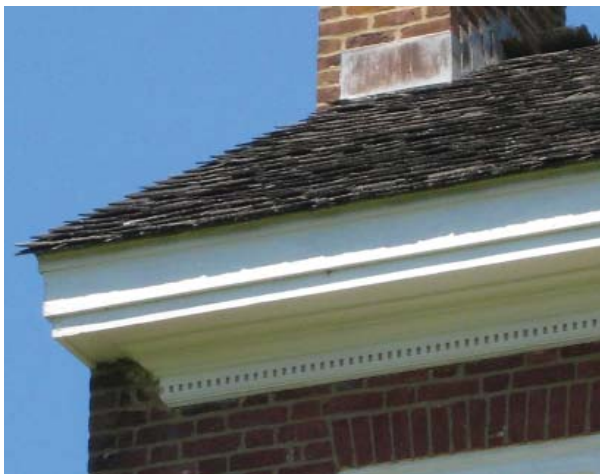
Figure 71. Wood shingle roof and reproduction dentil cornice. (2010 photograph)
