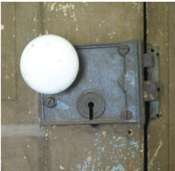
Figure 137. Rim lock of door on stairway to second floor.
