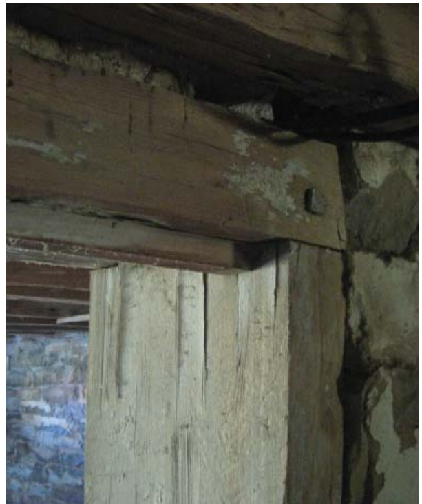
Figure 122. Doveled and tenon framing of interior doorway.
