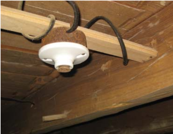
Figure 102. Typical porcelain light bulb socket of 1977-78.
