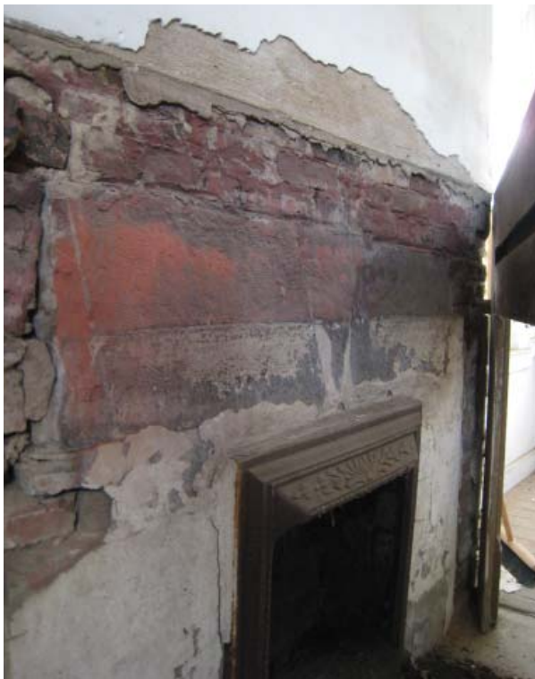
Figure 138. Faux-dressed stonework behind replacement mantle of Room 101.
