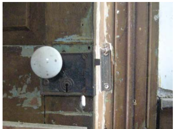
Figure 110. Replacement rim lock - secondary entrance door.
