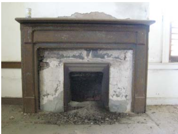
Figure 139. Fireplace of Room 101.
