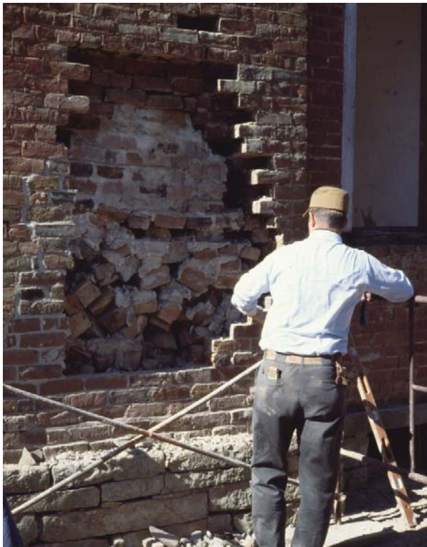
Figure 70. Brick repair of east chimney, 11/1977. (color transparency, NATR collection)
