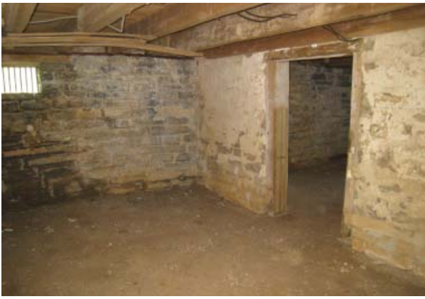
Figure 127. Southwest oblique of Room 002.
