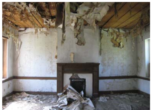
Figure 157. Fireplace of West Bedroom (Room 201).
