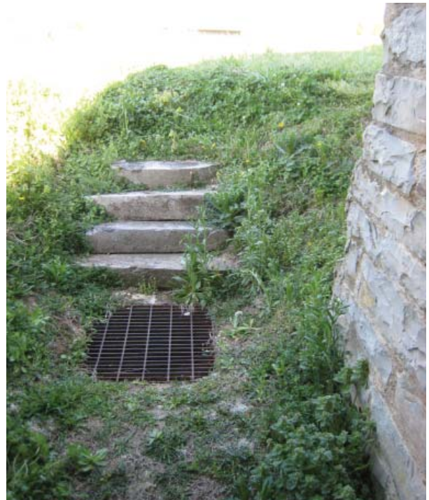
Figure 91. Stone steps leading from Basement. Modern catch basin is at the base of the steps.
