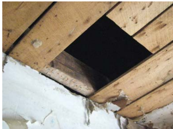
Figure 161. Ceiling access opening of West Bedroom (Room 201).
