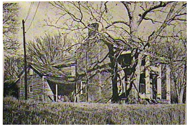
Figure 72. 1976 photograph shows power pole. Underground connection was made to the basement in 1977. (NATR collection)
