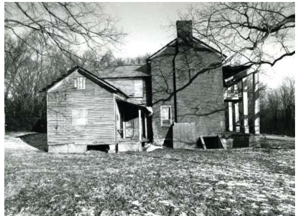
Figure 64. West elevation in 1977 before front porch and rear sections were removed. (NATR collection)
