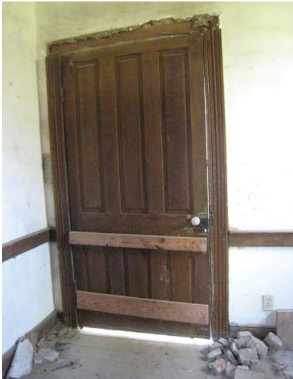
Figure 108. Interior view of the original secondary entrance doorway, at the rear or north elevation, Parlor (Room 102). The door dates to c. 1840-50 and the interior casing to the early twentieth century.
