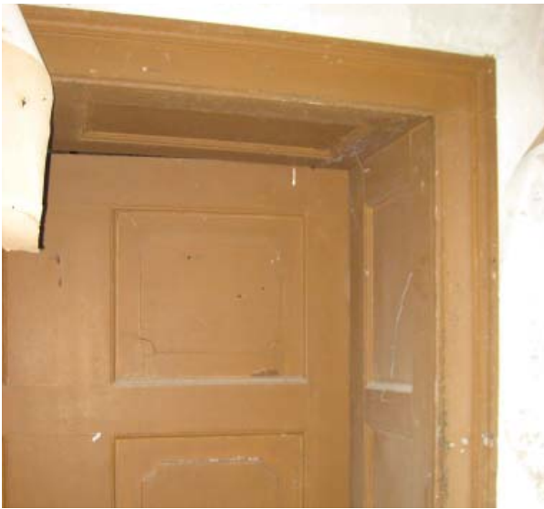
Figure 156. Paneled jamb of doorway between Room 201 and Room 202.
