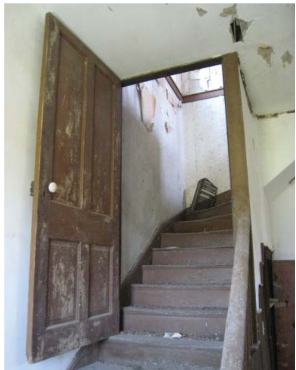
Figure 135. Early-twentieth century stairway enclosure in Room 101.
