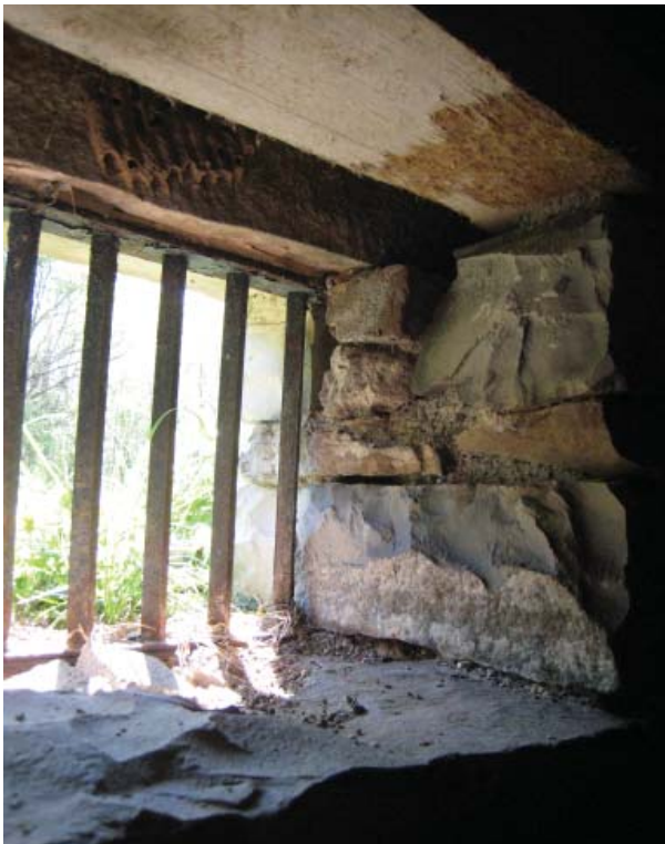
Figure 130. Vent in foundation wall.
