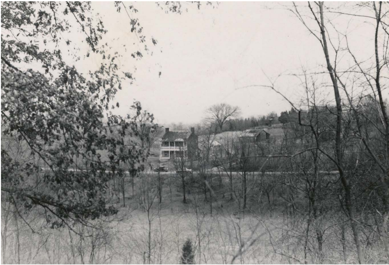
Figure 49. View of the Gordon House in 1945 looking northwest from the ridge between the Duck River and Fattybread Branch and showing Highway 50 in front of the house. (Phelps, 1945, NATR collection #6084)
