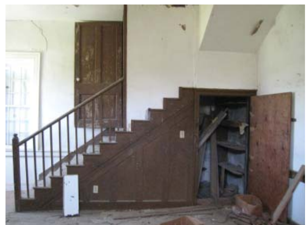
Figure 140. Staircase of Hall (Room 101).
