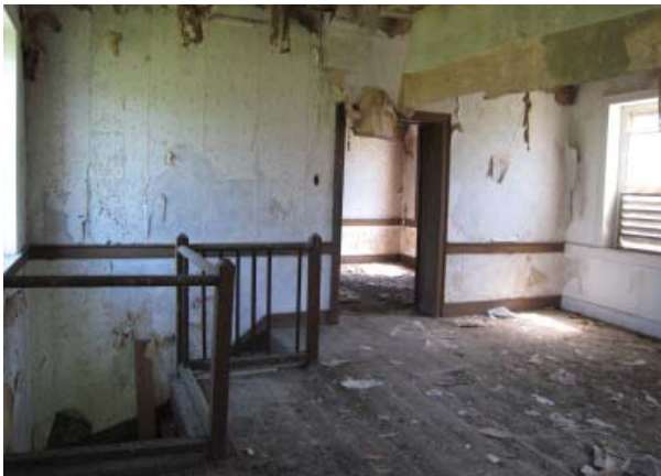
Figure 158. Staircase at West Bedroom (Room 201).
