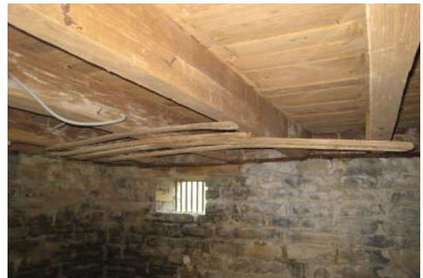
Figure 128. Split wood hangers nailed to bottom of joists.
