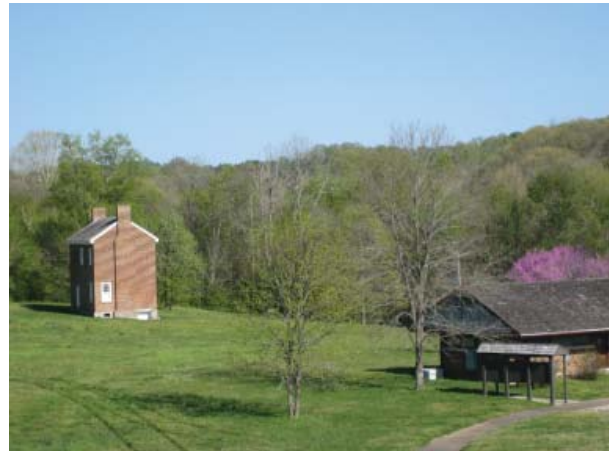
Figure 85. Gordon House and comfort station/picnic shelter.
