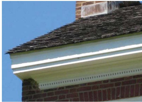
Figure 107. Roof cornice of north and south elevations.
