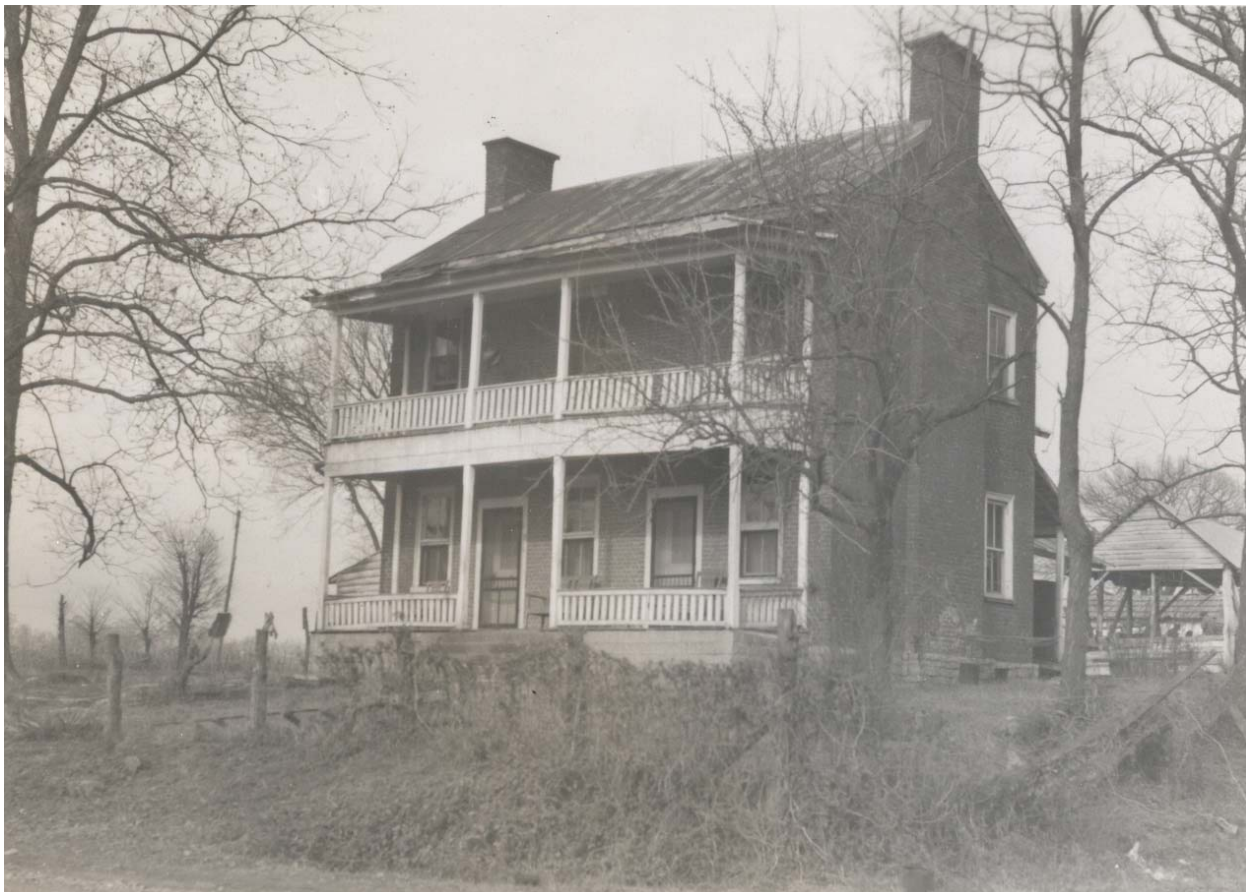
Figure 46. 1944 photograph shows the double-gallery porch built ca. 1907 and replacement two-over-two-light sash.. (Phelps, 1944, NATR collection #5485)
