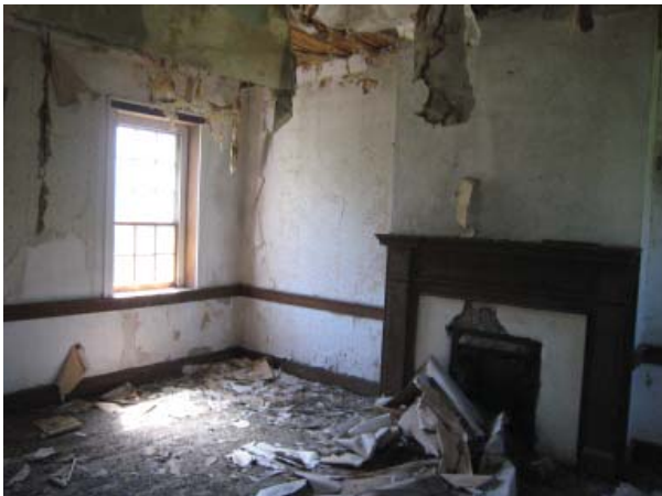
Figure 154. Southwest oblique of West Bedroom (Room 201).
