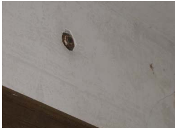
Figure 144. Bolt and nut on the upper south wall of the Hall, probably for securing the upper section of the double gallery.
