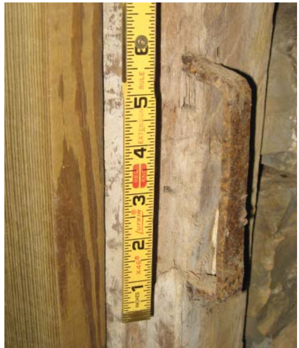
Figure 123. Wrought-iron staple on north jamb of doorway between Room 001 and Room 002.
