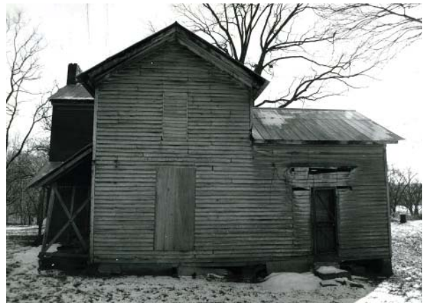
Figure 65. North elevation of rear ell before removal in 1977. (NATR collection)
