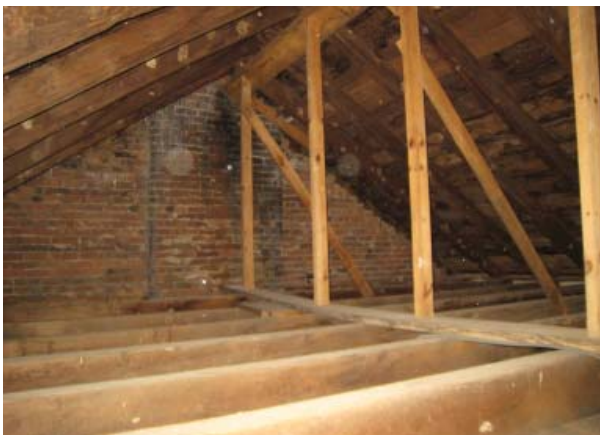
Figure 100. Supplemental support of rafters.
