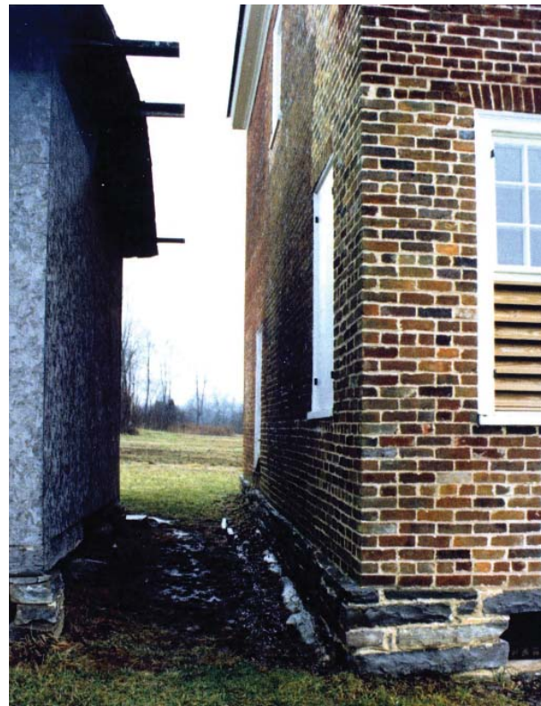
Figure 75. 1991 view showing braced frame structure, with protective roof and sidewalls, at the rear of the house. (HSAR 1992)
