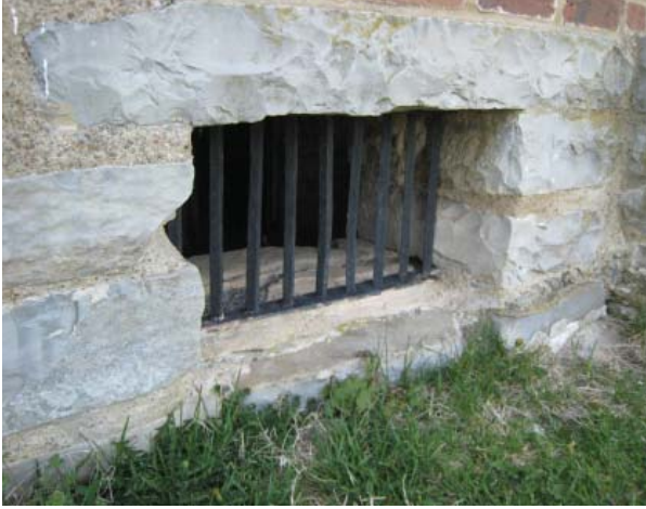
Figure 95. Typical foundation vent.
