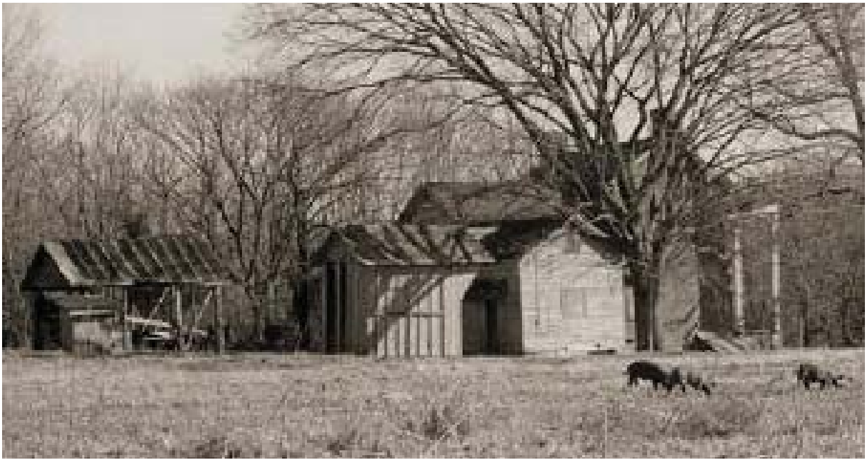
Figure 62. 1976 photograph showing front porch, complex of rear additions, woodshed, and pasture. (gordonhouse.50megs.com)
