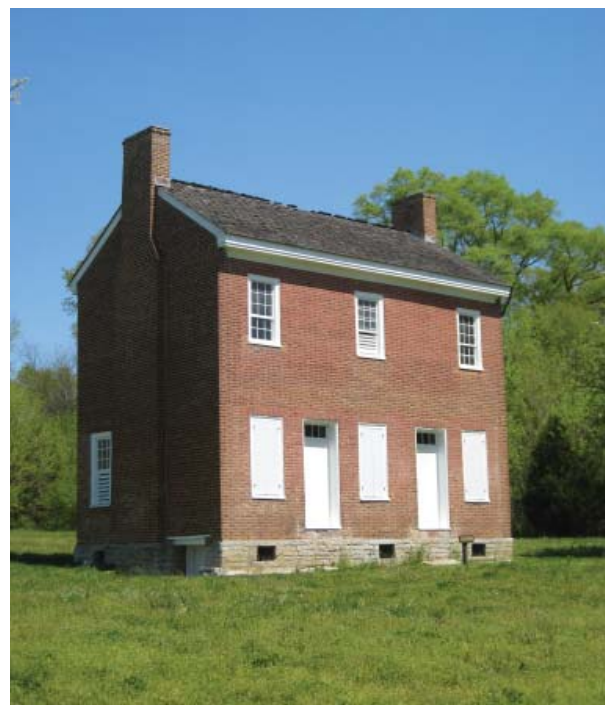
Figure 89. Flemish bond and five-bay design of south facade.
