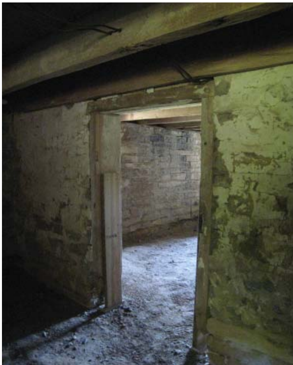
Figure 121. Connecting doorway as viewed from Room 002.
