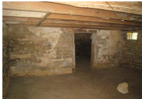
Figure 120. Southeast oblique of Room 001.
