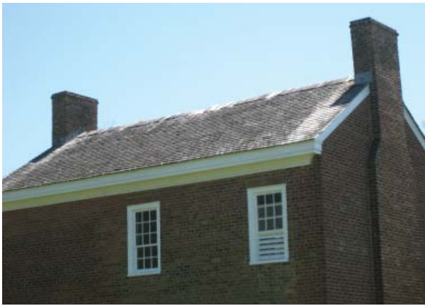
Figure 105. Split shingle roofing.
