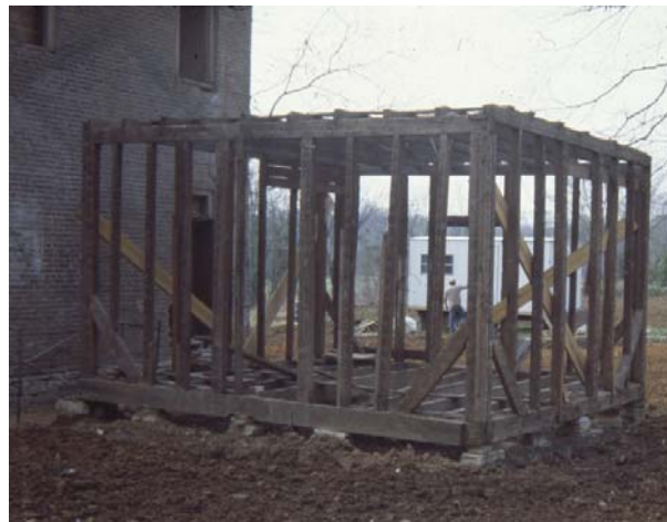
Figure 66. Braced frame structure found within two-story ell, 11/1977. Possible ghostmark of a front-gabled roof is visible on the rear wall of the brick house. (color transparency, NATR collection)
