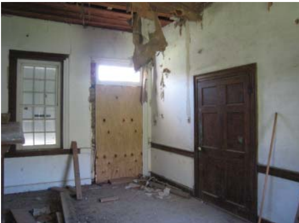
Figure 145. Southwest oblique of Parlor (Room 102).
