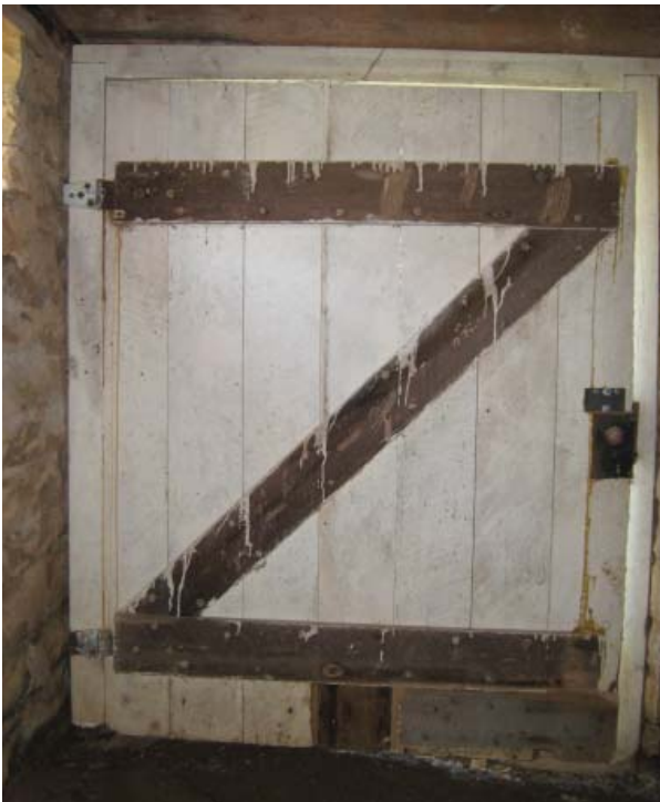
Figure 112. Interior view of basement doorway.
