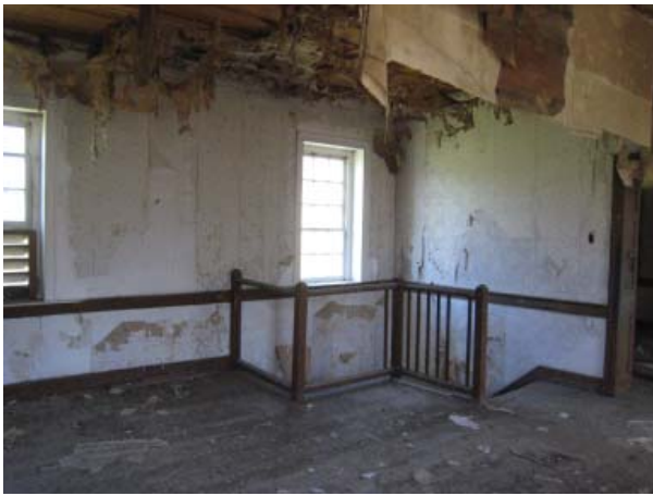
Figure 152. Northeast oblique of West Bedroom (Room 201).
