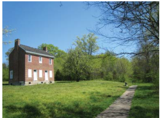
Figure 86. Walkway along old State Highway 50 road bed.
