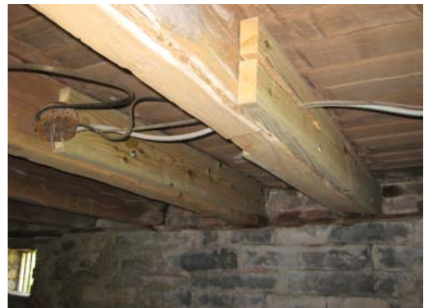
Figure 98. Sistered joists on south wall of Room 001.
