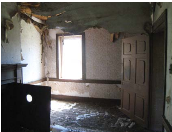
Figure 163. Southeast oblique of East Bedroom (Room 202).
