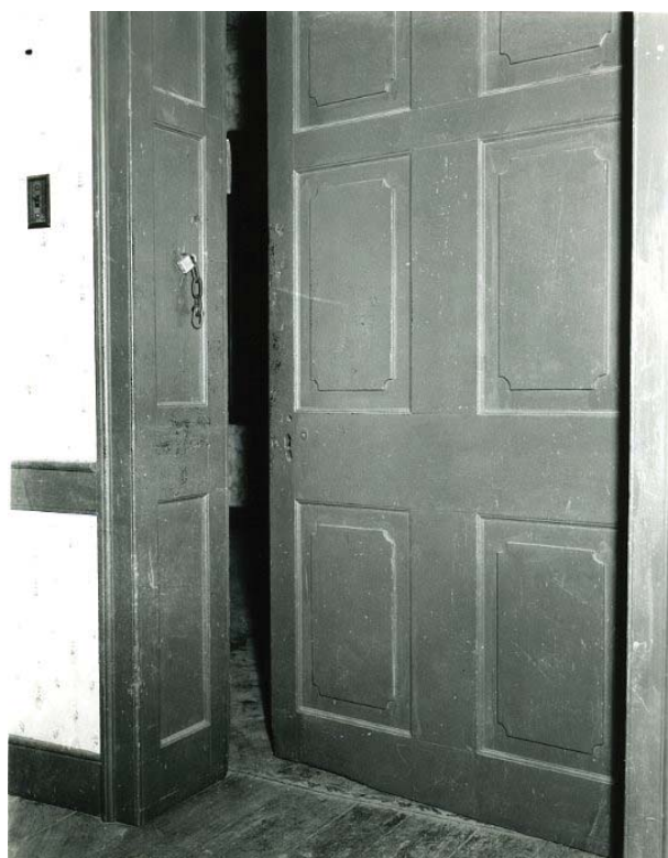
Figure 61. Door leading from Room 201 to Room 202. (Trout, stapled in 1969 report, NATR collection)
