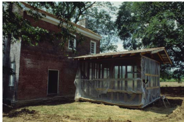
Figure 67. Temporary roof during installation on braced frame structure, 8/1978. (color transparency, NATR collection)
