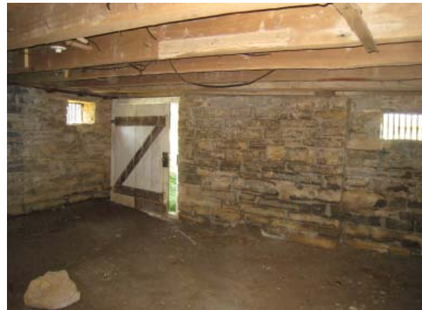
Figure 119. Southwest oblique of Room 001.
