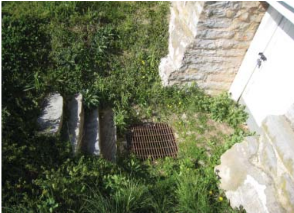
Figure 106. Catch basin at entrance to Basement.
