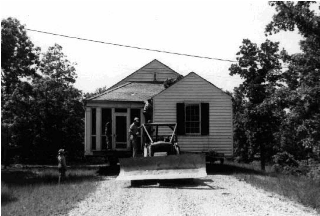
Moving the custodian's residence, 1960
