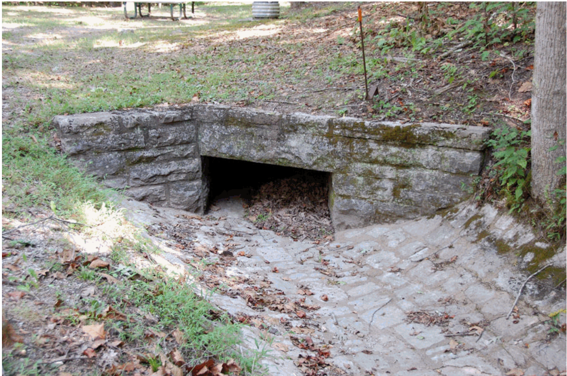
Old Spring culvert, south of picnic loop. 2008.
