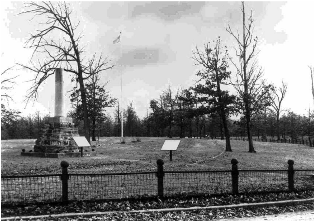
War Department improvements circa 1934. Note the interpretive tablets, the iron fence with cannonballs, and the curbing in the foreground .
