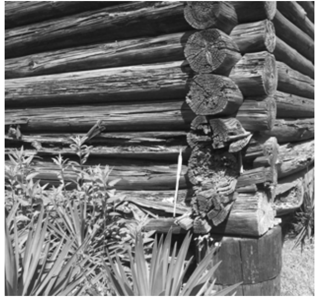
FIGURE 25. View of deteriorated logs around building's north corner.
