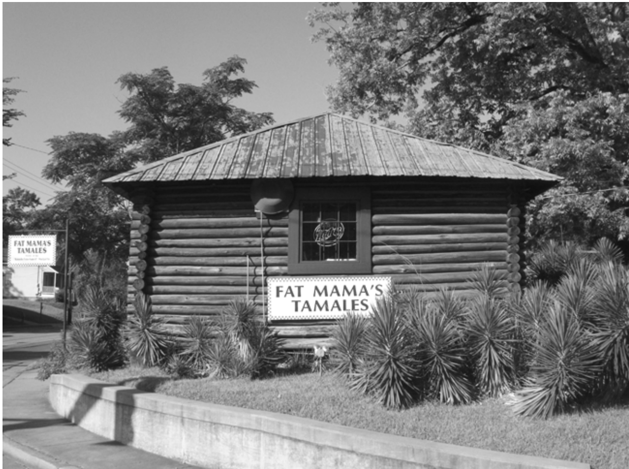
FIGURE 27. View of northeast end of building.
