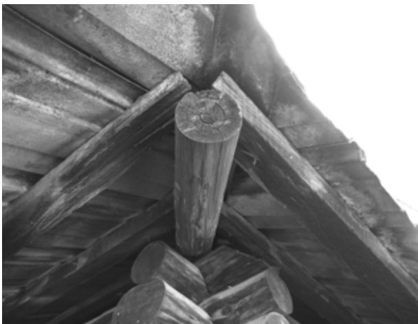
FIGURE 33. View of southwest corner of roof.
