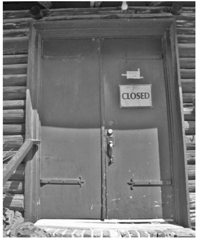
FIGURE 39. View of front doors.
