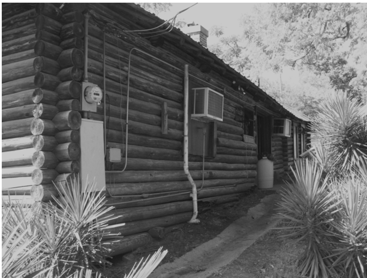
FIGURE 23. View south of rear of building.
