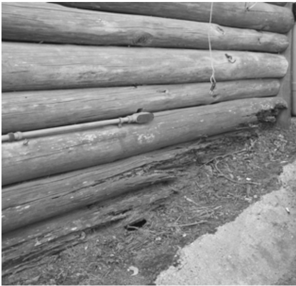
FIGURE 26. View of partially buried, badly deteriorated logs near back door. The sill log is
