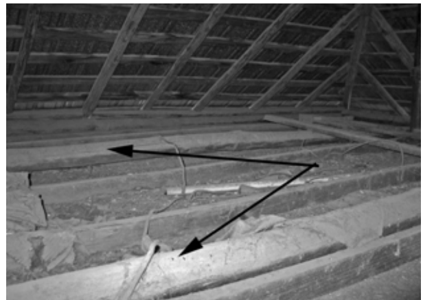
FIGURE 30. View of tie logs (indicated by arrows) and ceiling joists at southern end of building.
