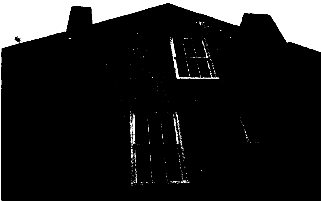
29-A Main House - Gap between left window frame and wall on west elevation. Right window frame and sash unpainted.
