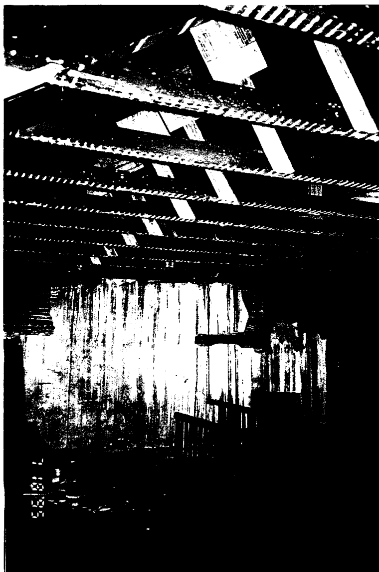
40-A Main House - Missing third-floor plaster.
