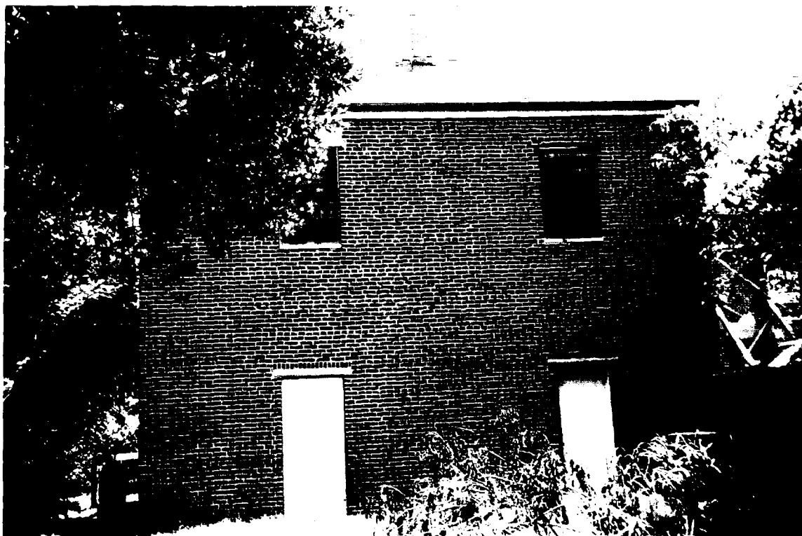
66-A Dependency - Caulk gaps at window frames on north facade.
