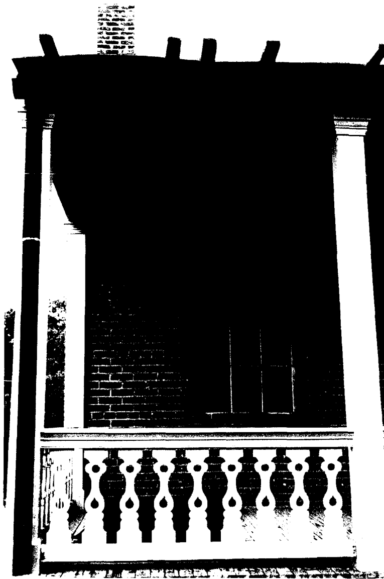
30-A Main House - Second-floor window frames on south elevation need to be caulked and painted.
