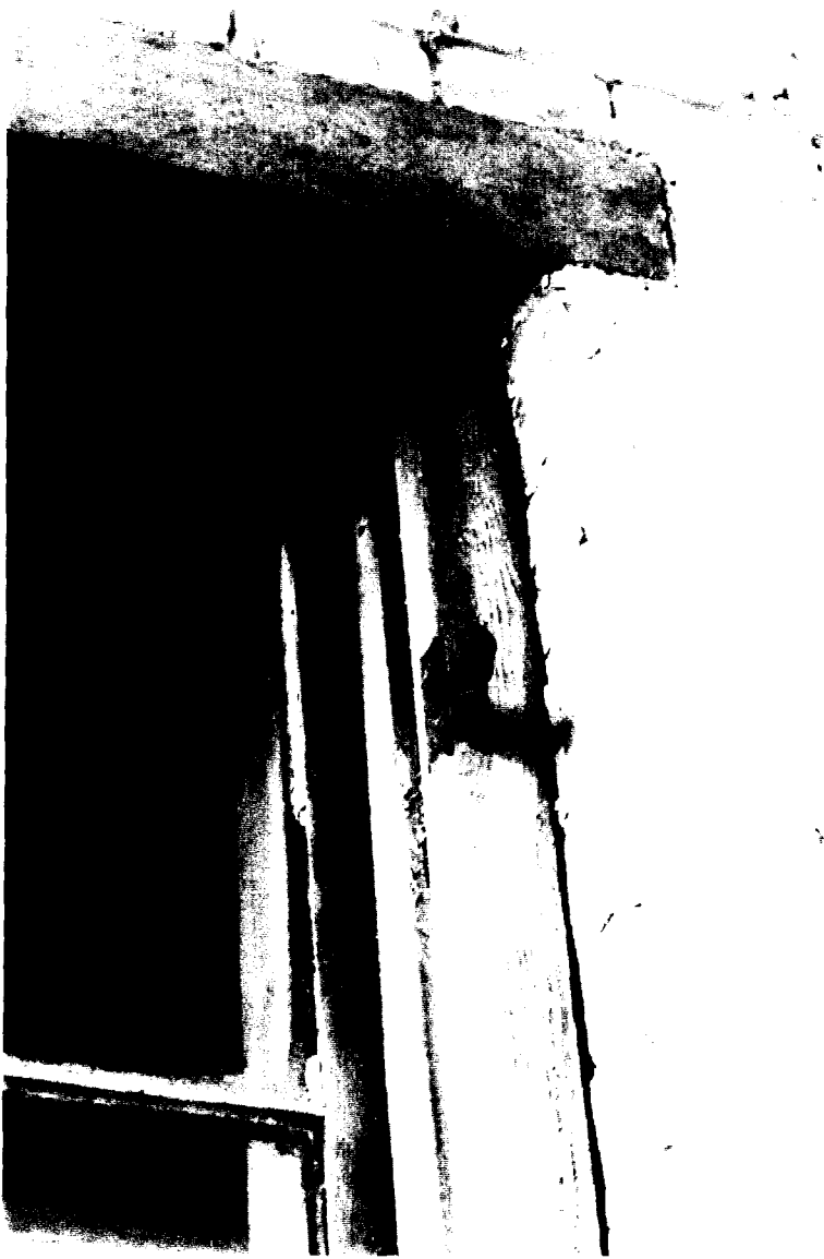
66-A Dependency - Caulk gaps at window frames on north facade.
