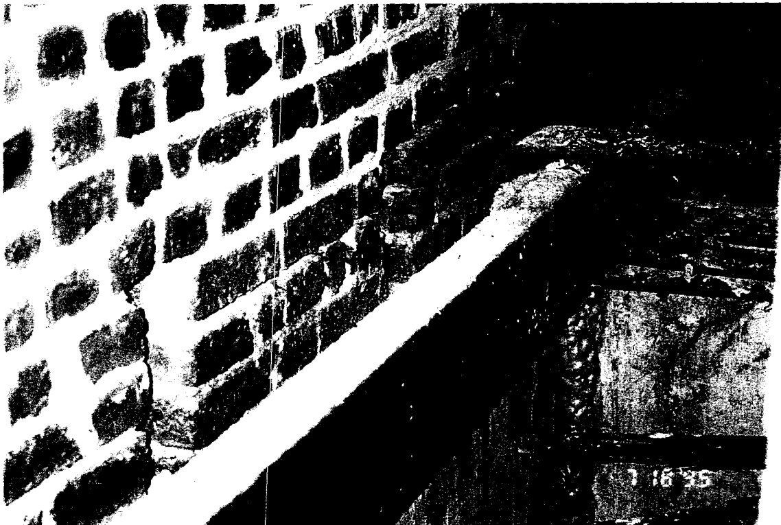
22-A Main House - Gap in wall injected with foam at southeast corner of second floor.
