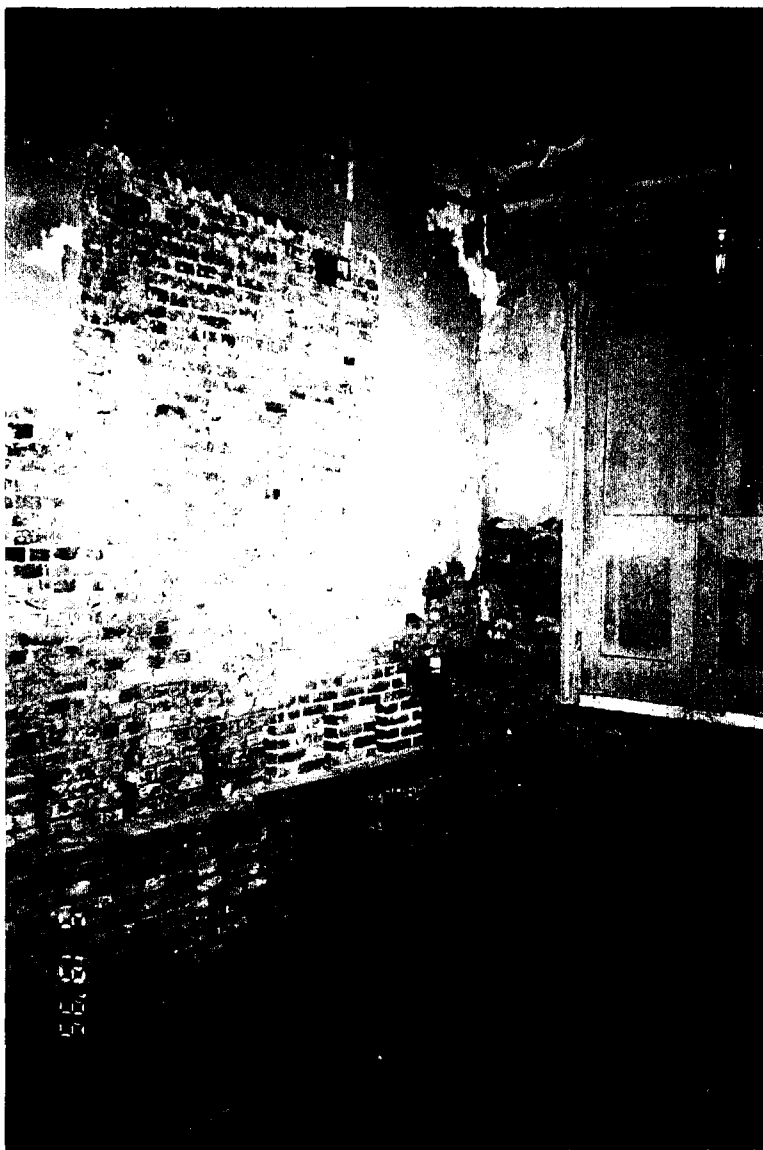
32-A Main House - Missing floor joists and floor from first floor. Missing plaster from walls.
