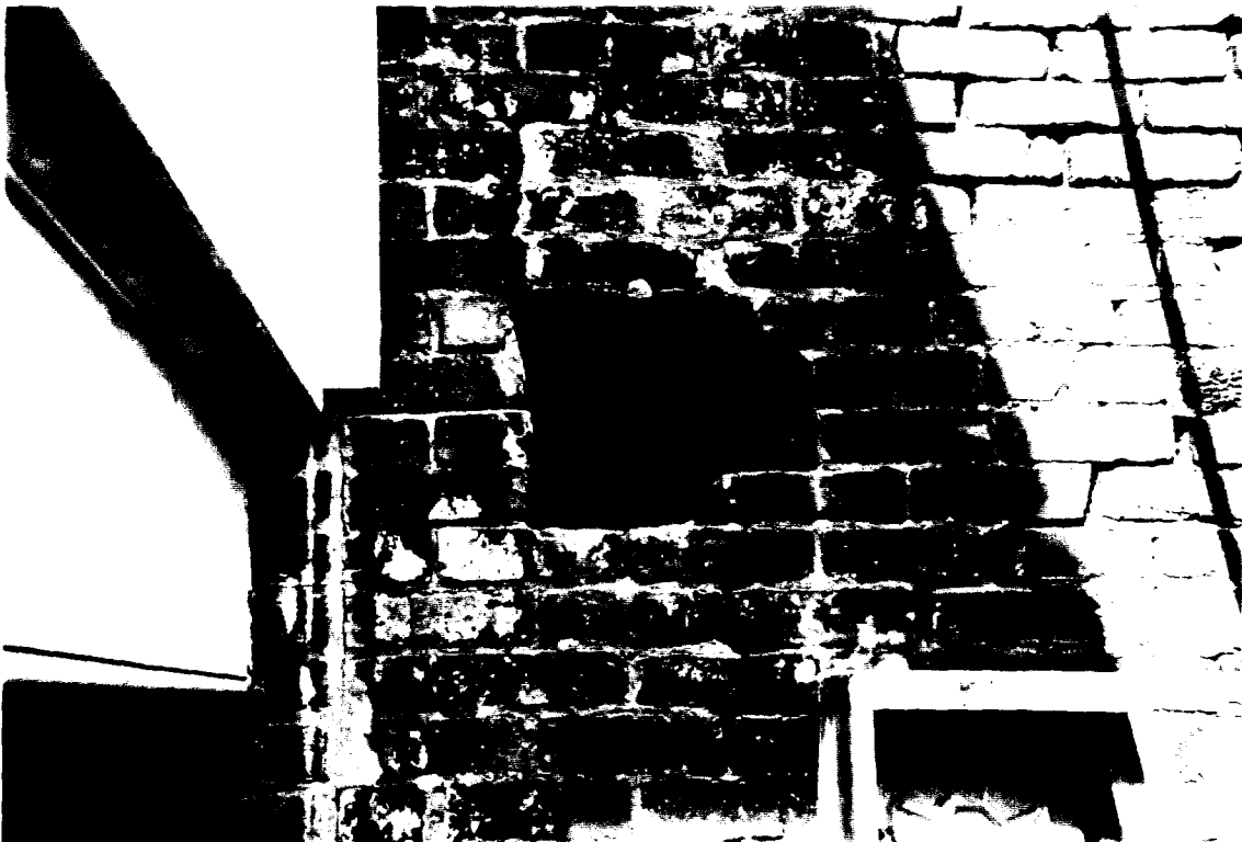
60-S Area of probe made into the south elevation of the McCallum House and William Johnson House.
