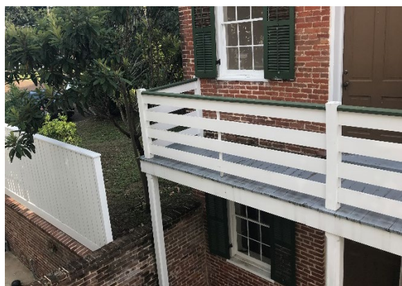
FIGURE 3-9. Photograph taken in 2019 of the north side of the 1897 kitchen dependency. Suzanne Turner Landscape Architects.
