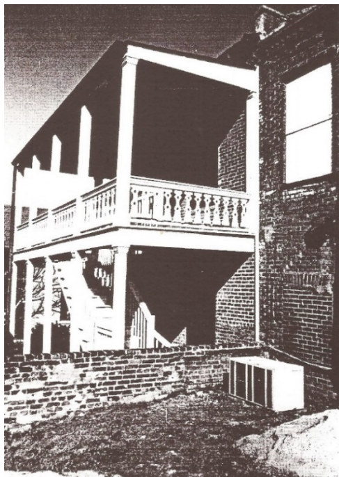
FIGURE 2-31. Photograph taken in the 1990s, showing a freestanding wall between the Johnson and McCallum courtyards. Atkinson.
