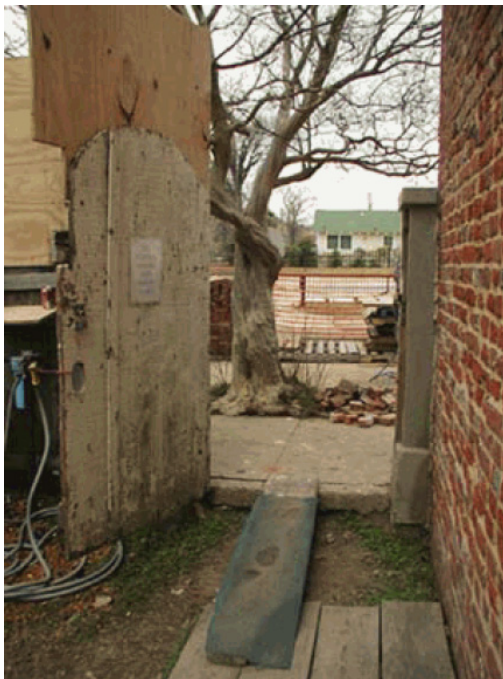
FIGURE 2-39. Arch-top, vertical plank entrance gate at the William Johnson House in 2003. Jaeger Associates.
