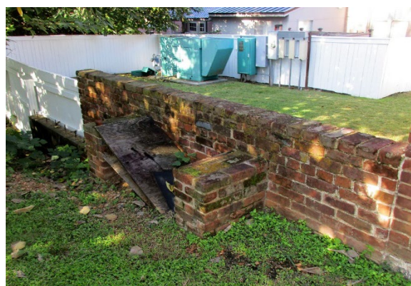
FIGURE 3-11. Photograph taken in 2019 of the combined retaining and free-standing brick wall and its concrete extension. Suzanne Turner Landscape Architects.
