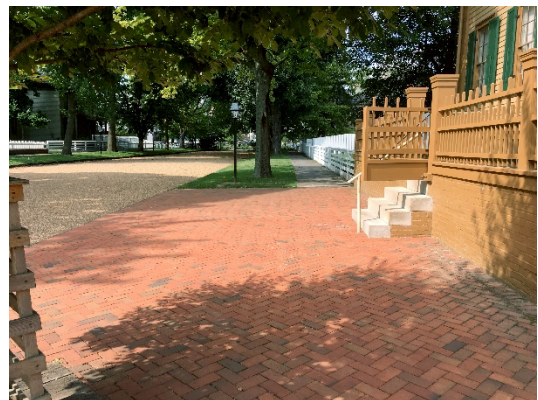
FIGURE 5-1. Brick walkway at Lincoln Home Historic Site. The walkway was designed and installed to meet ABAAS standards. Christina Osborn.
