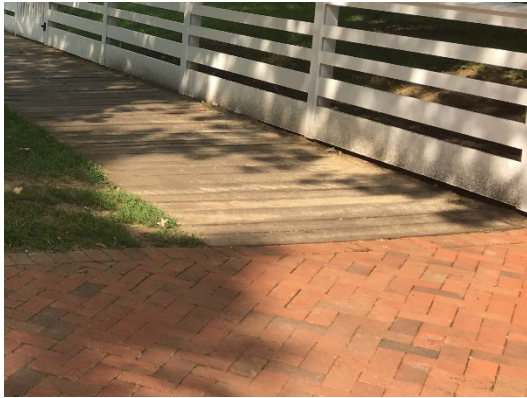
FIGURE 5-2. Wood boardwalk adjoining brick walkway at Lincoln Home Historic Site. The two materials were joined to meet ABAAS standards. Christina Osborn.
