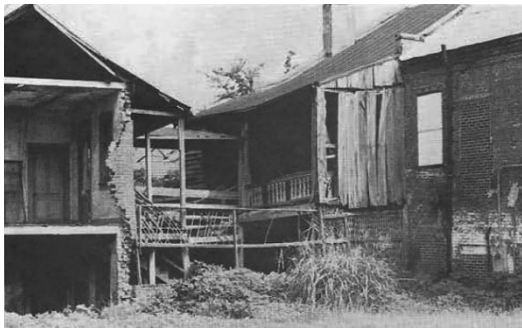
FIGURE 2-12. Photograph taken of the rear gallery of the William Johnson House in the 1970s before restoration. The crisscross lattice is used here as a privacy screen. Padgett.
