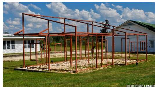
FIGURE 5-7. Ghost structures at Tuskegee Airmen National Historic Site were constructed to indicate the scale and shape of missing buildings. National Park Planner (npplan.com).
