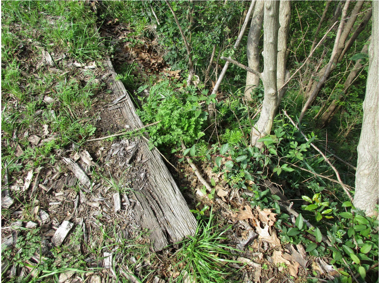
Figure 71: Retaining lumber, assumed to be from the circa 1940s Fort Rosalie reconstruction.
