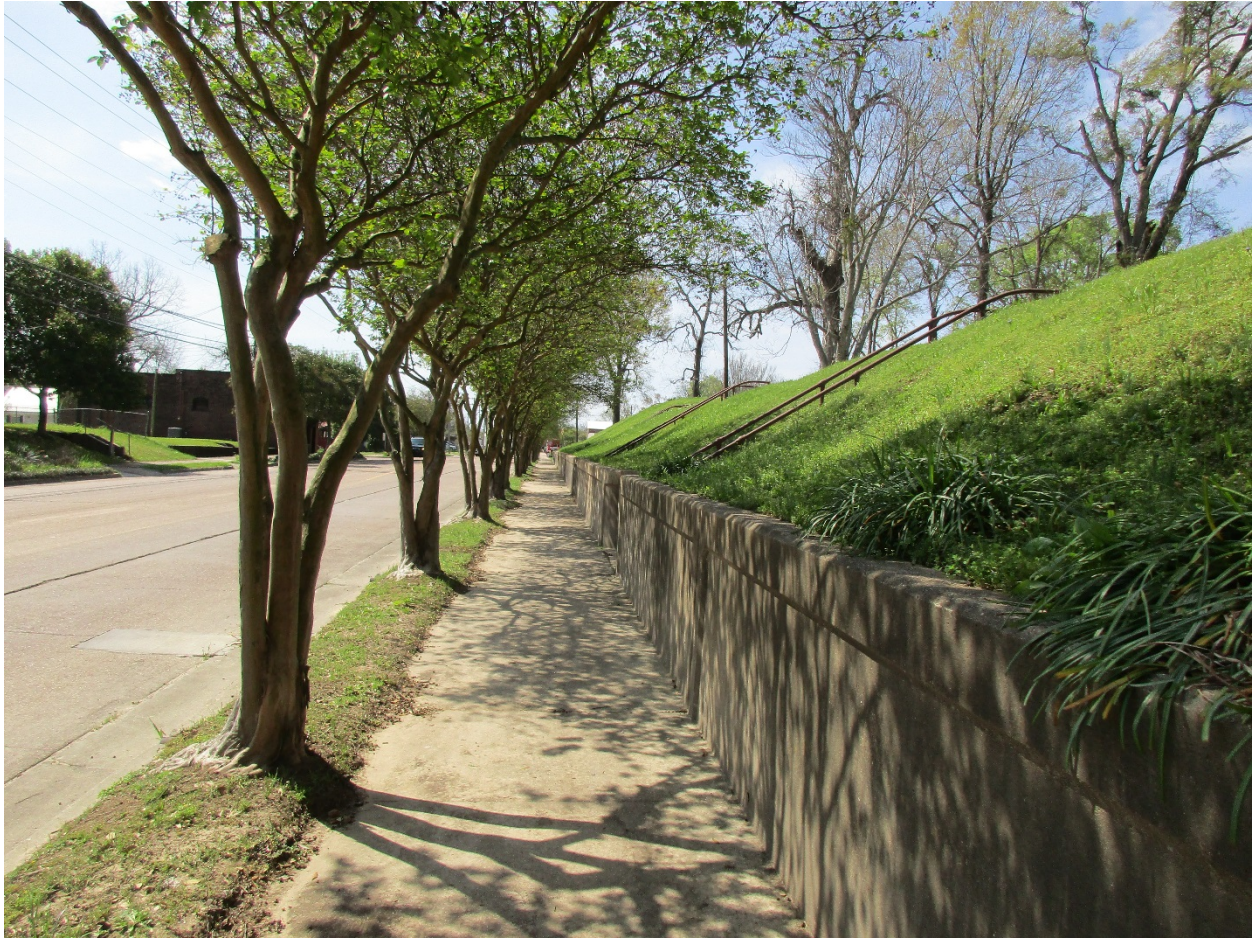
Figure 67: Concrete retaining wall associated with the early 1900s neighborhood located on site.
