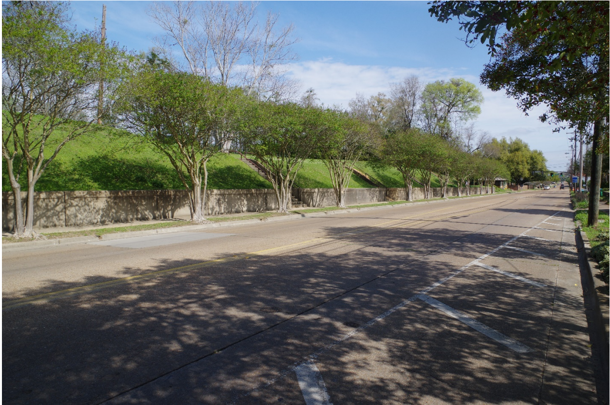
Figure 39. The concrete retaining wall is visible along South Canal Street.
