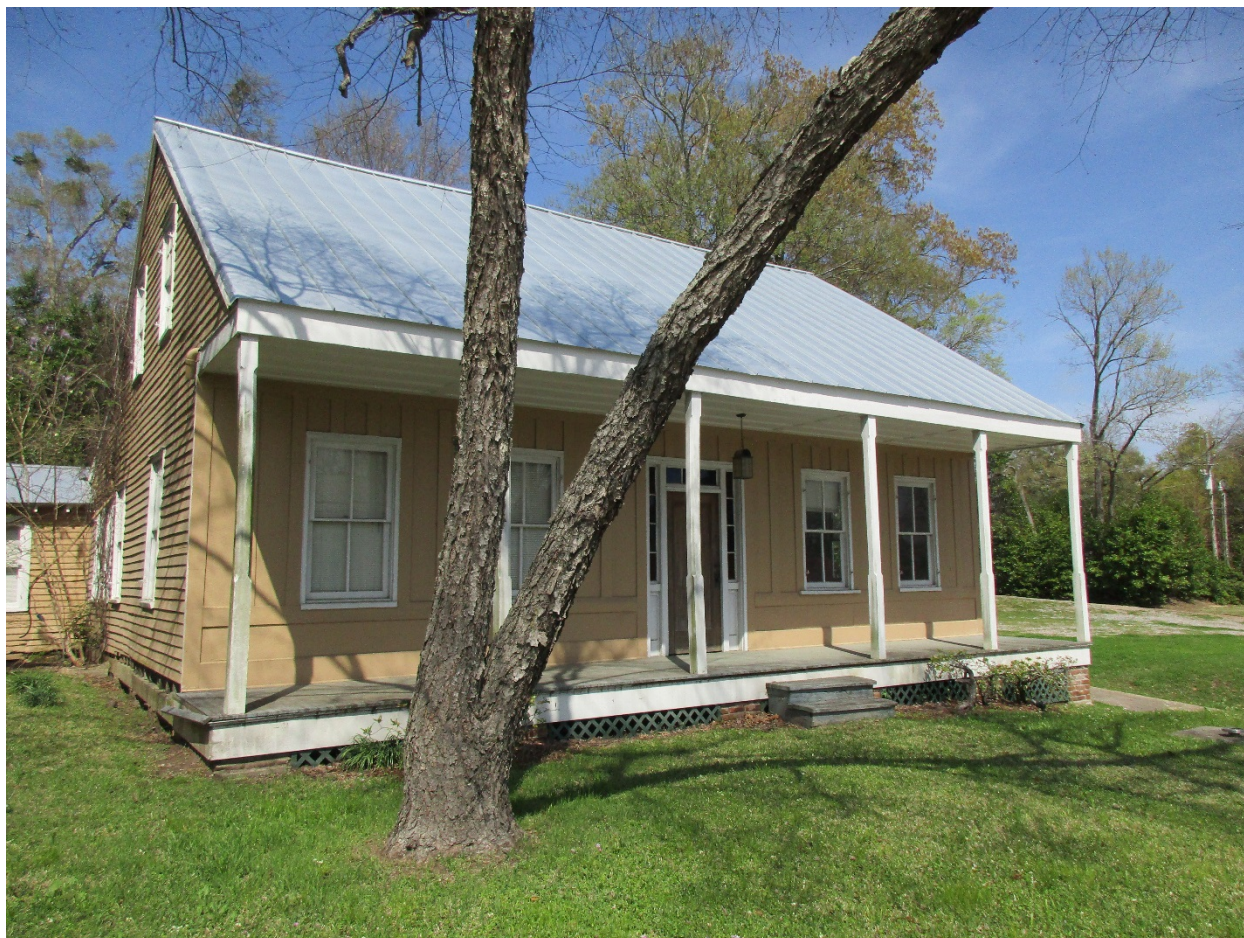
Figure 66: Stietenroth House is the only home left on the NPS property from the box factory period. Currently not in use.
