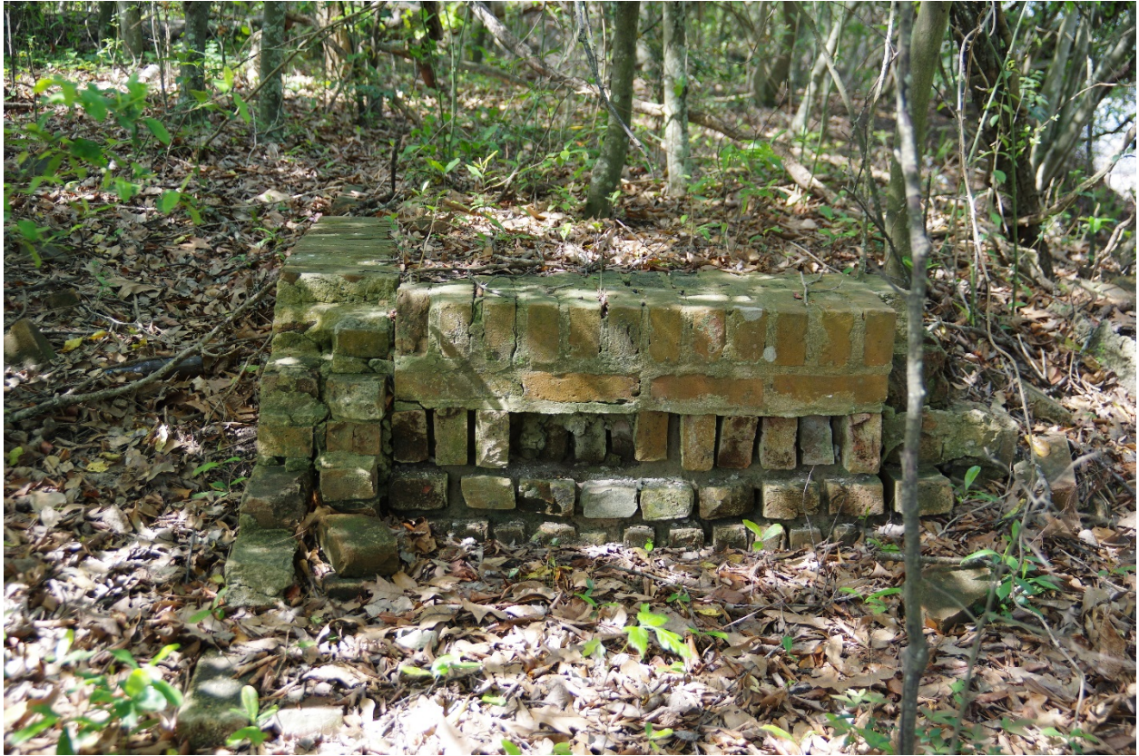
Figure 79: Brick ruins located behind the log cabin in a wooded area assumed to be associated with the circa 1940s reconstructed Fort Rosalie.
