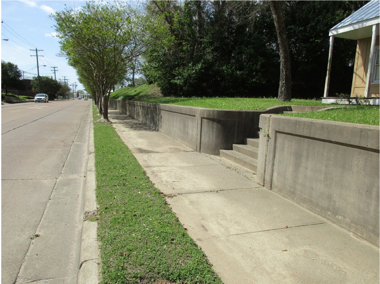
1 2 Figure 46: The retaining wall and steps leading to the Stietenroth House is associated with the Box 3 Factory era.
