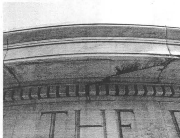
Photo 9. Crack extending from right joint to center of the cornice soffit.
