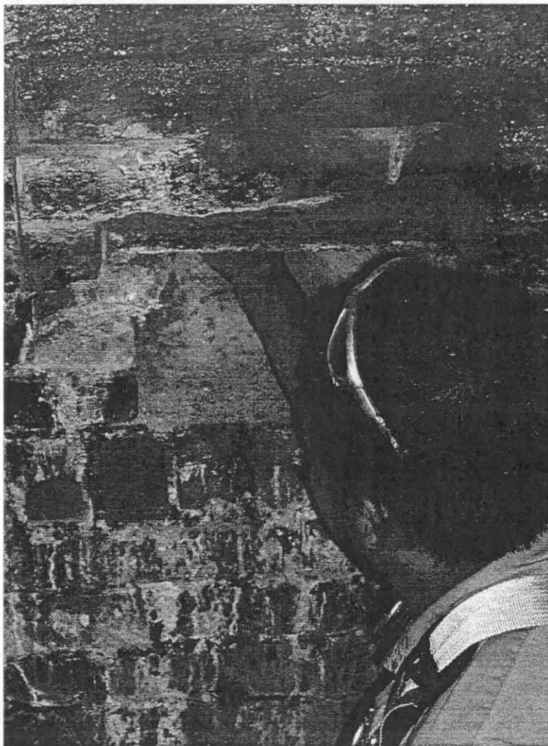
Binh Nguyen of the National Park Service investigating the void between the steel angle tension ring and the marble construction beyond. [JGWA, 2005]
