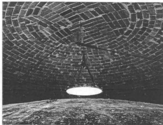
Photo 4. Interior surface of outer dome and counterweighted ceiling oculus.
