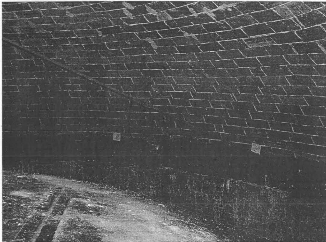
The tile construction of the upper dome bears on the brick drum below. [JGWA, 2005]
