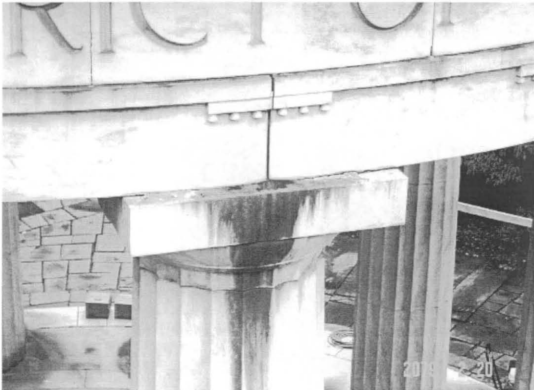
An open head joint above a column. [MSSC, 2005]
