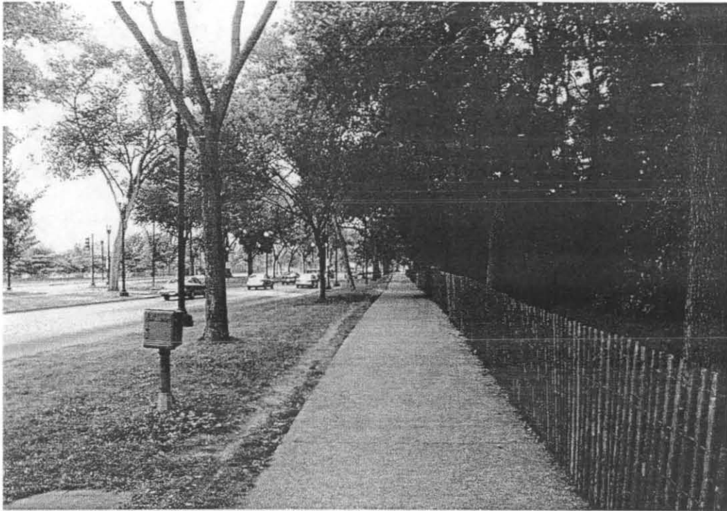
Exposed aggregate walk along Independence Avenue. [EDC, 2005]
