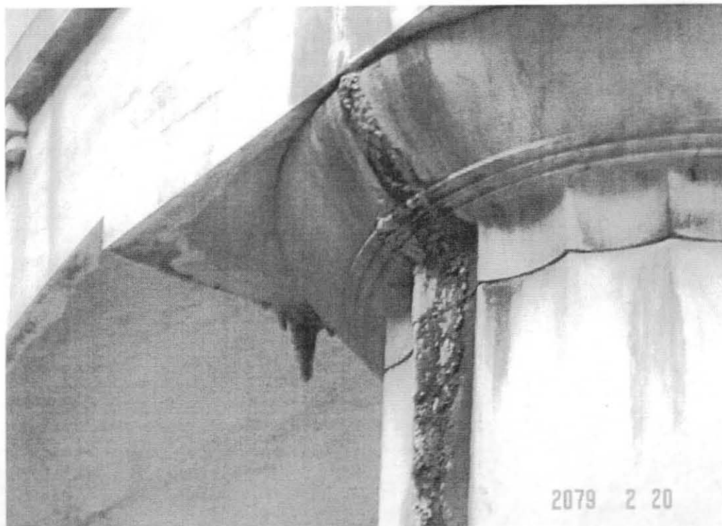
Stalactite on base of entablature. [MSSC, 2005]
