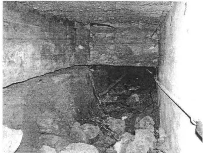
Photo 18. Concrete grade beams.
