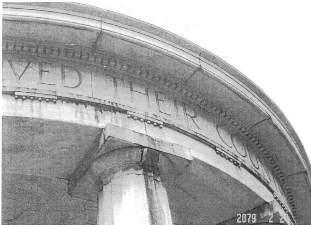
Mortar is missing and deteriorated in many locations on the entablature. [MSSC, 2005]
