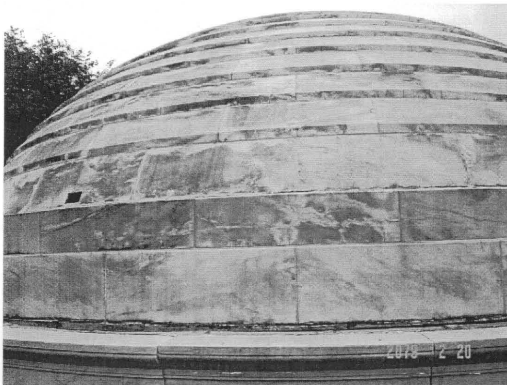
The marble of the dome exhibits dark mottling. [MSSC, 2005]
