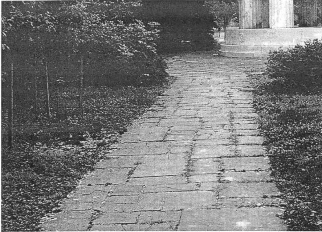
Weed infiltration along the flagstone walks. [EDC, 2005]
