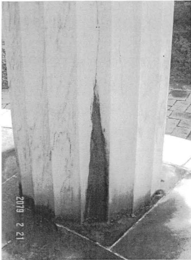
Severe dark-colored vertical stain at the base of column 4. [MSSC, 2005]
