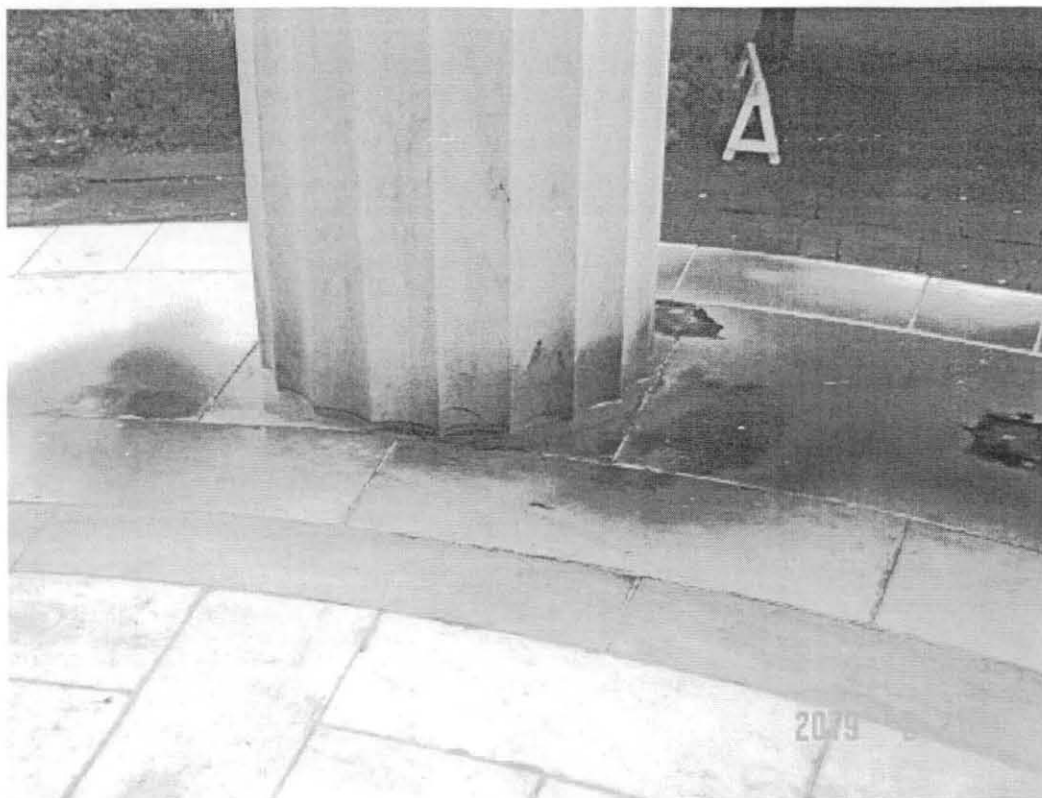
Dark-colored soiling and water pooling on marble floor near base of column. [MSSC, 2005]
