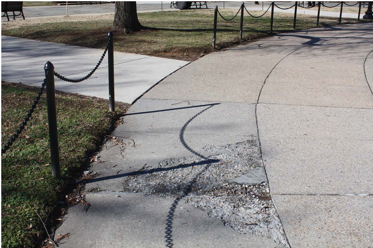
11. Concrete detail Direction: West
