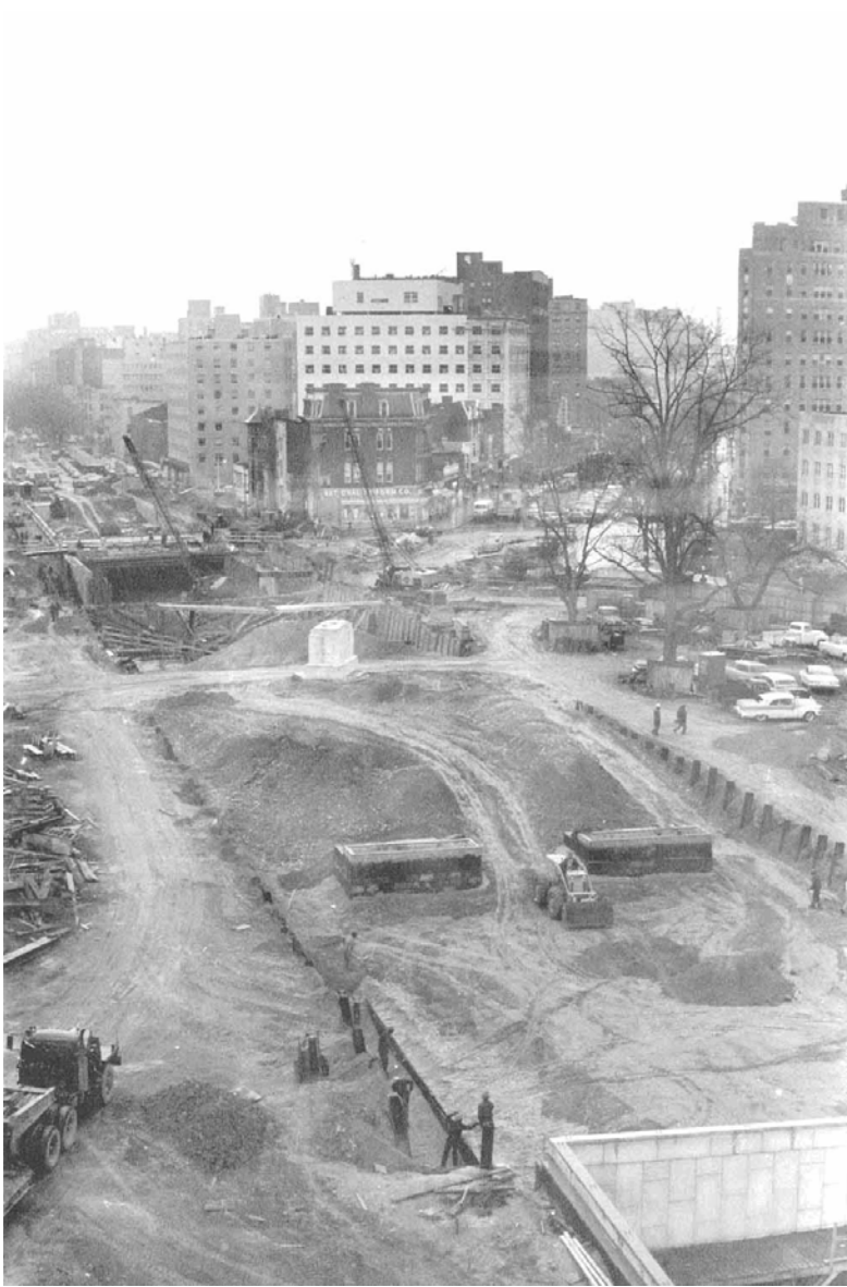
K Street underpass construction, c. 1961 (Washingtoniana Collection).
