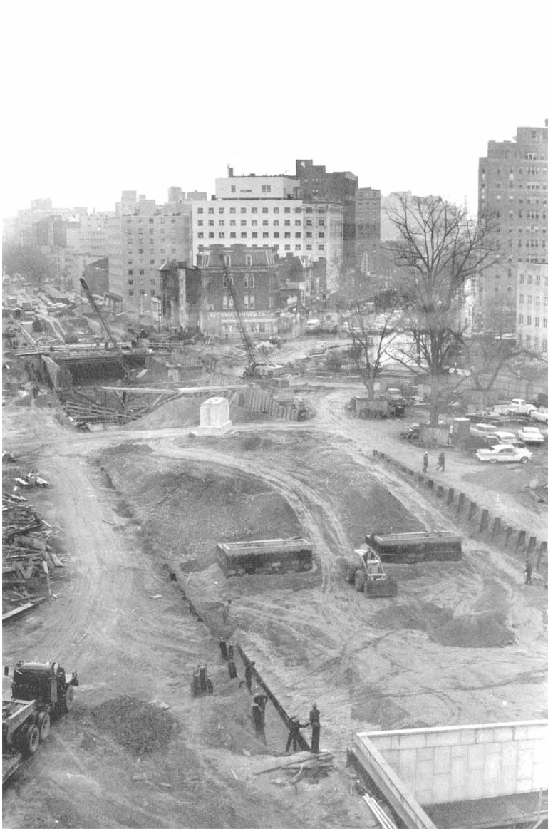
K Street underpass construction, c. 1961 (Washingtoniana Collection).
