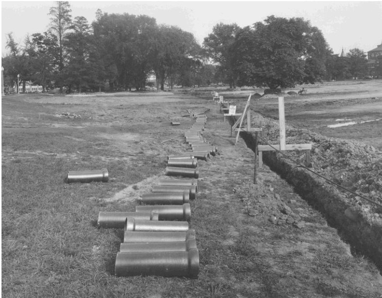
Grading and the laying of utilities on the Mall. In the distance can be seen some of the tree wells built around mature trees to be moved. (from MRCE; CLP file "Mall grading 7-12 Sts")
