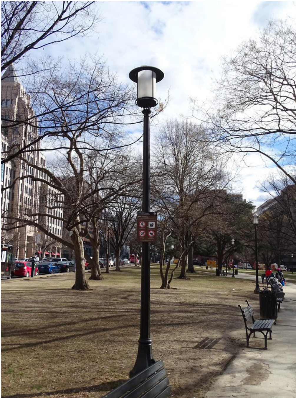
Example of the Saratoga style lights found in Franklin Park. (NCR CLR 2017)
