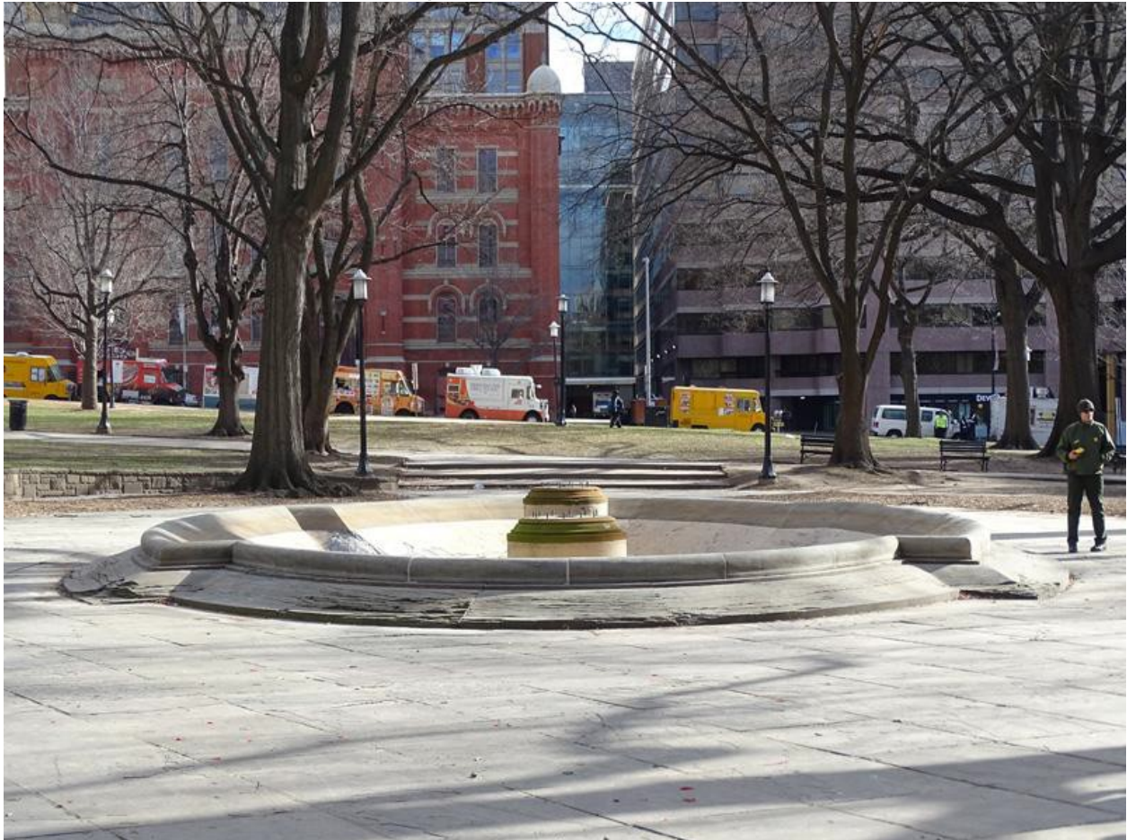
Current condition of the fountain facing east ( NCR CLP 2017)
