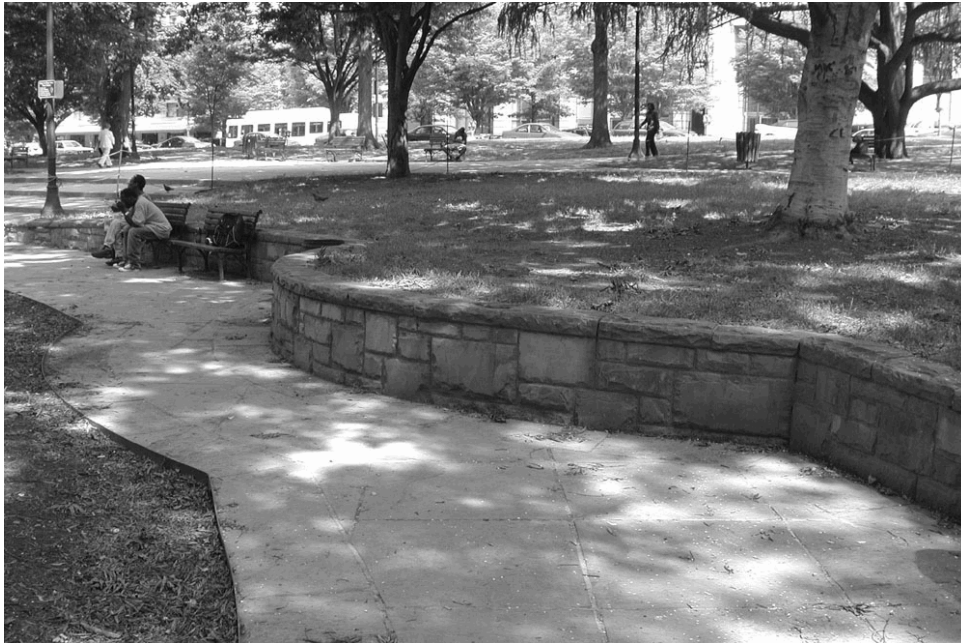
This rough-faced ashlar stone retaining wall extends along the plaza's northeast quadrant and incorporates a rounded projection, allowing for tree roots. (July 2004; CLP digital photofile "Franklin Park/CLI/SSF/stone wall looking W")
