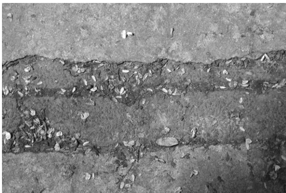
In areas on the walks where the 1976 synthetic bitumen paving has broken off, expansion joints of the 1936 asphalt paving are visible. (July 2004; CLP digital photofile "Franklin Park/CLI/circulation/pavement joint")
