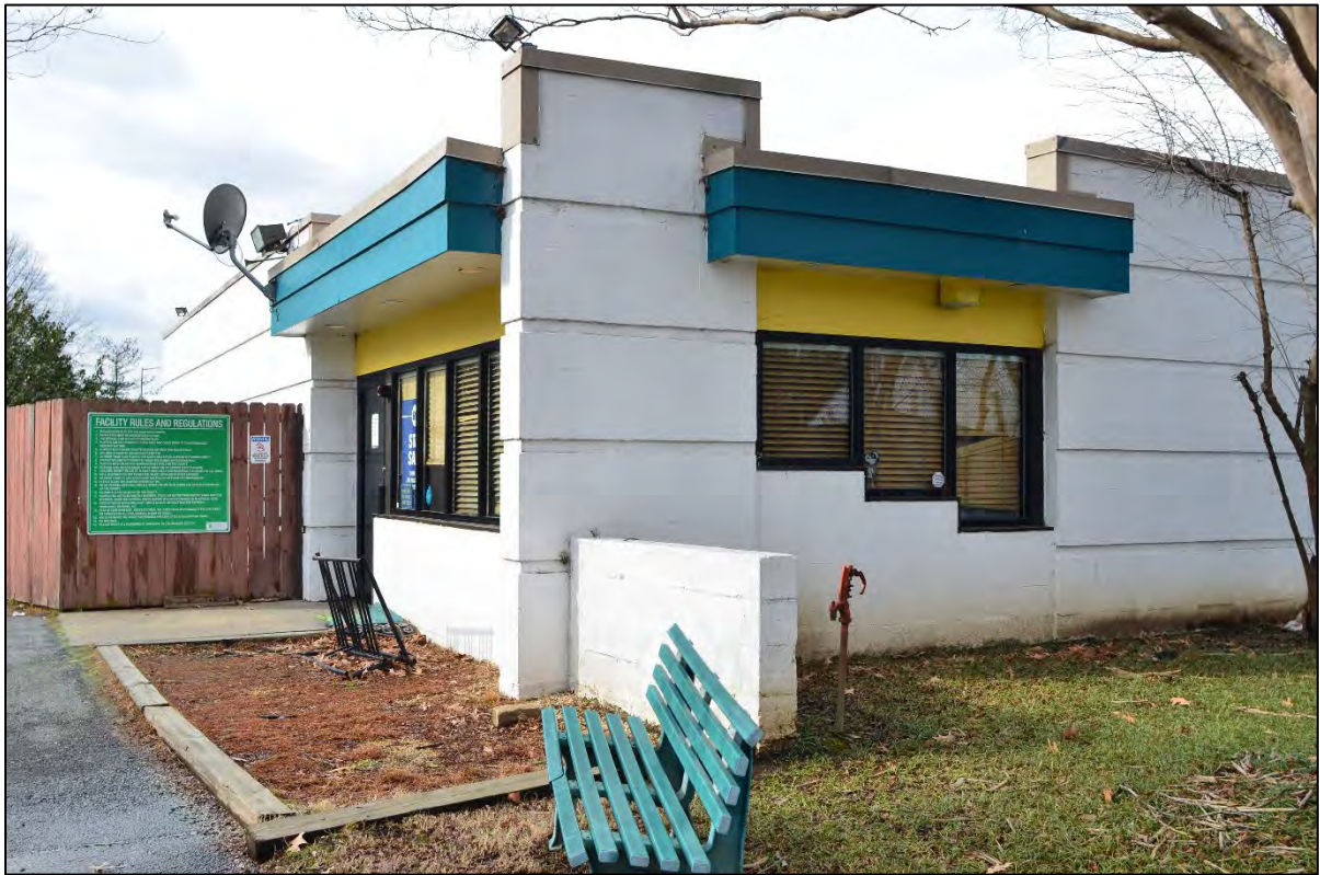
Fig 79. Photo looking northwest depicting East Potomac Park Tennis Administrative Building (Matthew Traucht 2021).
