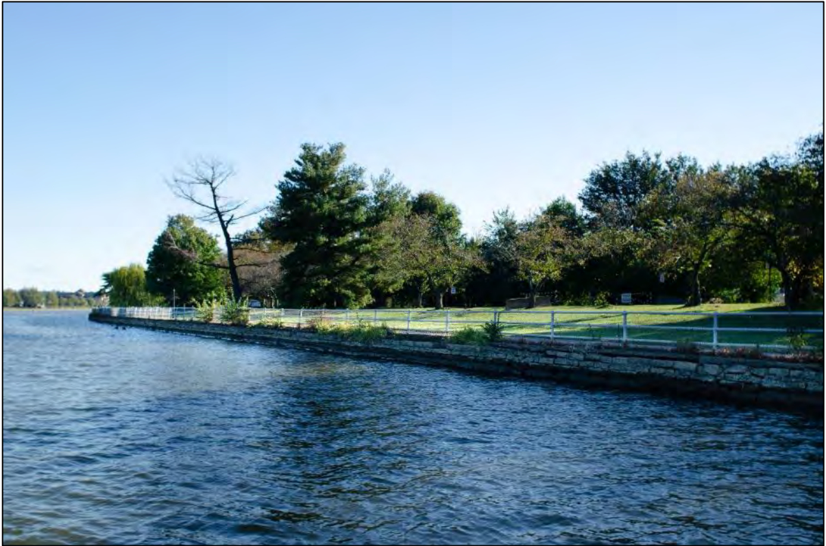
Fig 62. Photo looking southerly depicting seawall on Washington Channel side of island (Matthew Traucht 2021).
