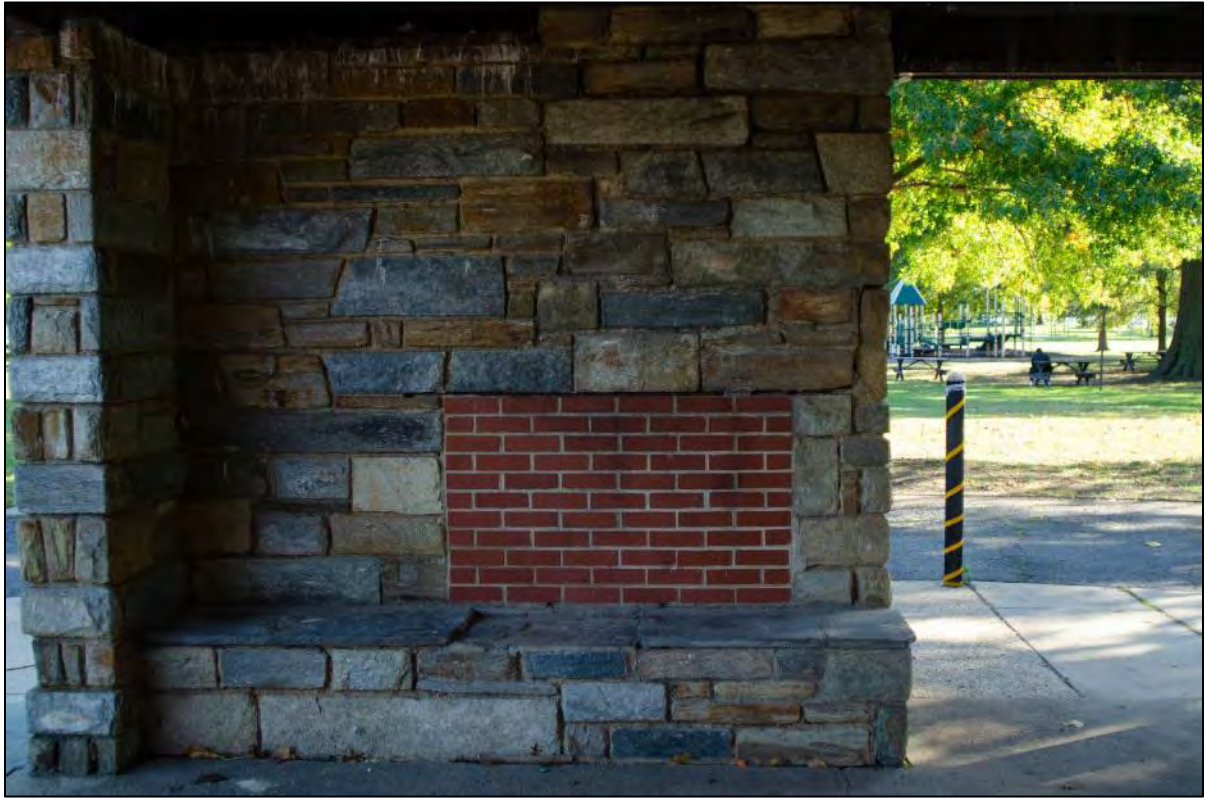
Fig 65. Photo looking south depicting filled fireplace in Mission 66 Comfort Station “Type B” (Matthew Traucht 2021).
