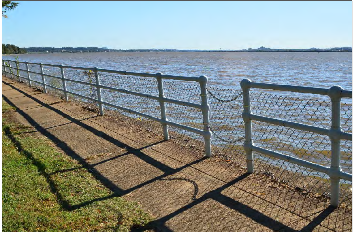
Fig 97. Photo depicting pipe railing in East Potomac Park. Occasional openings occur along the length of the railing at irregular intervals (Matthew Traucht 2021).
