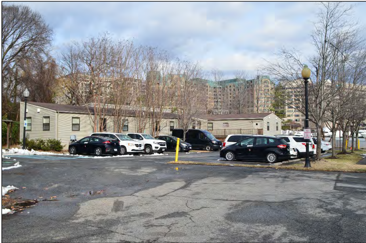
Fig 61. Photo looking northeast depicting modular office trailers to the north of the US Engineers' Storehouse(Matthew Traucht 2022).
