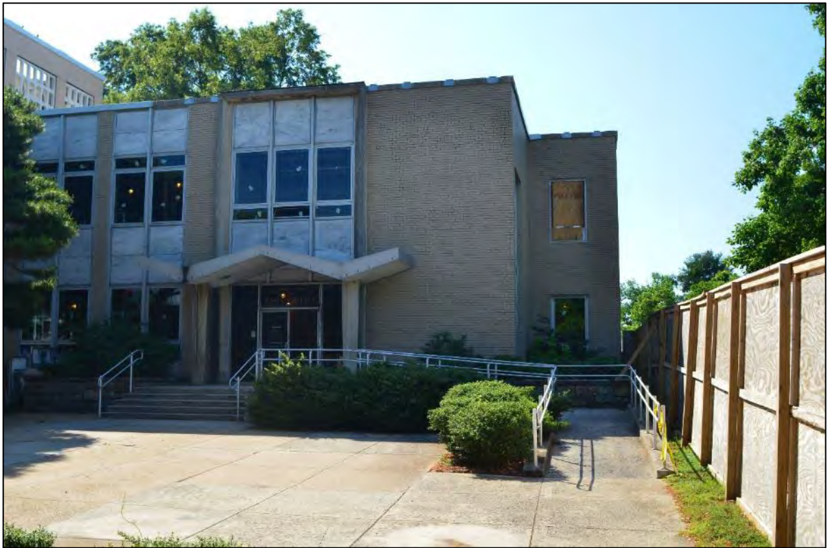
Fig 74. Photo looking south depicting entrance terrace at the United States Park Police Headquarters Building. Note noncontributing accessible ramp (Matthew Traucht 2021).
