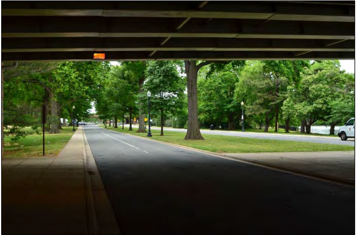
Fig 57. Photo looking northwest showing Ohio Drive SW from beneath the Francis Case Memorial Bridge, note planted median and sidewalk, Potomac Railroad Bridge in distance (Matthew Traucht 2021).
