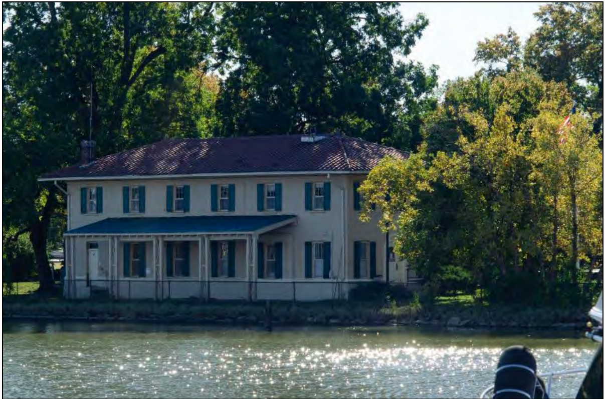
Fig 60. Photo looking west across Washington Channel depicting U.S. Engineers' Storehouse (Matthew Traucht 2021).
