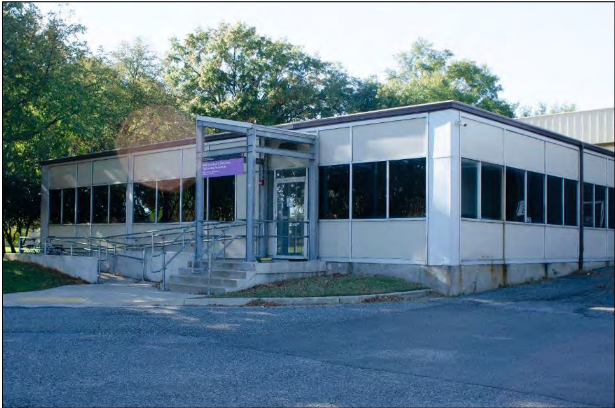
Fig 81. Photo looking west from Buckeye Drive SW depicting the Buckeye Building, formerly the Tourmobile Headquarters, which houses the Interpretation & Education and Partnerships-Volunteer divisions (Matthew Traucht 2021).
