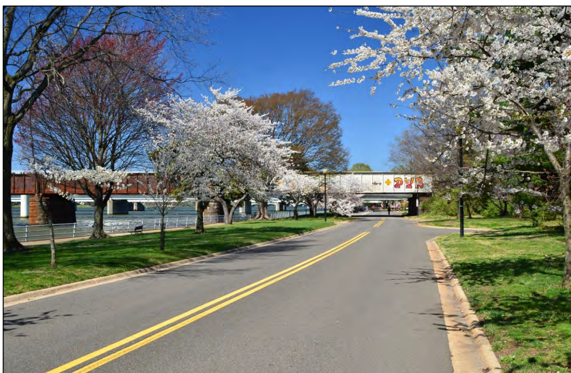
Fig 7. Photo looking northwest along Ohio Drive SW depicting Potomac Railroad Bridge as it crosses the Potomac River and enters East Potomac Park (Matthew Traucht 2021).
