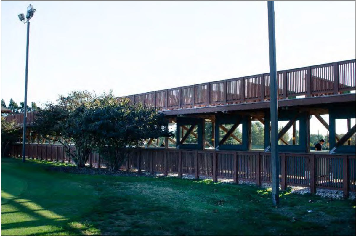
Fig 72. Photo looking southwest depicting East Potomac Park Driving Range Structure (Matthew Traucht 2021).
