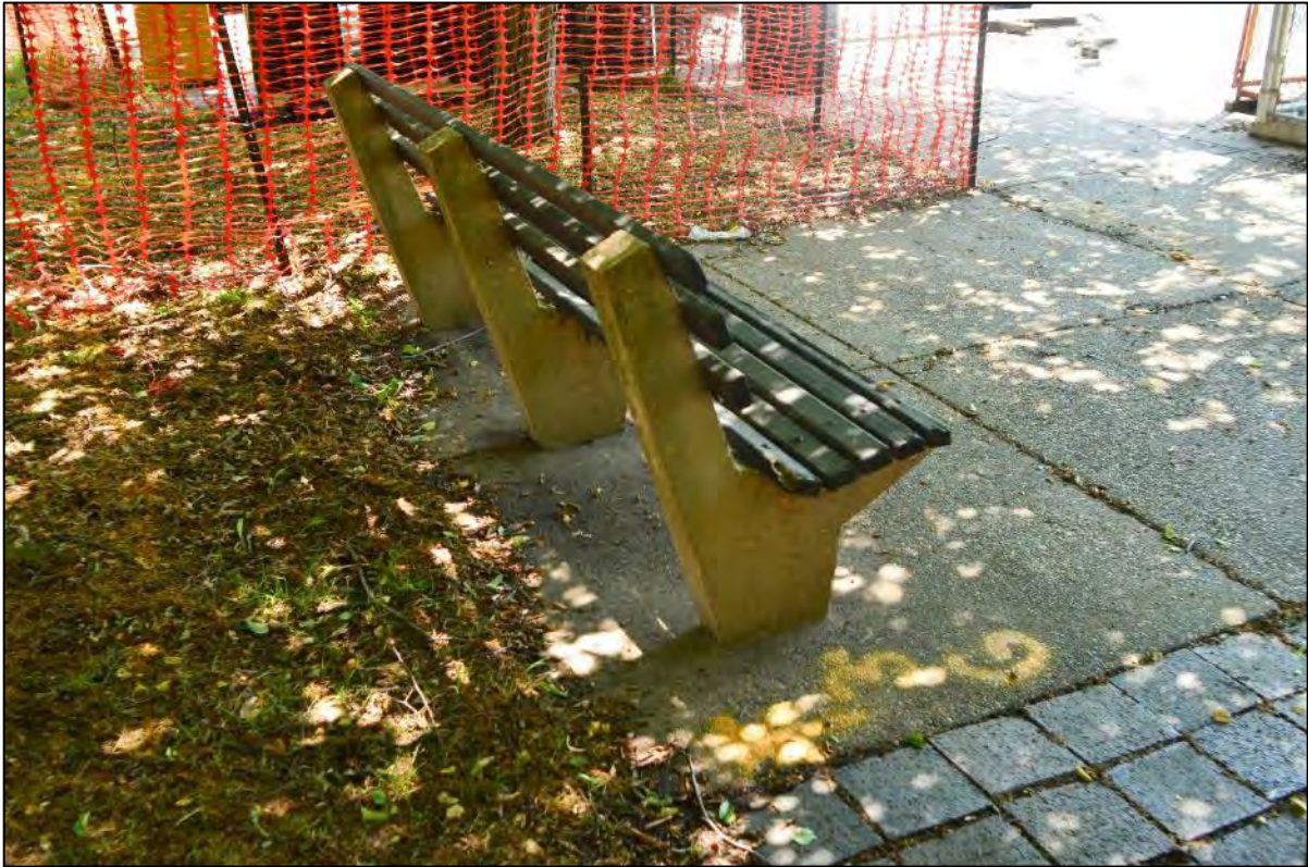
Fig 102. Photo of concrete and wood benches at the NCR Headquarters (Matthew Traucht 2021).
