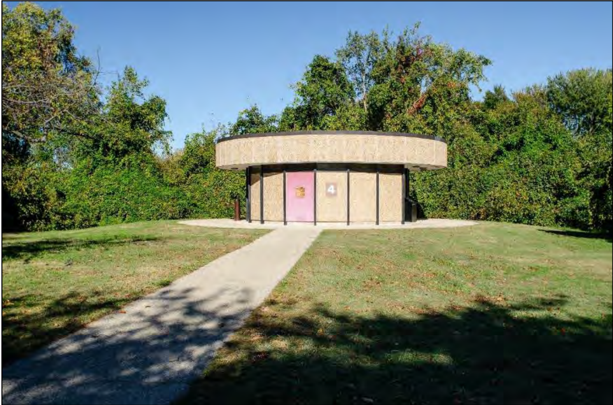
Fig 66. Photo looking northeast depicting Elliptical Comfort Station (NPS Restroom #4) on west side of East Potomac Park (Matthew Traucht 2021).
