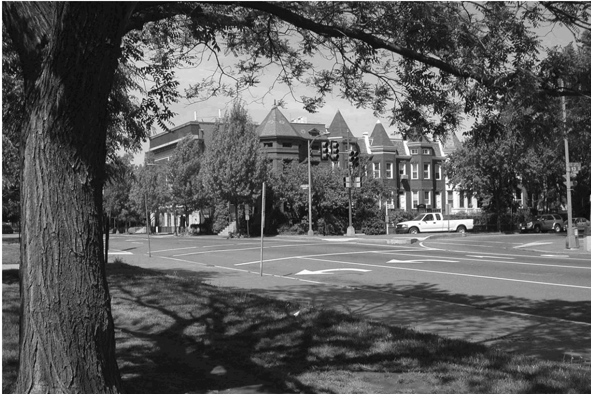
Rowhouses along East Capitol Street, seen from east end of park. Lincoln Park is surrounded by well-maintained late-Victorian structures, vividly conveying a sense of the historic neighborhood. (final images/rowhouses along E. Capitol St.)
