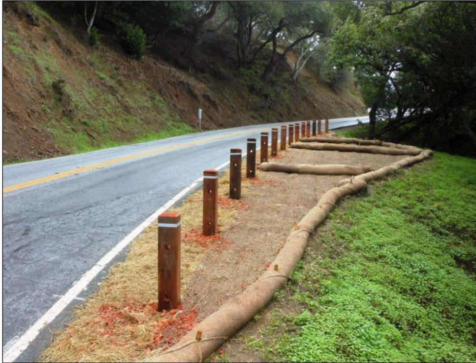
FIGURE 12. POST INSTALLATION AND EROSION CONTROL MEASURES
