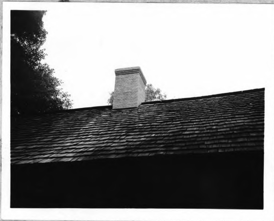
3. North and west sides of the repaired chimney.
