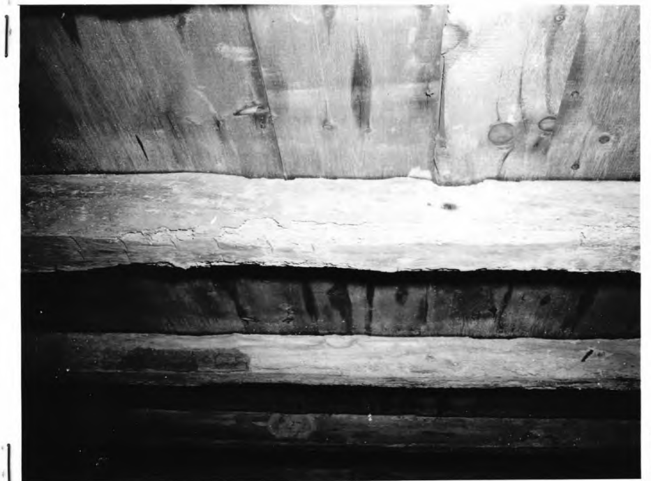
5. Another view of floor joists.
