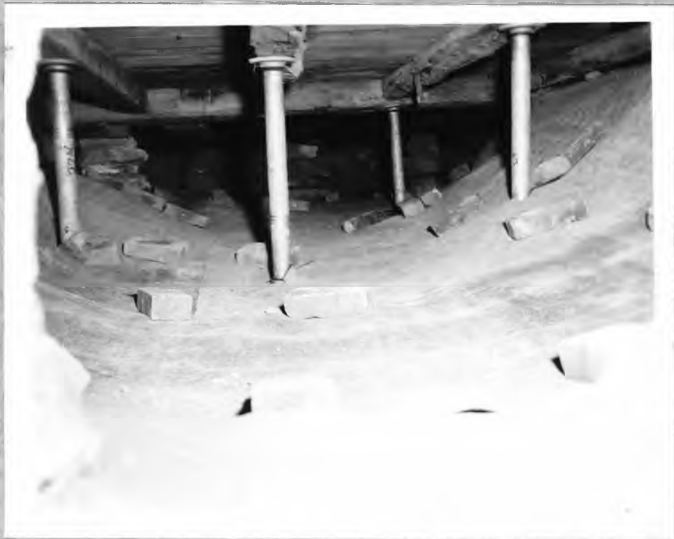
9. The deepened crawl space.
