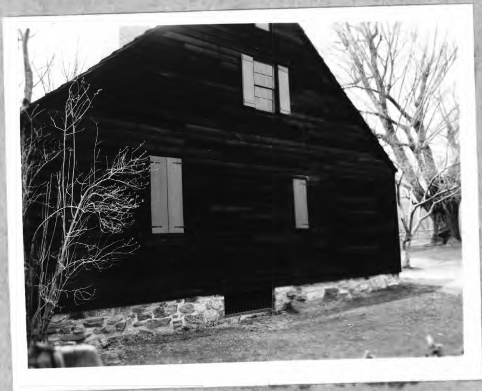
11. The east end after oiling.
