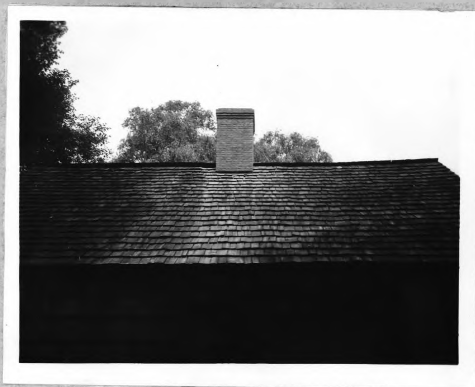
4. North side of the repaired chimney.
