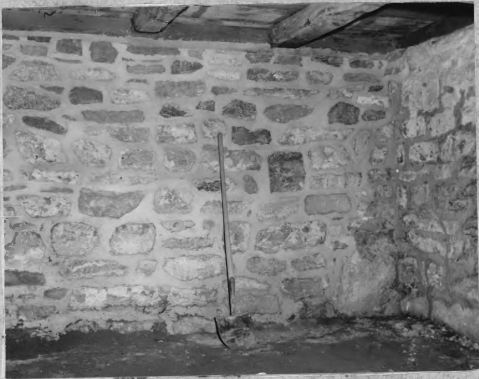
7. The rebuilt cellar wall.
