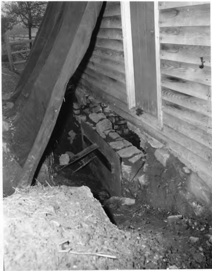
6. The reconstruction of the north basement wall.
