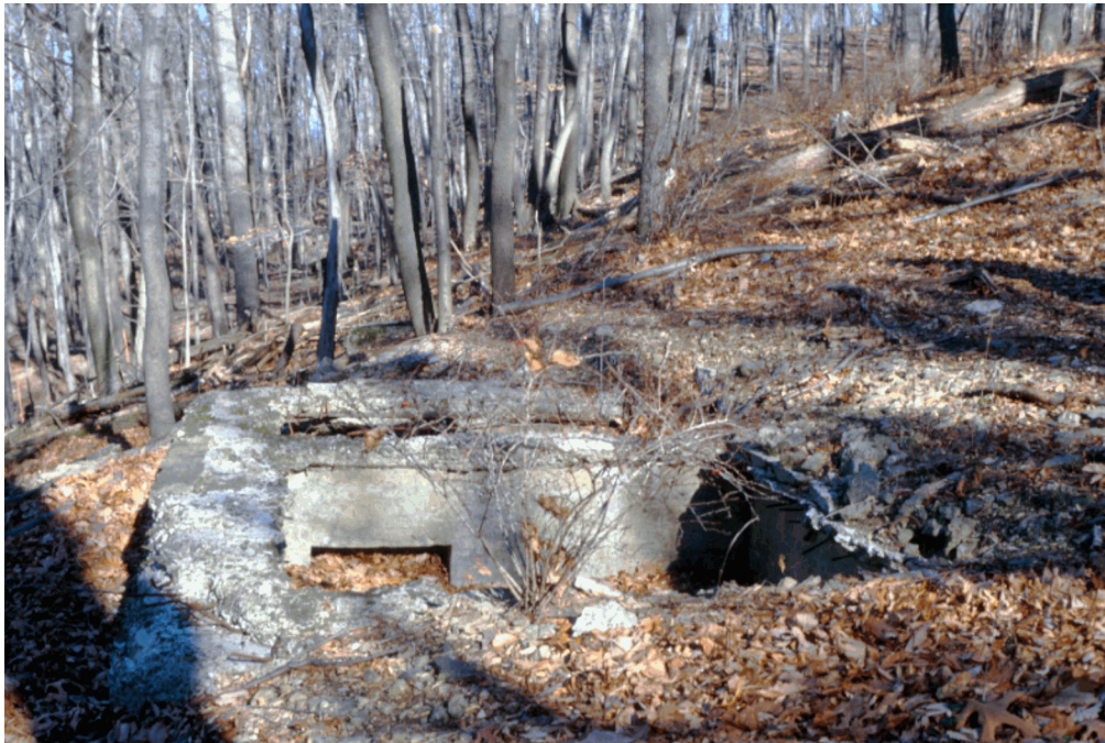
Restroom foundation (OCLP 1998).
