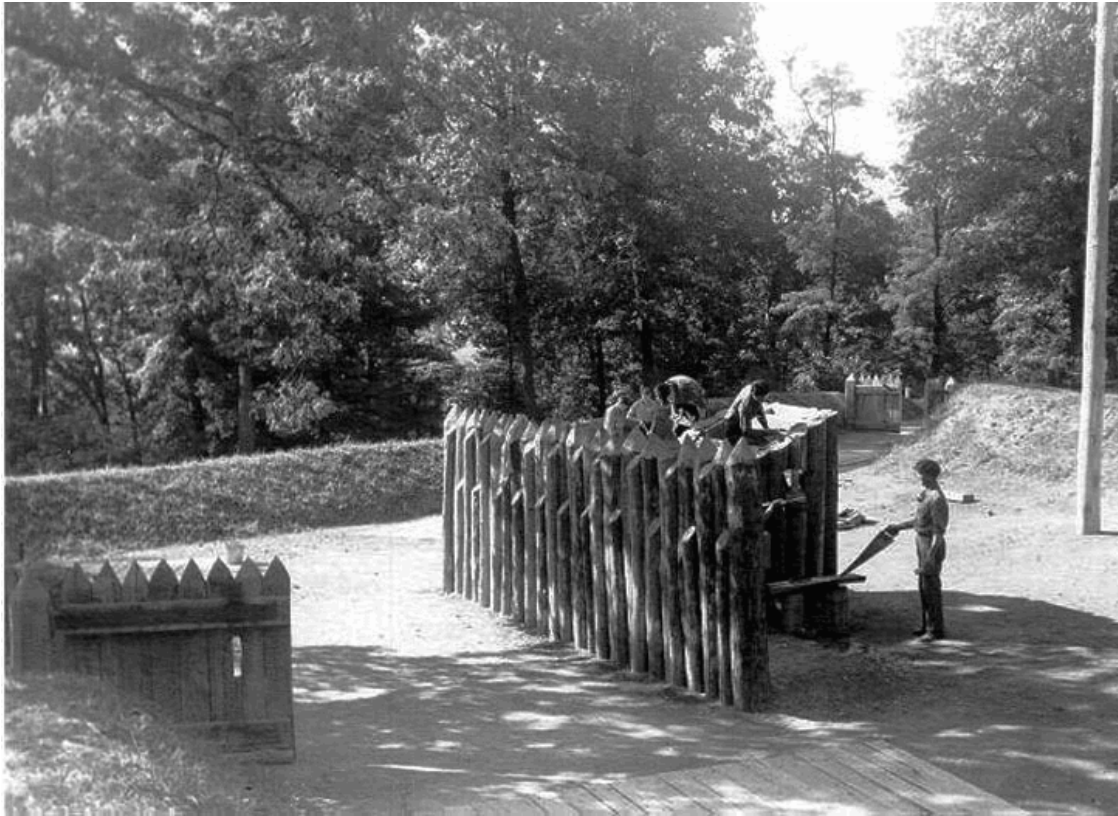
CCC Reconstructed Fort Nonsense timber picket gates and earthen parapets, 1937 (CCC Photo Scrapbook, MORR NHP Archives).
