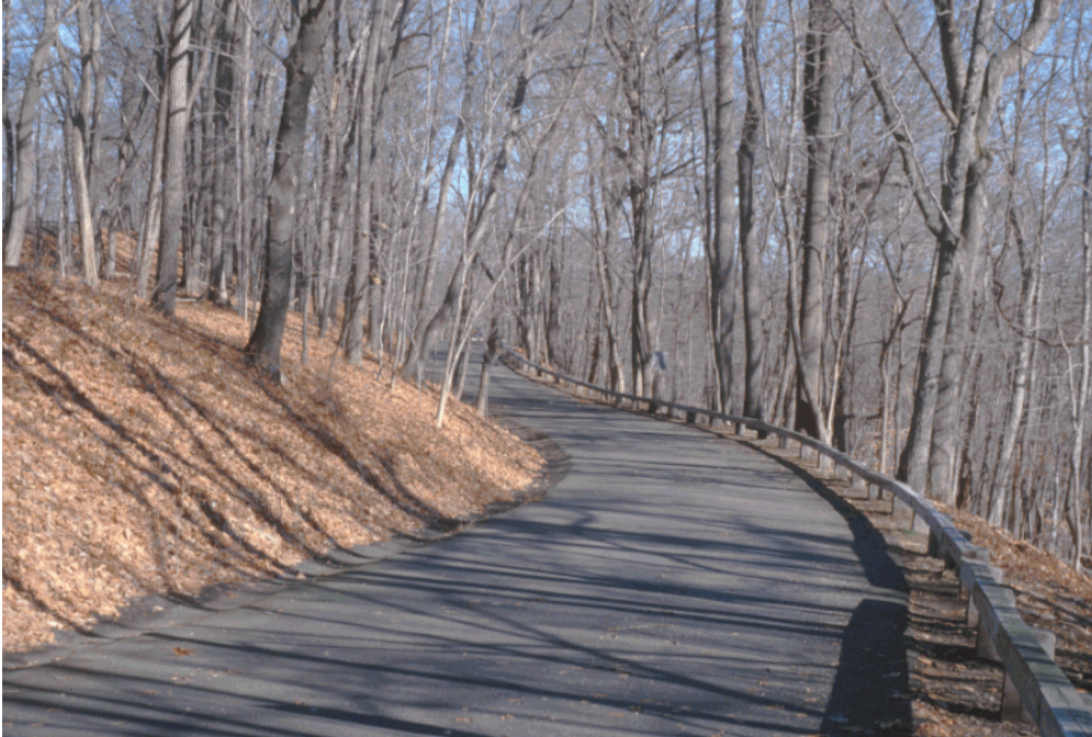
Timber guard rail along park access road (OCLP, 1998).
