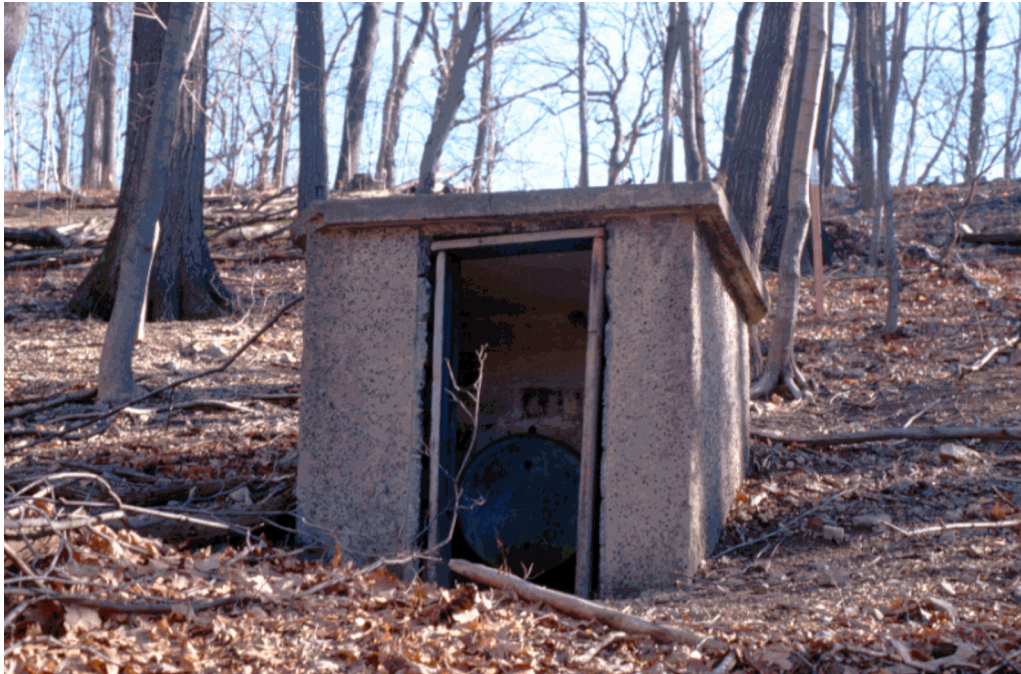
Restroom pumphouse (OCLP, 1998).
