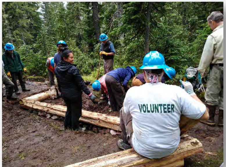
Volunteers working on a maintenance project. NPS Photo: Bacher
