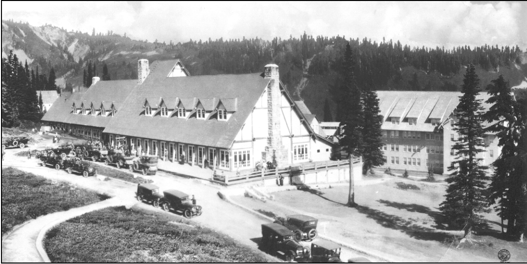
Figure 5. Paradise Inn and Annex in the 1920s.
