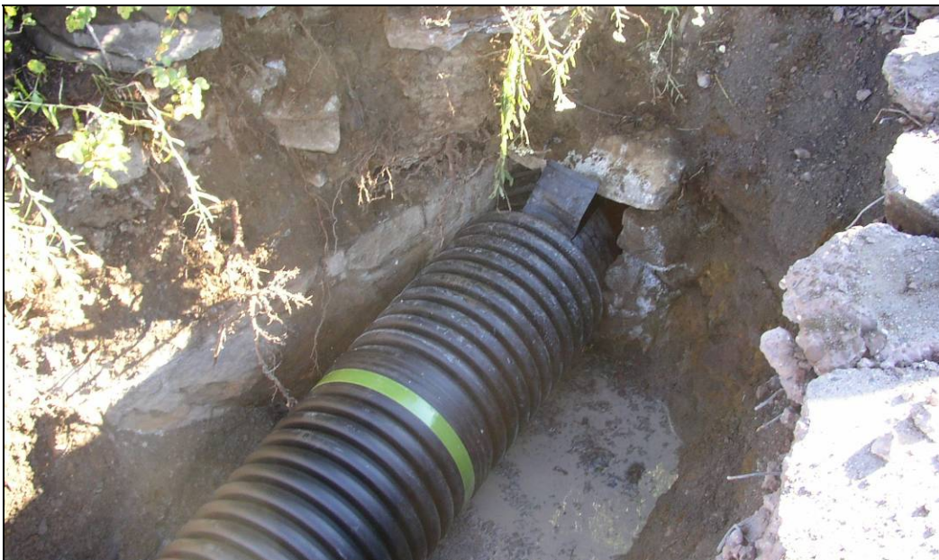
Figure 49. Slab Lined Aquaduct/Drain Feature 7.
