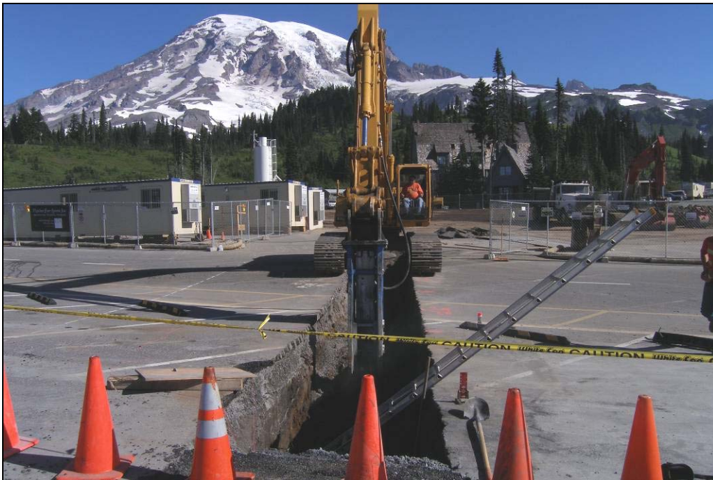
Figure 44. Trenching for Storm Drain
