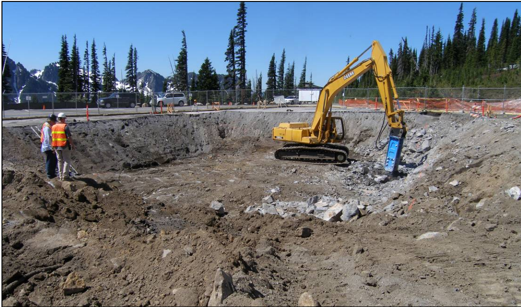
Figure 31. Excavating Paradise Visitor Center Foundation.
