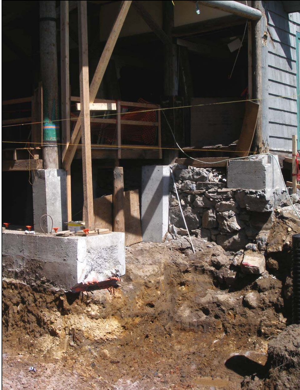
Figure 37. South Chimney Foundation Excavation
