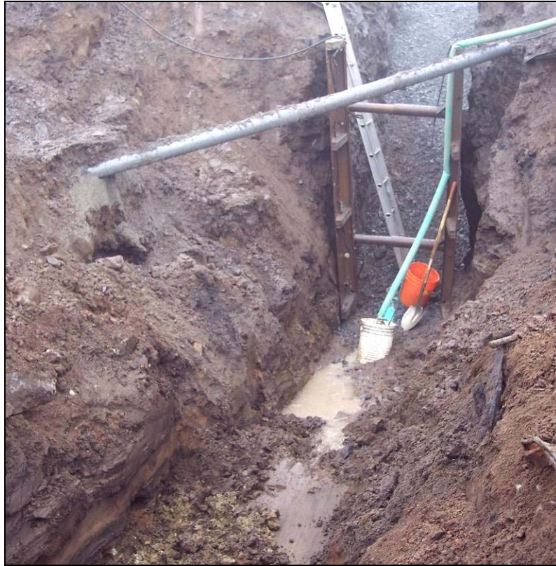
Figure 47. New Sewer Line Trenching in Progress.
