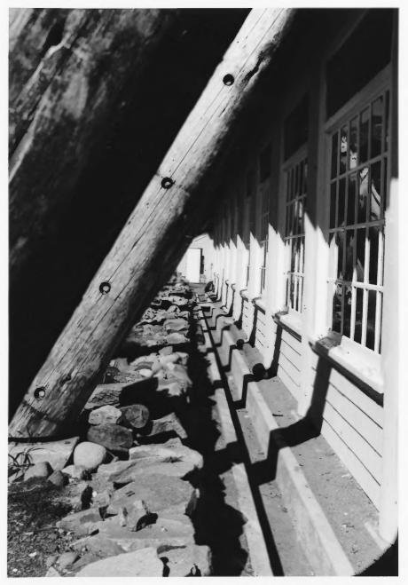
Steel Buttress Encase in Log Sheathing and concrete drain on the Exterior of the Dining Room
