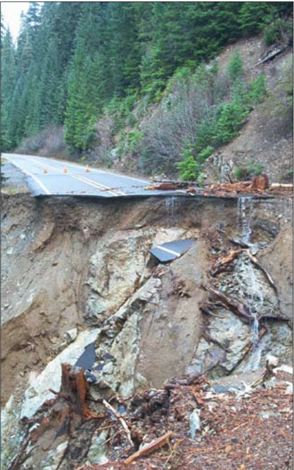
Highway 123, between Ohanapecosh and White River, suffered four washouts. Repairs cannot begin until winter snows have melted.
