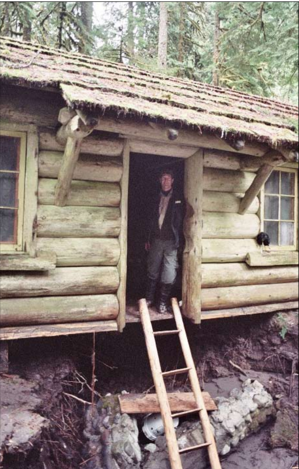
Above: A channel of the Carbon River carried away the ground beneath the historic Ipsut Creek Cabin.
