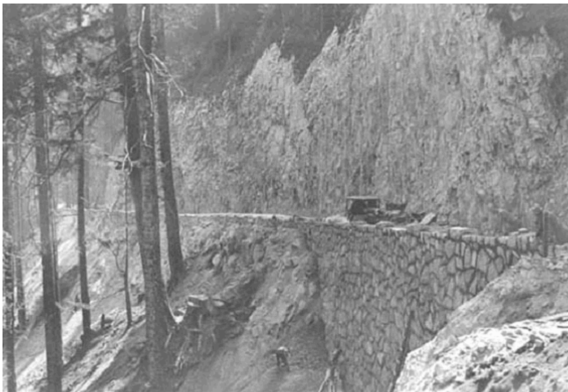
Historic photo showing a stone retaining wall and large rock cut along the North Puyallup segment, ca. 1934 (MORA Archives).
