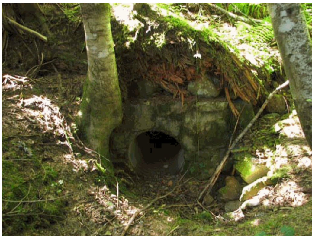
Contemporary photo showing a culvert with a stone headwall, 2005 (MORA).
