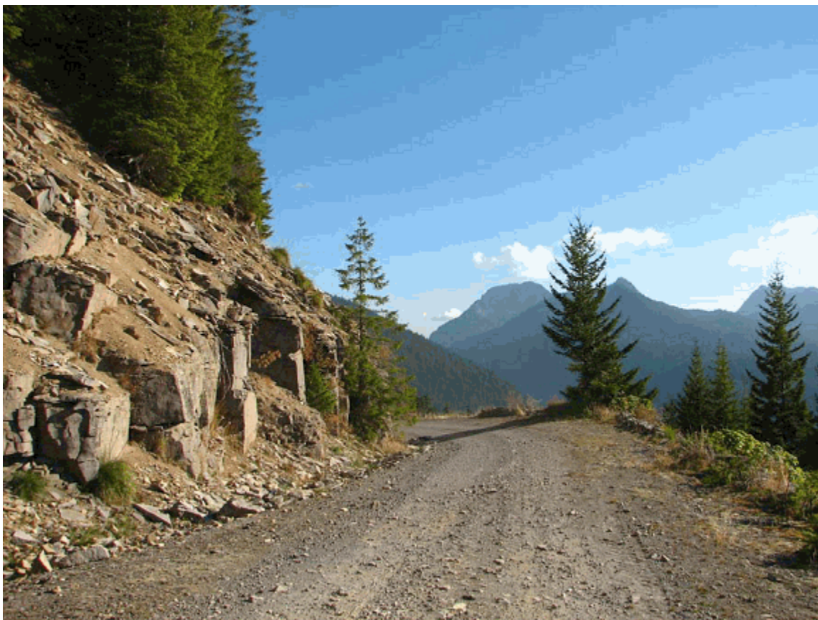
Contemporary photo showing road bench near Klapatche Point. Note the stone guardwall to the left and right of the tree closest to the road and jagged rock cut, 2005 (MORA).
