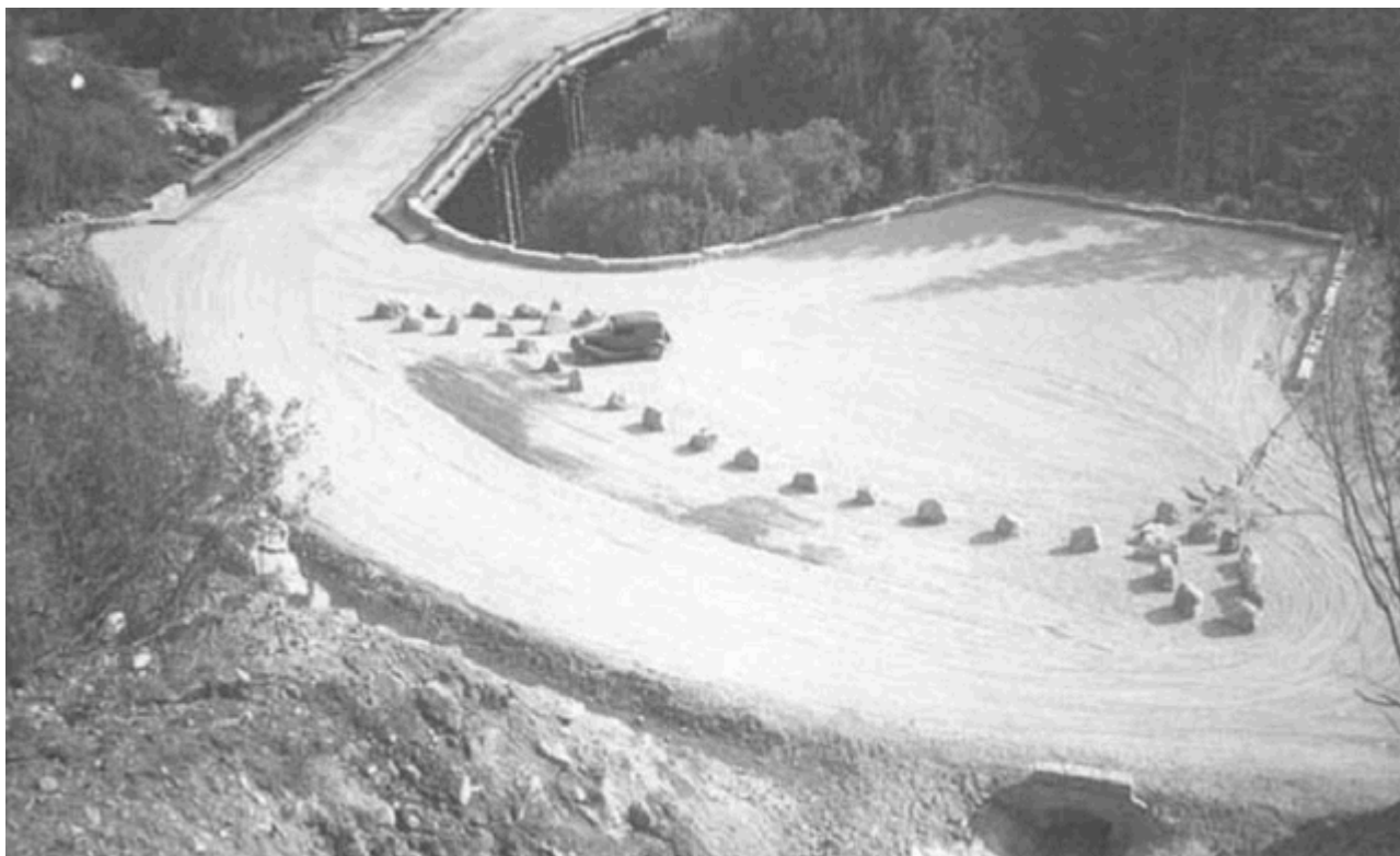
Historic photo showing a large turnout, rock barrier, box culvert, and rustic log bridge, on the north bank of the North Puyallup River ca. 1934 (MORA Archives).
