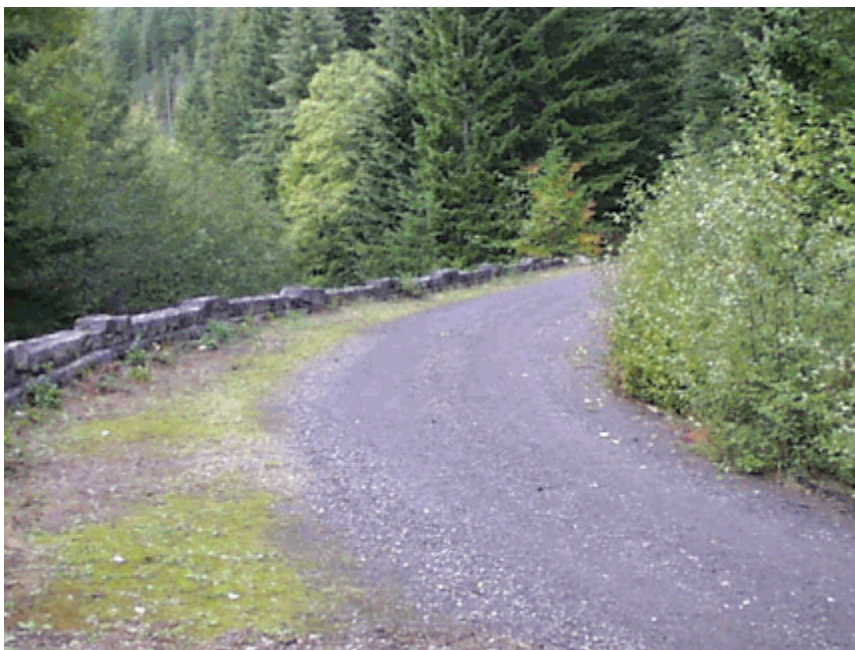
Contemporary photo showing a type 2B stone guardwall at Tahoma Vista, 2004 (MORA).
