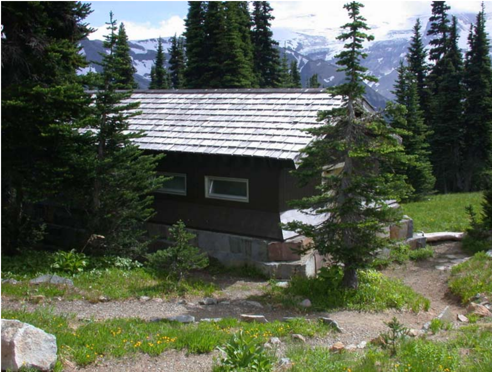
Contemporary photograph of the Sunrise Picnic Area Comfort Station. (PWRO 2002) This building was constructed in the 1930s, but the wooden portion of the walls and roof have been so altered that it has lost integrity and is no longer contributing. The stone foundation walls still remain, however, and this comfort station has the potential to be restored.
