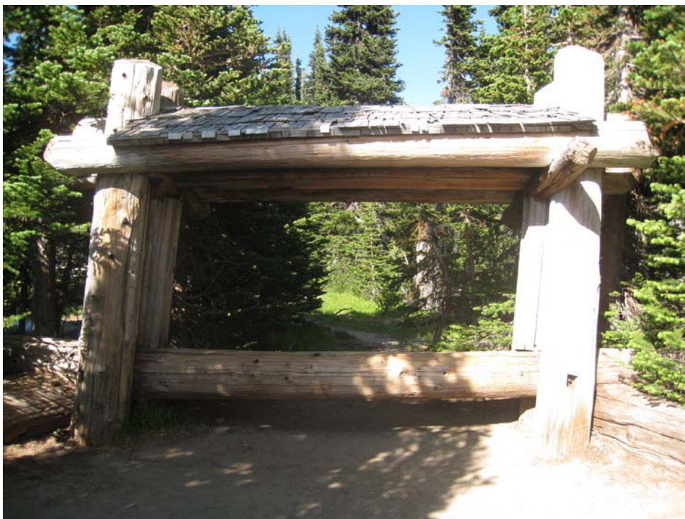
Contemporary photo of exhibit kiosk built by the CCCs at the historic Rim Trail Overlook #2.. The kiosk is leaning to the right and is missing roof shingles. (PWRO 2002)
