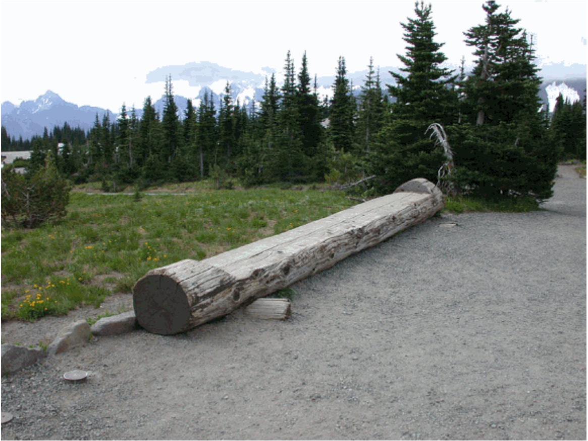
Contemporary photo of historic whole-log bench. The log support footings have decayed causing the bench to sink onto the ground. (PWRO 2002)
