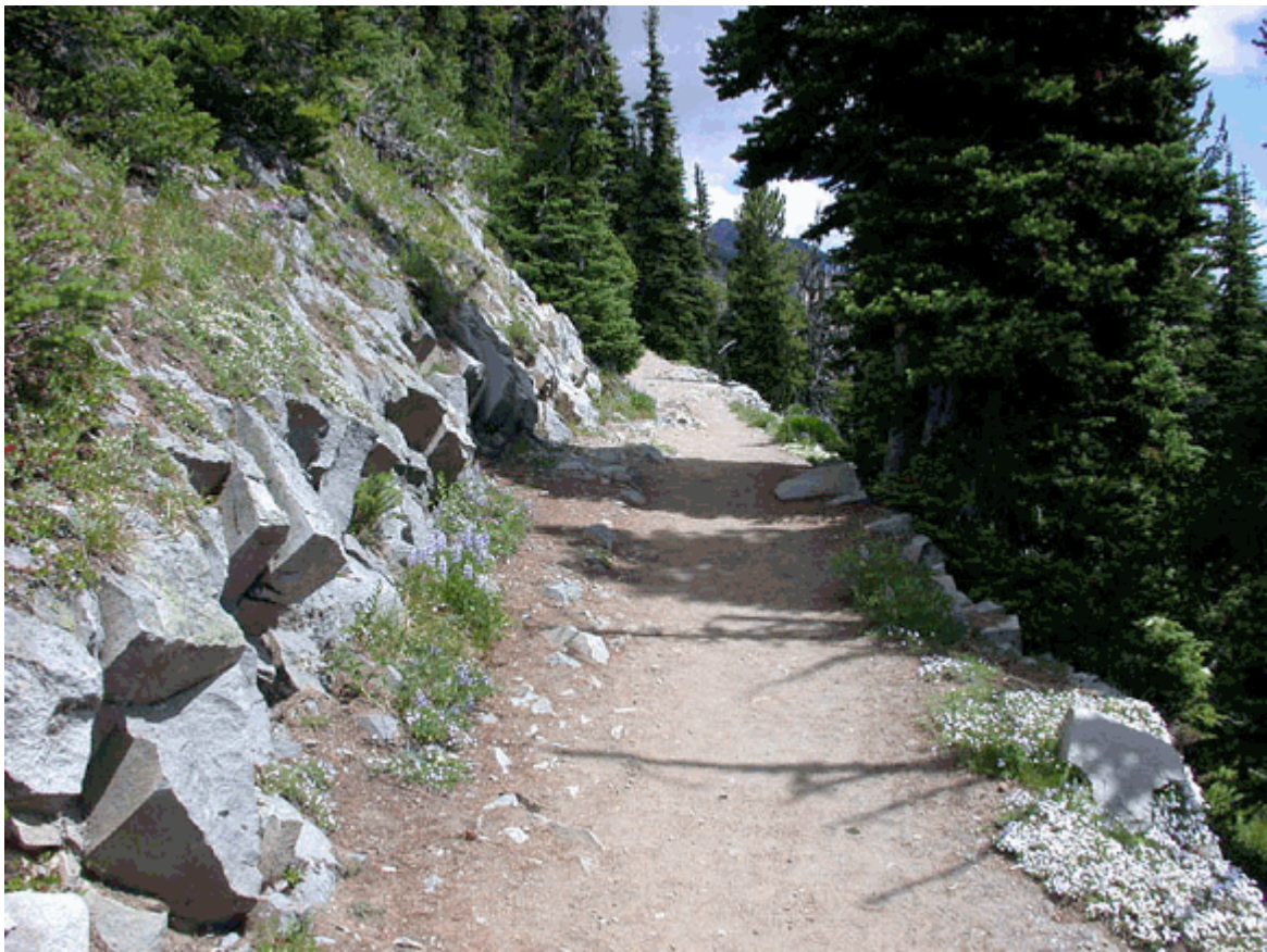
Contemporary photo of Sourdough Ridge Trail northwest of Sunrise showing dry-stacked retaining wall. (PWRO 2002)
