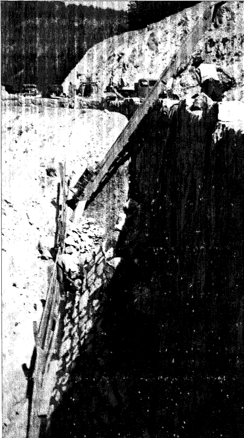
Figure 2.6. Historic photo showing construction of hand-laid rip rap on fill slope of Stevens Canyon, 1940 (MORA Archive).
