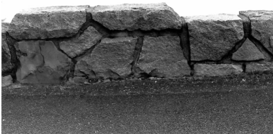
Contemporary photograph showing a detail of the stone masonry guardwall at Ricksecker Point. Note the crenellation in the top of the wall, and the recessed mortar joints, both standard details throughout the 1930s. (CCSO, 1994.)
