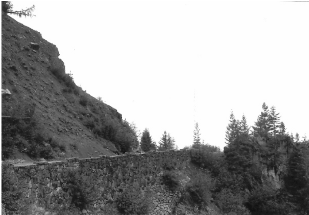
Contemporary photograph of the retaining wall and integrated guardwall along the edge of the road at Ricksecker Point. Note the crenellations in the top of the guardwall. (CCSO, 1994.)
