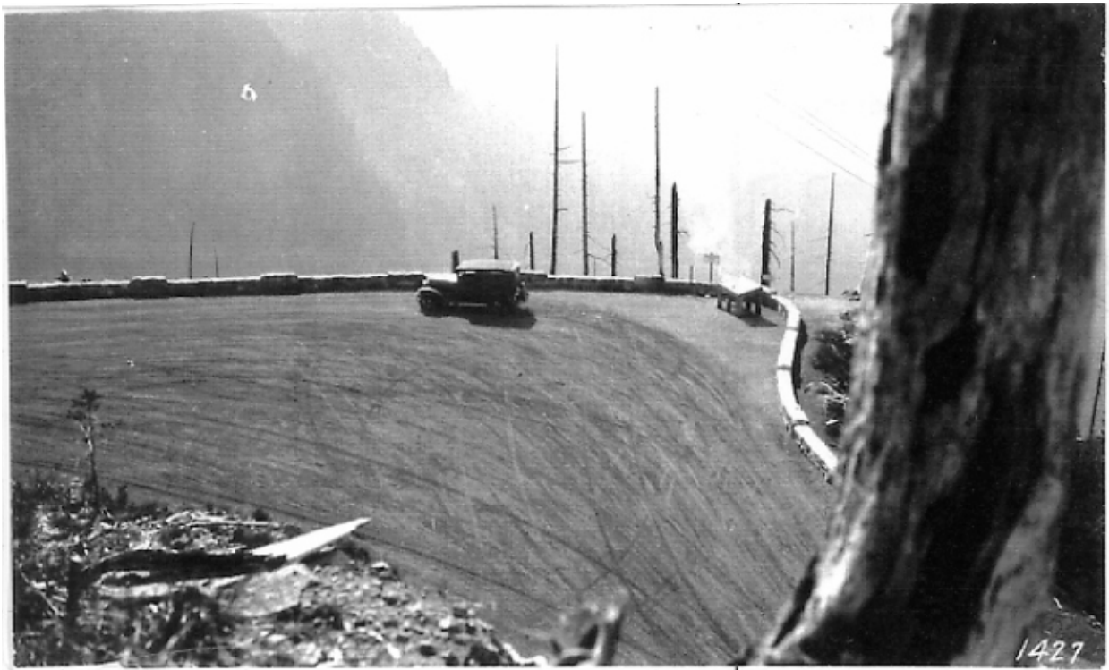
Historic photograph showing the parking area on the southeast side of Ricksecker Point. Note the crenellated stone guardwall, and an interpretive sign. (MORA photo file, neg. 1485, no date.)
