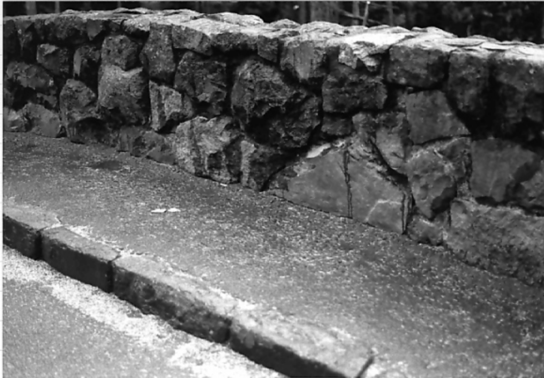
Contemporary photograph of the stone curbing and bituminous sidewalk on the Narada Falls bridge. CCSO, 1994.
