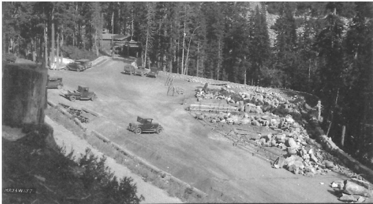
Historic photograph of the Narada Falls parking area, under expansion by the CCC in 1934. Note the stock-piled rubble, for the construction of a guardwall; and the temporary ECW camp across the bridge in the distance. MORA, photo file, neg. 4019.
