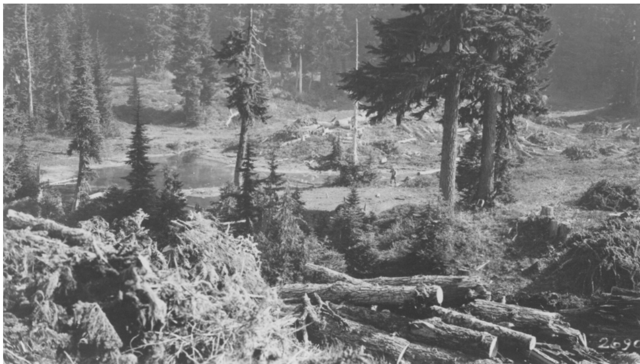
Historic photograph showing the road's terminus at the lake during its clearing and grubbing stage, c. 1928. (MORA Archives, ps 2690)
