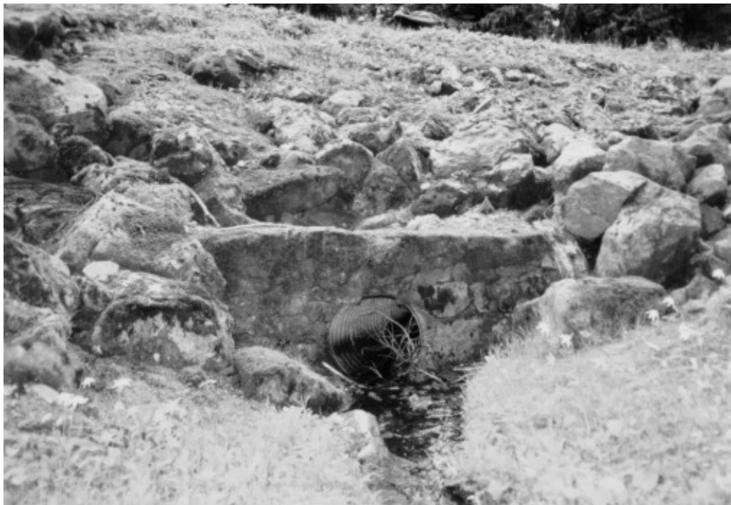
Contemporary photograph showing a typical culvert inlet. Note that the pipe is surrounded by a mortared stone headwall. All original culverts on the Mowich Lake Entrance Road have inlets such as this one. (CCSO 2001)
