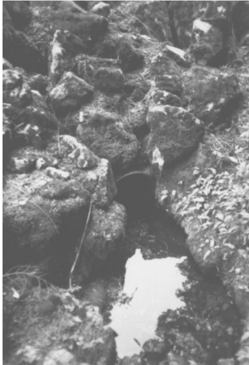
Contemporary photograph showing a typical culvert outfall. Note that the pipe is covered by loosely piled rock. All original culverts on the Mowich Lake Entrance Road have outlets such as this one. (CCSO 2001)
