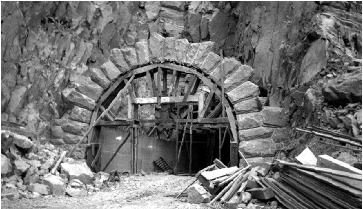
Historic photo showing construction of the north portal of the East Side Highway Tunnel, 1939. (MORA Archives, ps2255)
