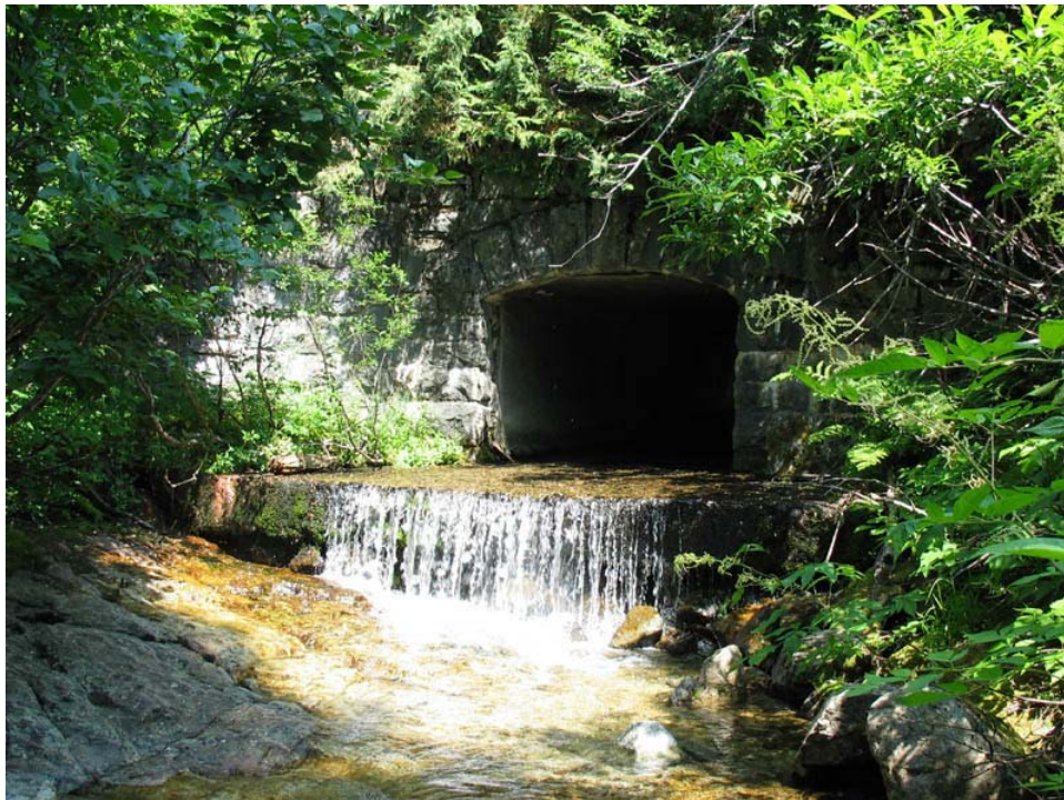
Contemporary photo showing the box culvert and headwall of the Dewey Creek culvert. (MORA, 2004)
