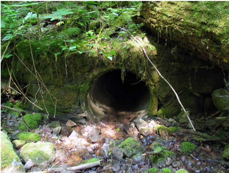
Contemporary photo showing a typical culvert and stone headwall on the East Side Highway. (MORA, 2004)
