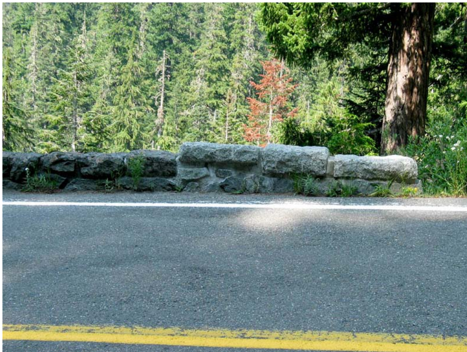
Contemporary photo of a guardwall on the East Side Highway showing modern repairs using incompatible stone. (MORA, 2004)
