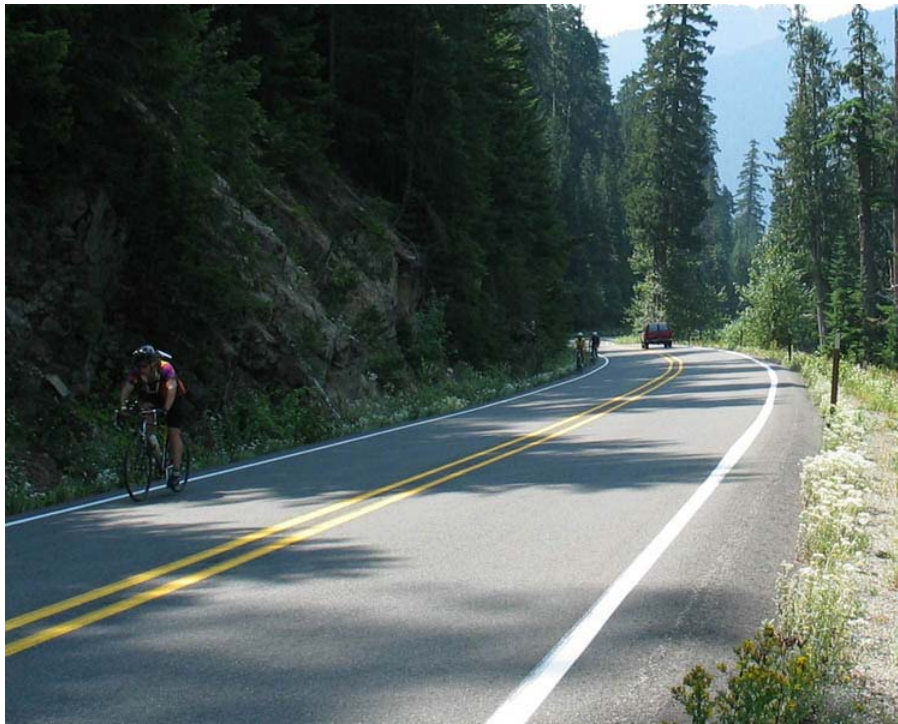
Contemporary photo showing road with paved travel lanes, paved shoulders, and painted lines. The road serves both vehicular and bicycle travel. (MORA, 2004)
