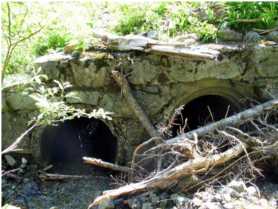
Contemporary photo showing the double culvert at Chinook Creek on the East Side Highway. The culvert is being obstructed by debris. (MORA, 2004)
