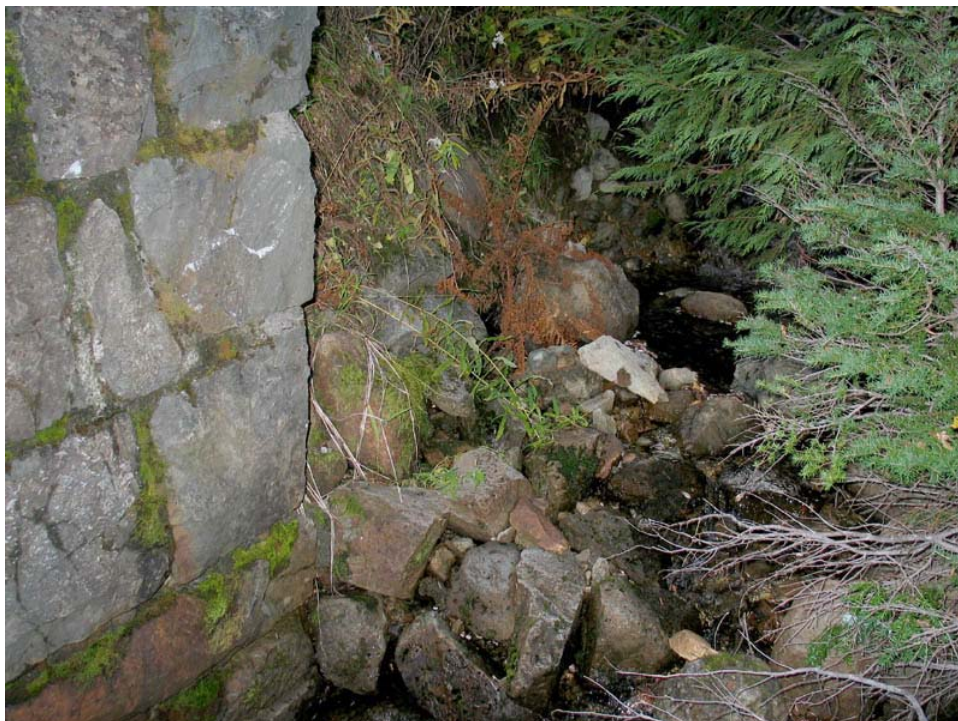
Contemporary photo of a ditch and culvert on the East Side Highway. Constrictions in the ditch create small pools to trap sediment and debris. (MORA, 2004)
