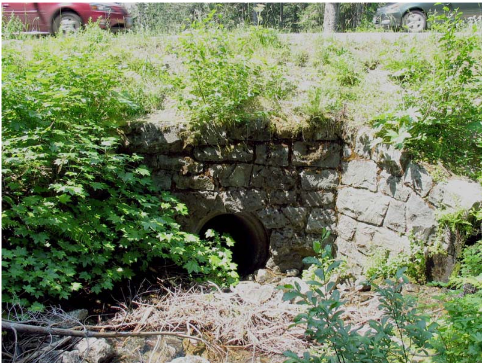
Contemporary photo showing a culvert headwall with angled wing walls. (MORA, 2004)
