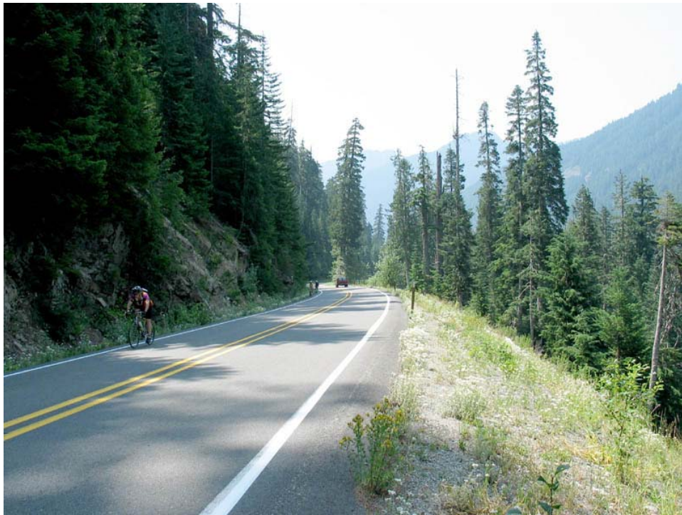
Contemporary photo of the East Side Highway showing a typical half-bench cross section. (MORA, 2004)
