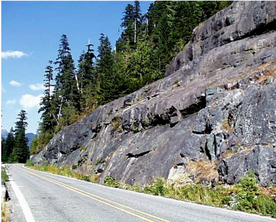
Contemporary photo showing a battered rock cut on the East Side Highway. (MORA, 2004)
