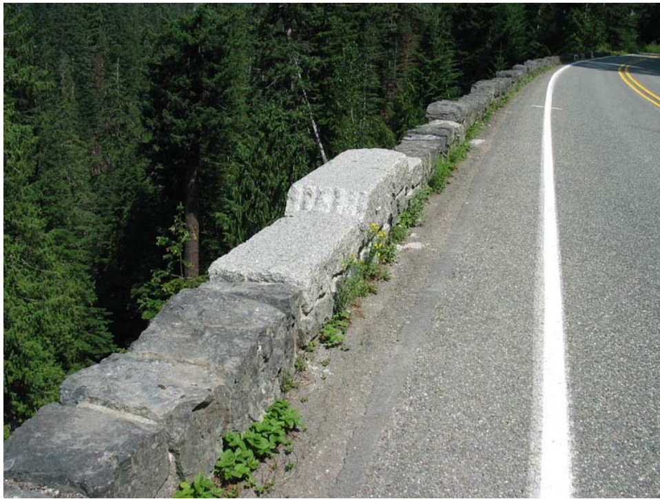
Contemporary photo of a guardwall on the East Side Highway showing recent repairs using incompatible granite. (MORA, 2004)
