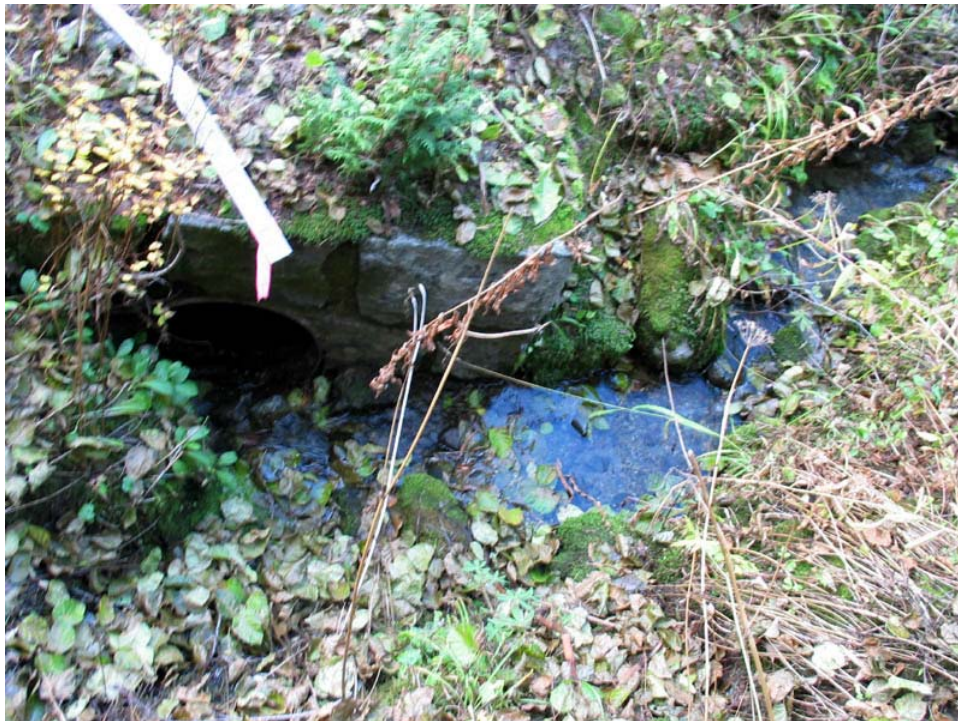
Contemporary photo showing water conveyance in a ditch on the East Side Highway. The water is diverted just before the culvert to trap sediment and debris. (MORA, 2004)
