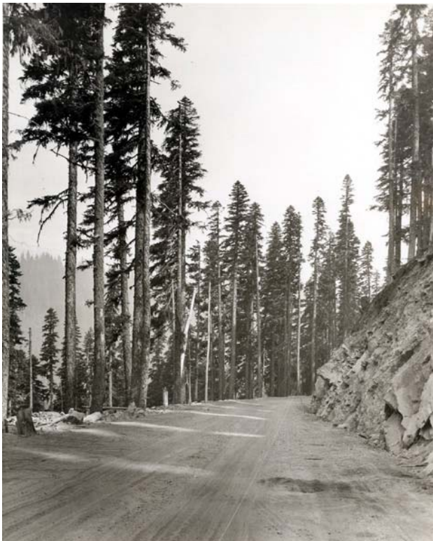
Historic photo showing rock cut and retention of trees adjacent to the road, 1937. (MORA Archives, twc2763)
