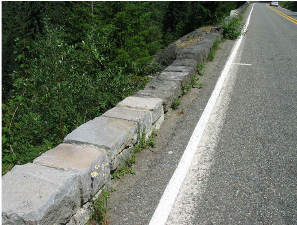
Contemporary photo of a guardwall on the East Side Highway showing a recent repair with compatible stone material. (MORA, 2004)
