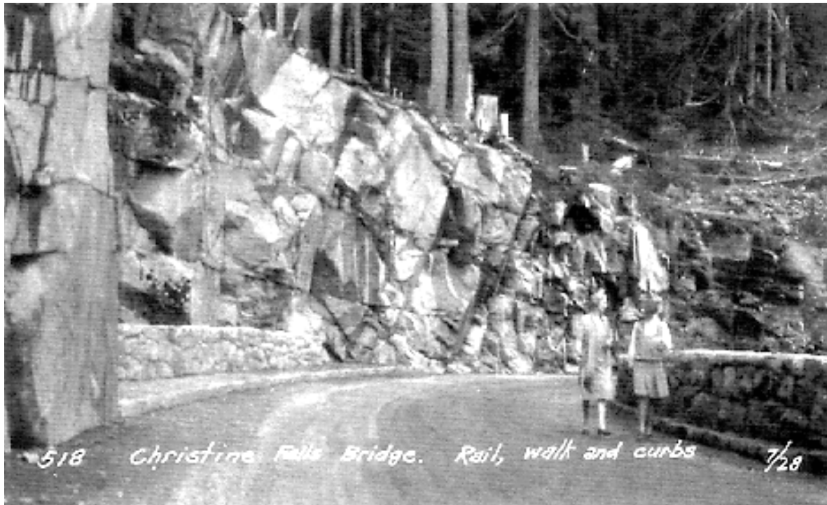
1928 photograph illustrating the guardwalls, curbs and sidewalk along the north side of the Road to Paradise at Christine Falls bridge. MORA photo file, neg. 1312.
