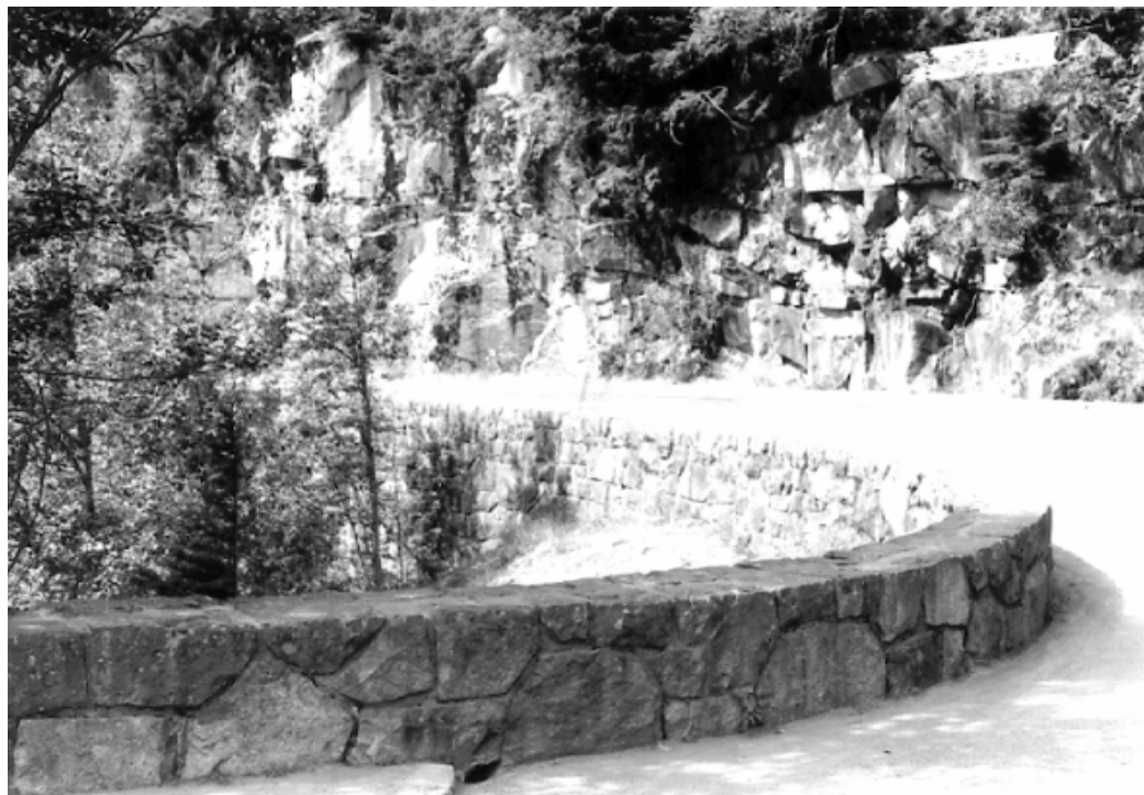
Masonry walls at the pullout on the east side of Christine Falls bridge. This wall was built as an extension to the original guardwall in 1941. CCSO, 1994.
