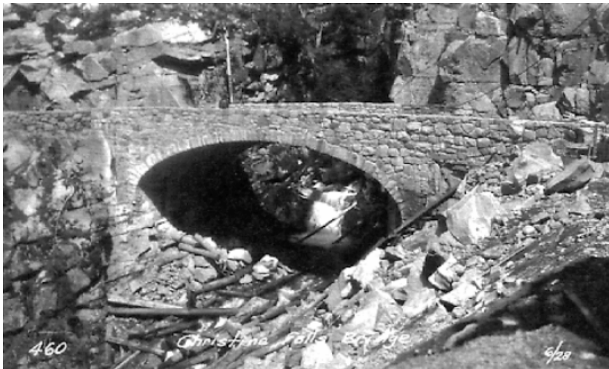
1928 photograph illustrating debris beneath Christine Falls bridge, as a result of construction work. The debris was removed after construction, and the creek bed was lowered, resulting in a more picturesque drop for the falls. MORA photo, neg. 1311.
