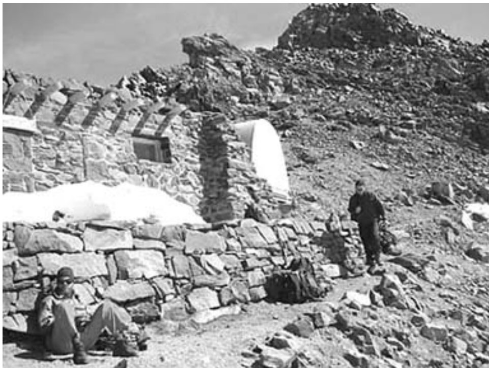
Contemporary photograph of the Public Shelter. Note the blocked in historic door at the far left of the photograph, taken 2001. Note the exposed whole log rafter tails, a character defining feature of the Public Shelter. NPS Photo
