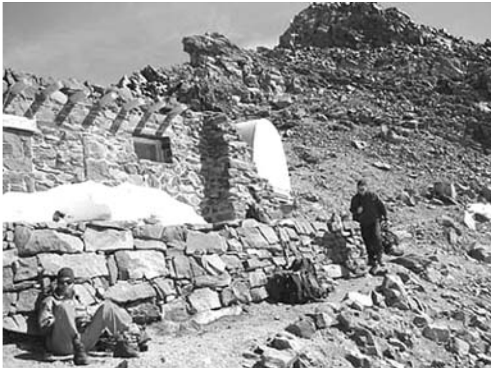
Contemporary photograph of the Public Shelter, 2001. Note the historic sign at the far left side of photo above the blocked in historic doorway. A wood and stone bench is located under the snow drift, above the rock retaining wall. NPS Photo
