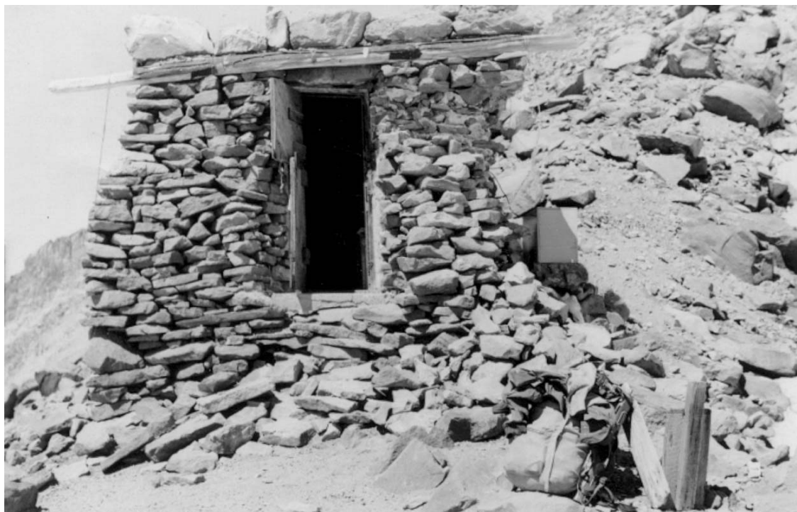
Historic photograph of the Guide Shelter, 1962. Note the dry-laid masonry walls. MORA Archive (muir1)
