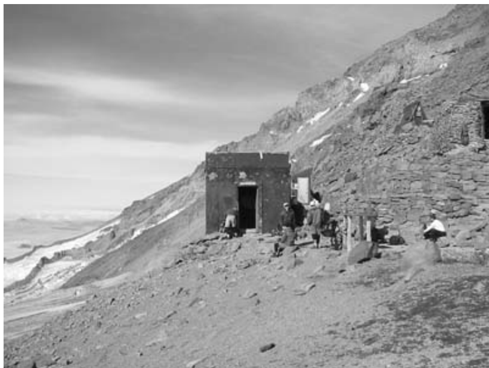
Contemporary photograph of the Gombu Shelter, Guide Shelter, Butler Shelter, and Pit Toilet, 2001. Also note the retaining walls built on the downhill sides of the Gombu Shelter, Guide Shelter, and Butler Shelter. NPS Photo
