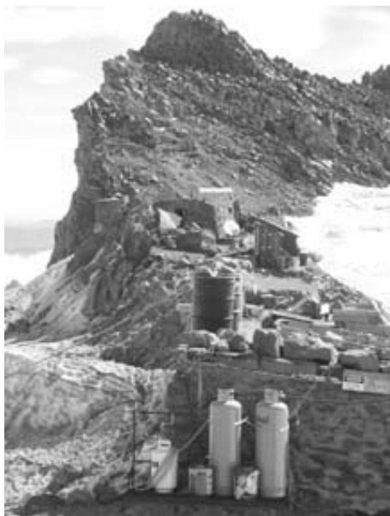
Contemporary photograph of the narrow ridge on which Camp Muir is sited. NPS Photo
