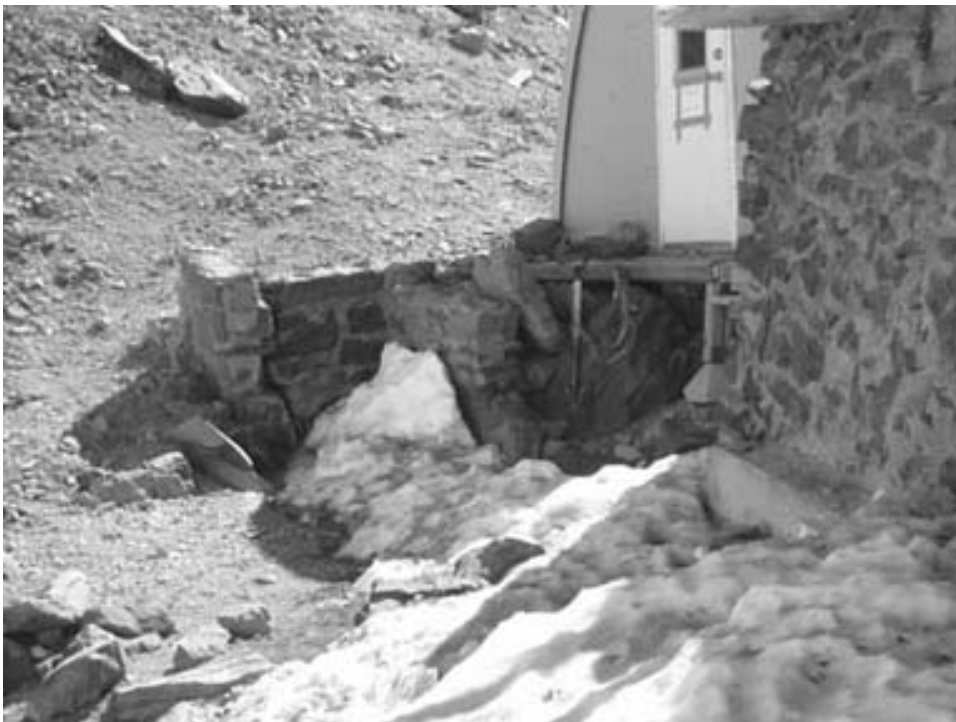
Contemporary photograph of the ruins of the women's pit toilet, 2001. Also note the rear wall of the Public Shelter showing mortar applied to the stone after the period of significance, and the Weatherport behind. NPS Photo
