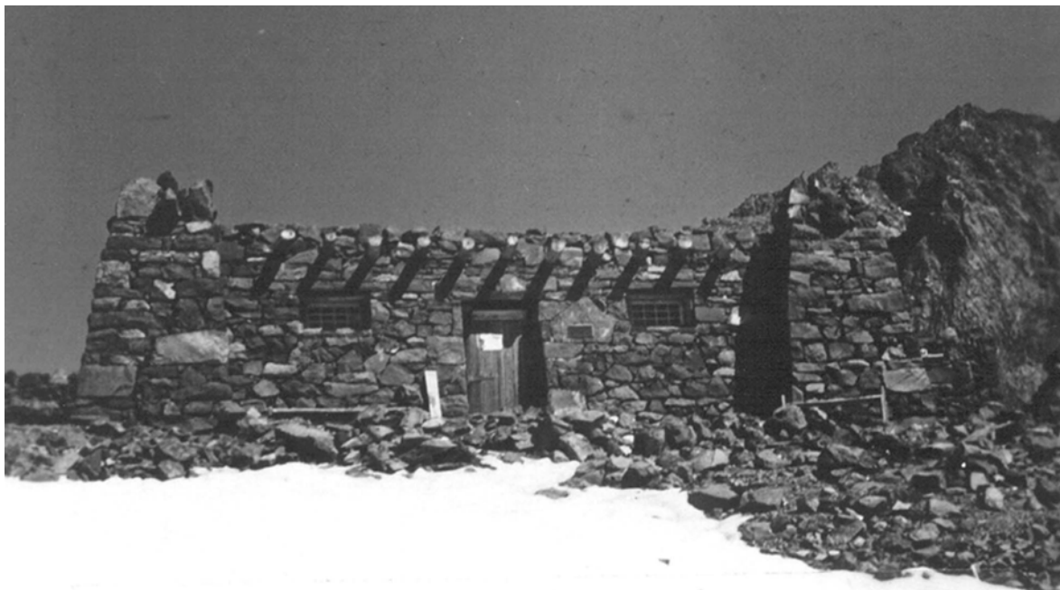
Contemporary photograph of the Public Shelter. Note the blocked in historic door at the far left of the photograph, taken 2001. Note the exposed whole log rafter tails, a character defining feature of the Public Shelter. NPS Photo
