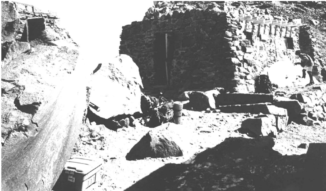
Contemporary photograph of the Public Shelter, 2001. Note the rock outcropping and the loss of finials from the tops of the wing walls. NPS Photo
