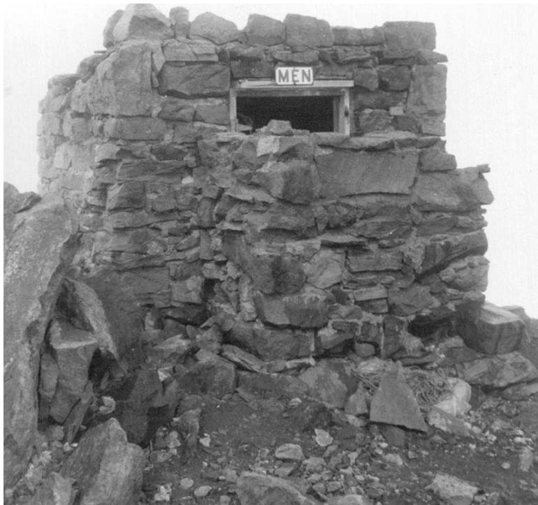
Historic photograph of the men's pit toilet, 1962. Converted for use as a storage shed in 1973. Note the stone masonry parapet wall in front of the door, which was removed in 1973. MORA Archive (muir8)
