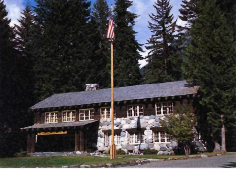
Longmire Administration Building
