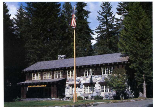
Longmire Administration Building NPS
