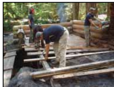
The historic Ipsut Creek Patrol Cabin, undermined by flood waters, was deconstructed in August and transported to Tahoma Woods for restoration.
