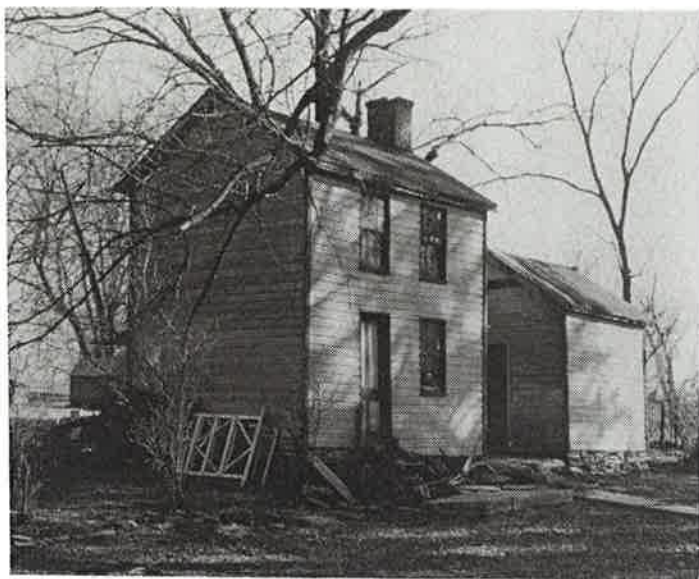
Photograph 4. Circa 1872 Servants' quarters and smoke-house. Photograph courtesy of the Vivino family, 1962.
