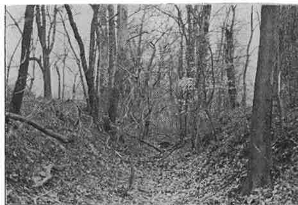
Photograph 11. The millrace, (JMA, 1993).
